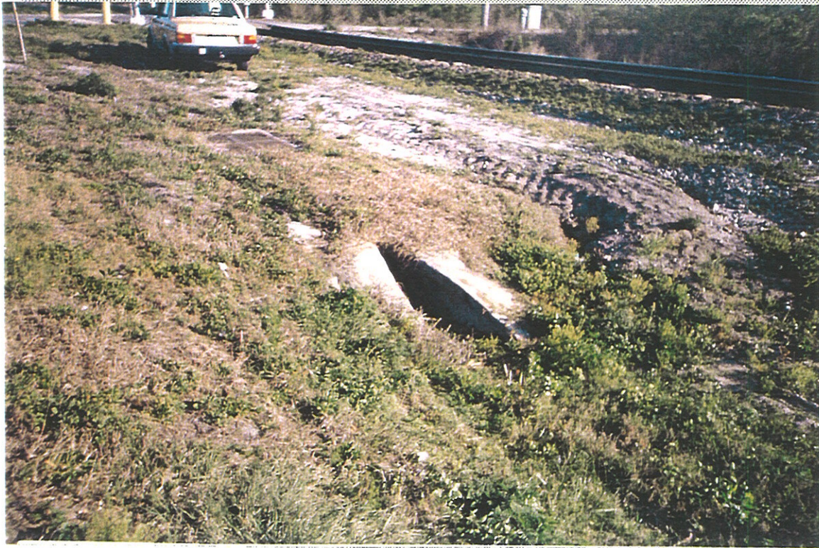
VIEW OF D-3 LOOKING NORTH
