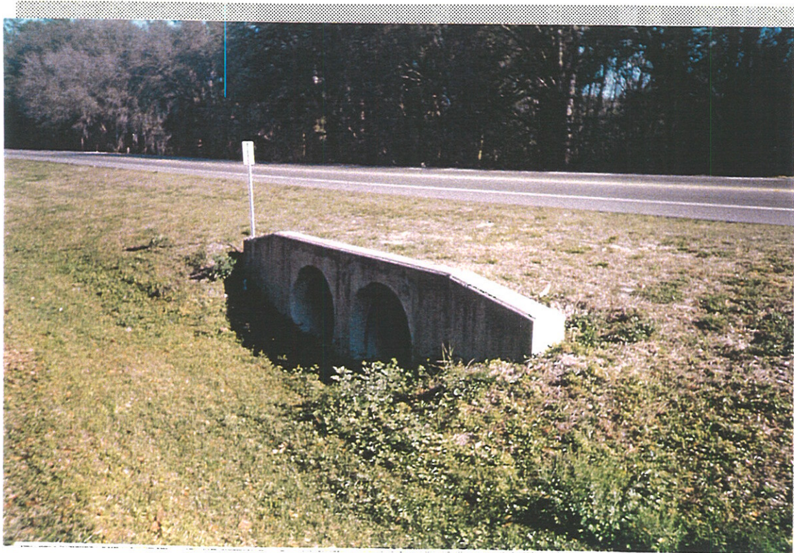
VIEW OF D-17 LOOKING EAST
