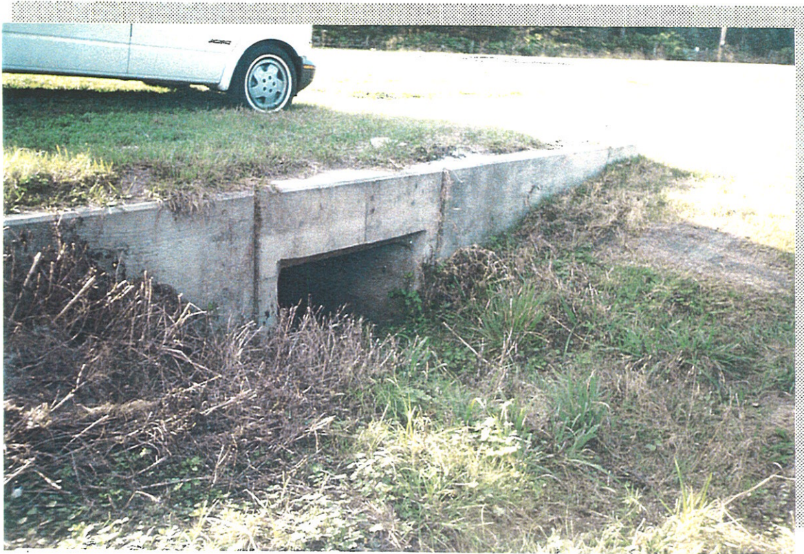
VIEW OF D-9 LOOKING WEST
