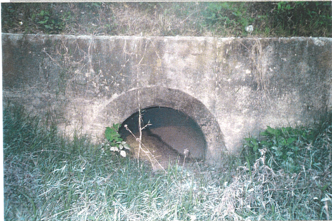
VIEW OF D-23 LOOKING EAST
