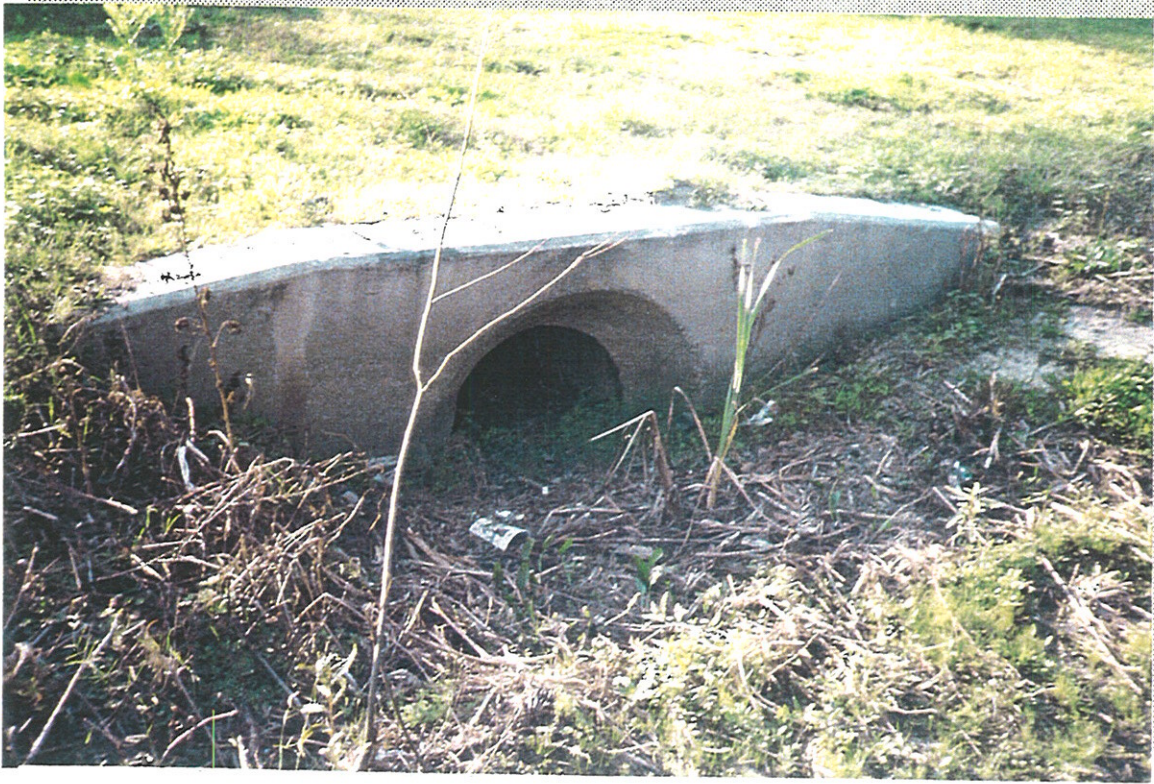
VIEW OF D-16 LOOKING WEST
