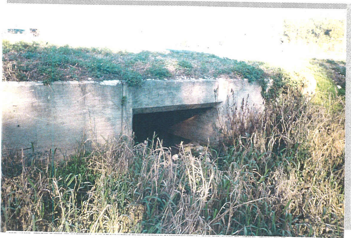
VIEW OF D-1 LOOKING WEST
