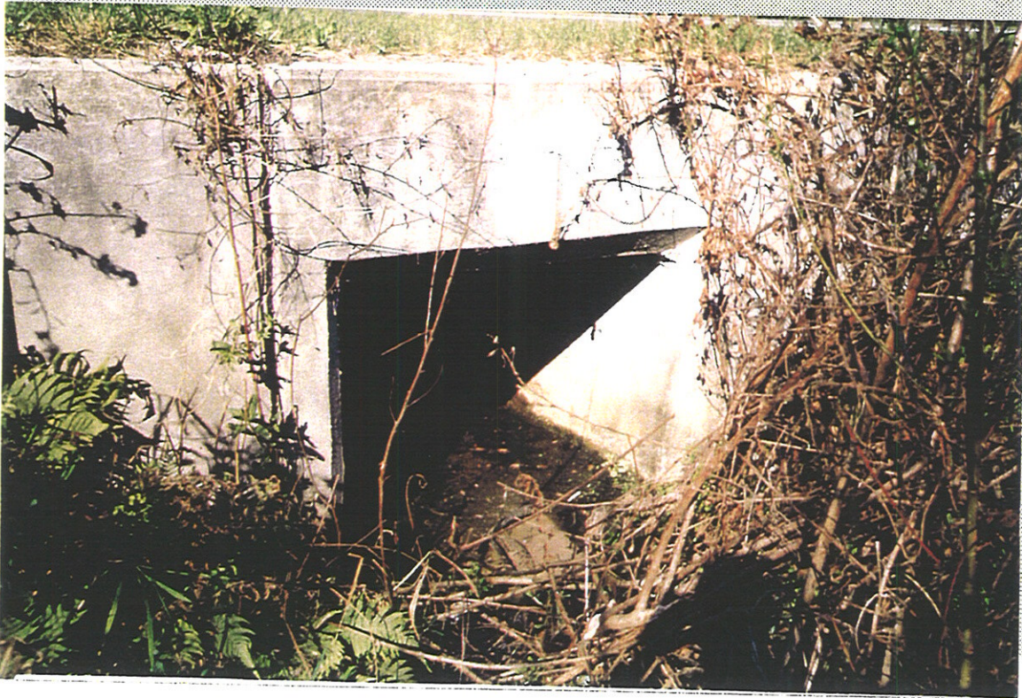
VIEW OF D-14 LOOKING WEST
