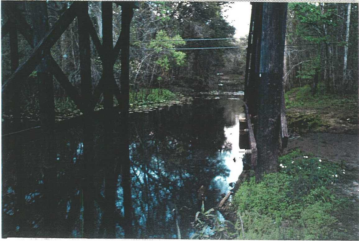
VIEW OF THE HILLSBOROUGH RIVER (B-3)
