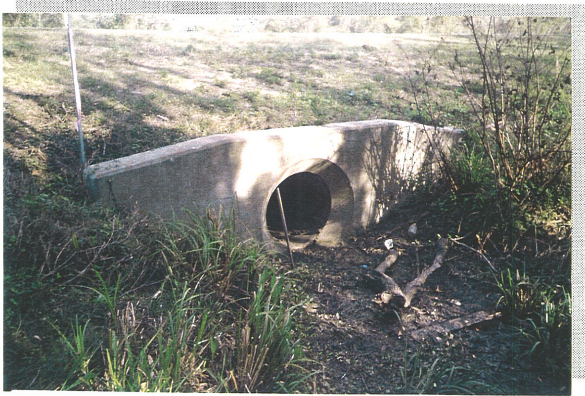
VIEW OF D-8 LOOKING EAST
