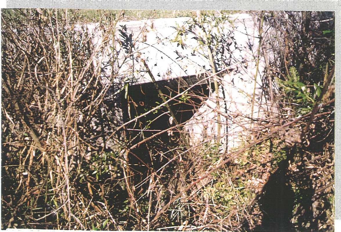
VIEW OF D-13 LOOKING WEST
