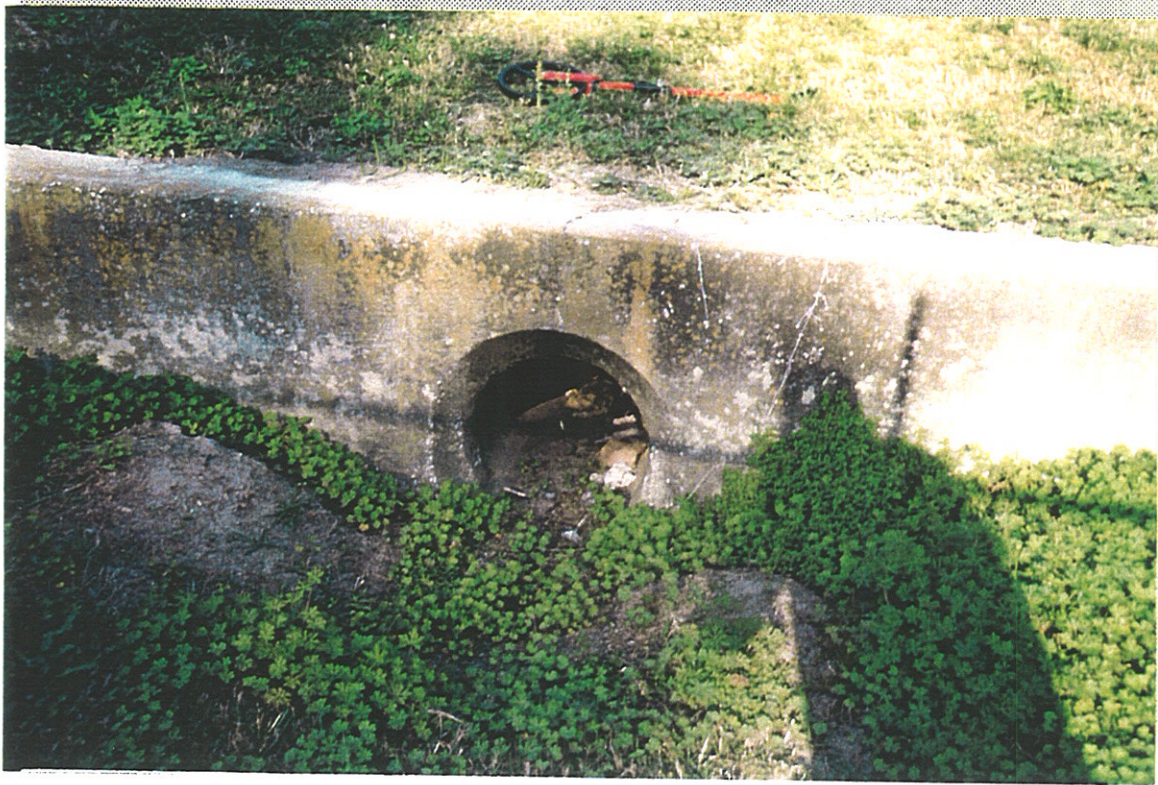
VIEW OF D-18 LOOKING EAST
