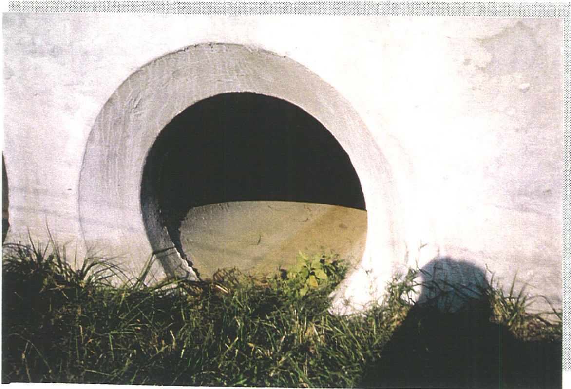
VIEW OF D-21 LOOKING EAST
