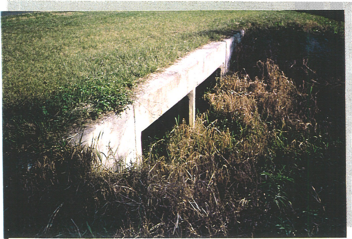
VIEW OF D-5 LOOKING EAST
