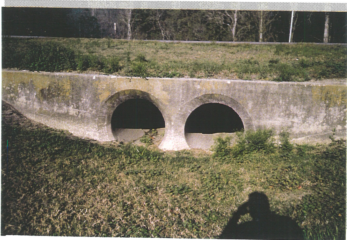
VIEW OF D-19 LOOKING EAST
