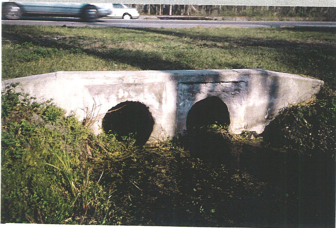
VIEW OF D-15 LOOKING EAST
