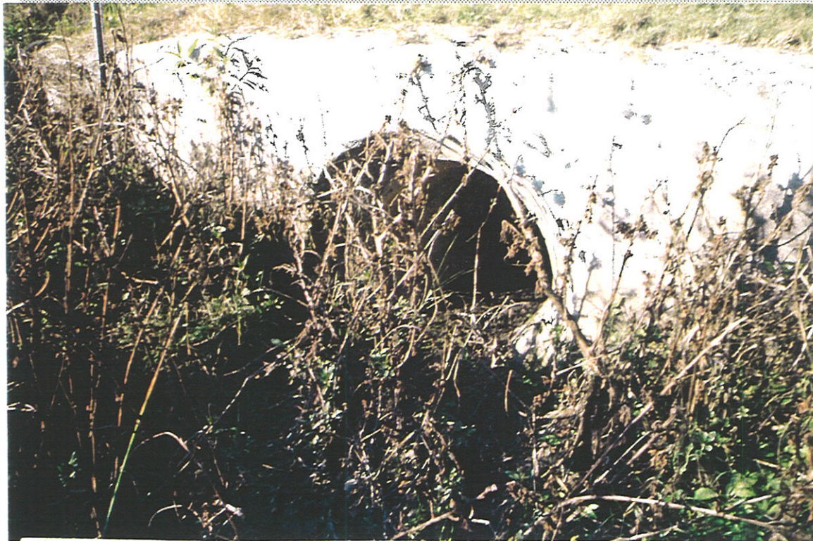
VIEW OF D-4 LOOKING WEST
