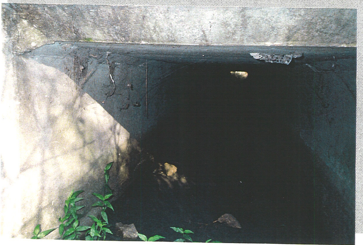
VIEW OF D-10 LOOKING EAST
