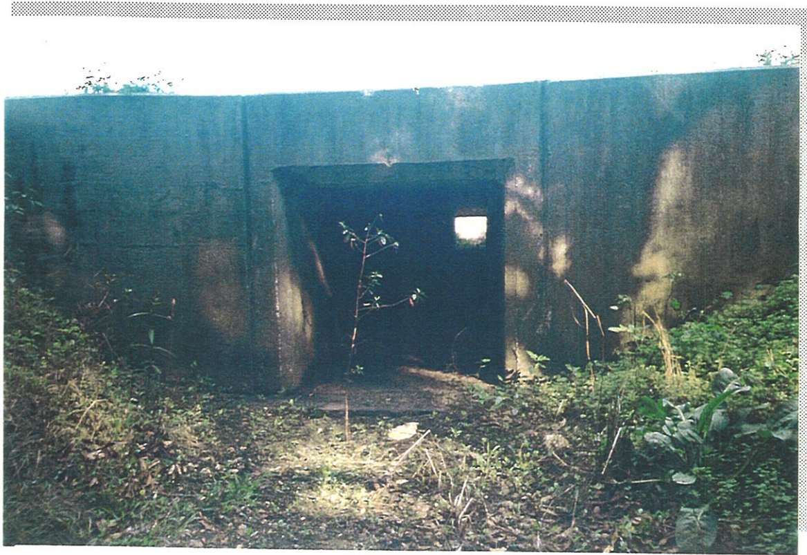
VIEW OF D-7 LOOKING EAST
