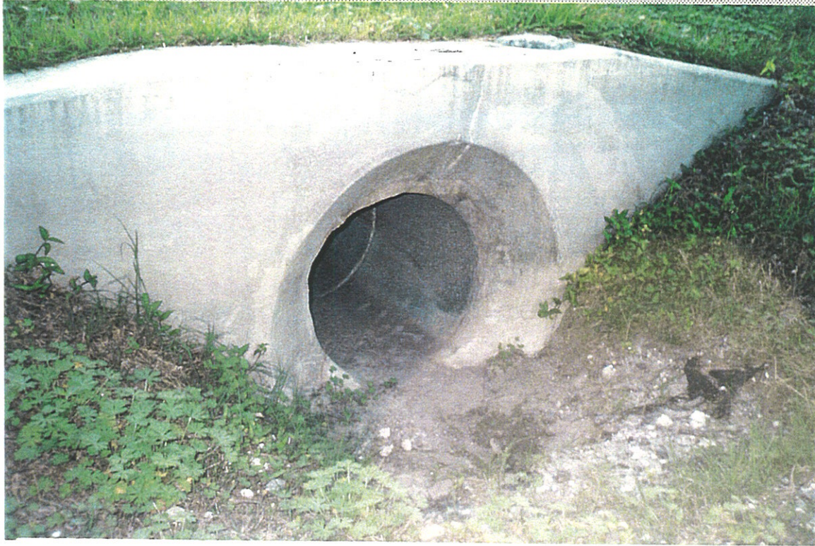
VIEW OF D-22 LOOKING WEST
