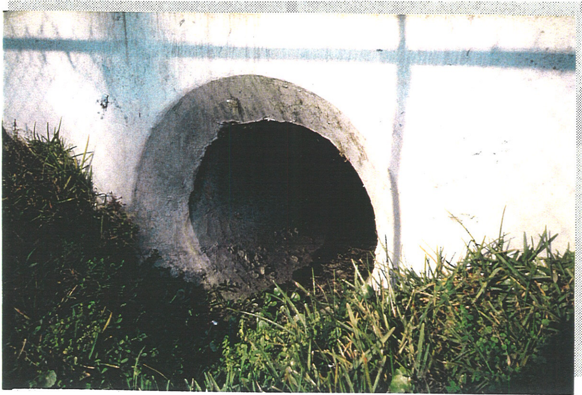
VIEW OF D-20 LOOKING EAST
