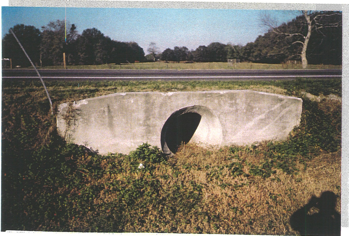
VIEW OF D-2 LOOKING WEST
