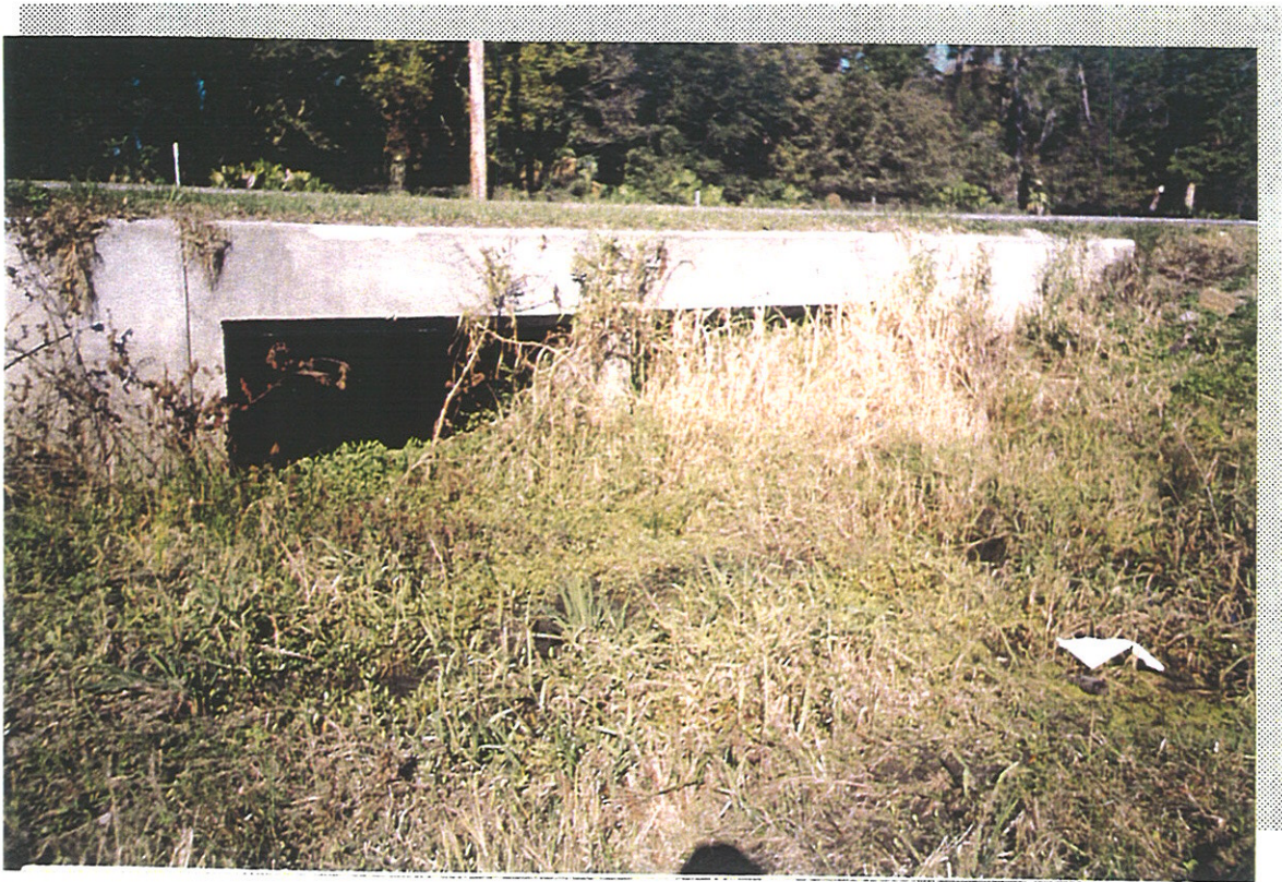
VIEW OF D-11 LOOKING WEST
