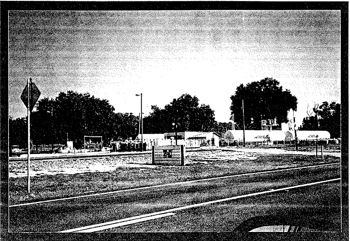
Photograph 4. AmeriGas. View is to the southeast. Note the railroad tracks.
