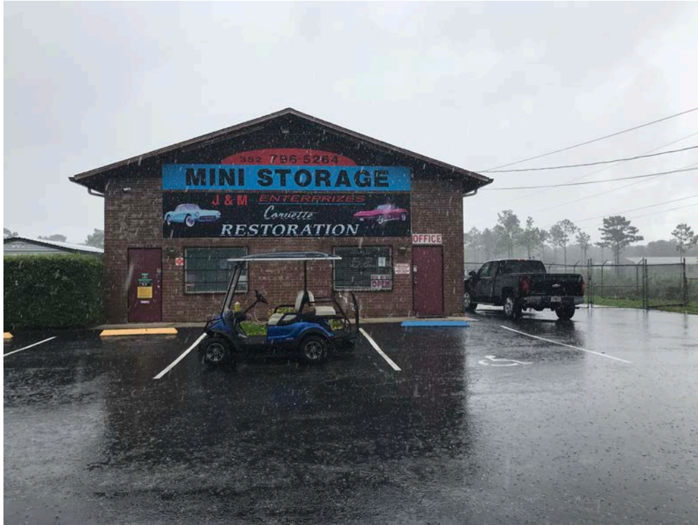
Site 20: J&M Enterprizes Inc. taken from SR 50 looking north; Photo taken June 14, 2019.
