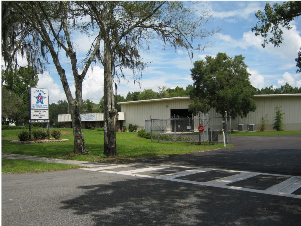
Site 4: Five Star Refrigeration and Air Conditioning (F.K.A. Coca-Cola Bottling Co.) taken from SR 50 looking north; Photo taken August 12, 2015.
