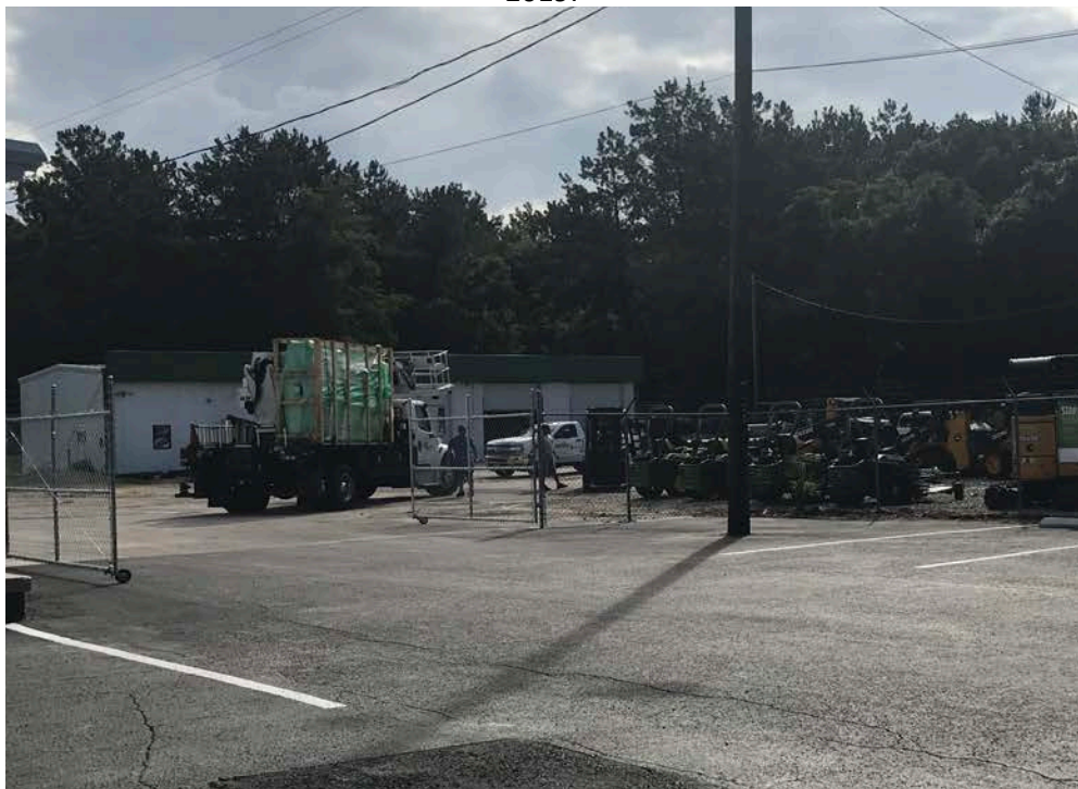
Site 3: Precision Powerstroke (now vacant) taken from SR 50 looking northeast; Photo taken June 18, 2019.
