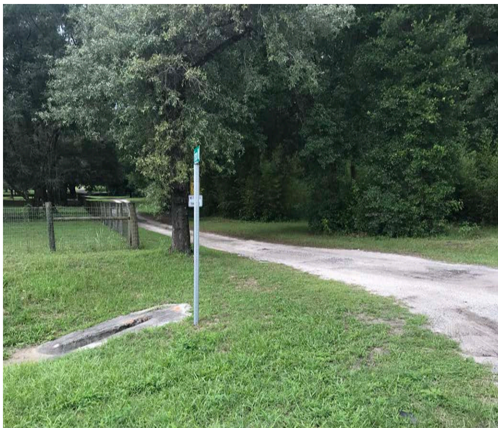
Site 15: Corner of Frisco Road taken from SR50 looking south; Photo taken June 14, 2019
