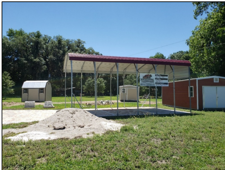
Photo 2. South view of FPC 3-4A.
