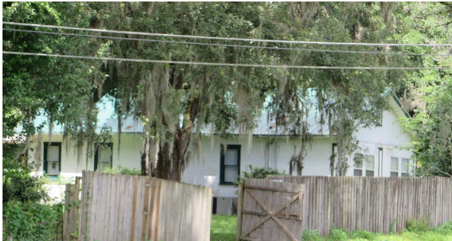
Photo 5-19 24286 Cortez Boulevard (8HE719), looking northwest
