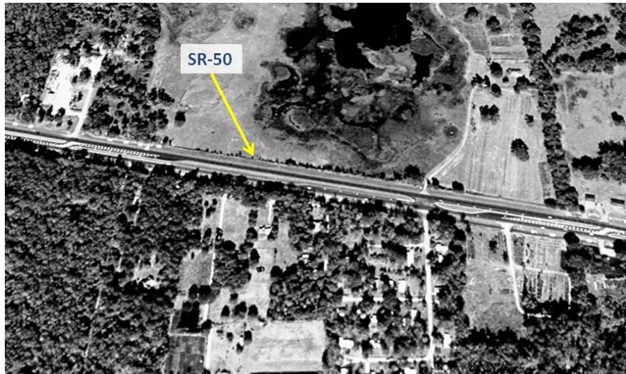
Figure 5-10 1999 satellite image depicting an enlarged SR 50 featuring four lanes and a median (Google Earth 1999)
