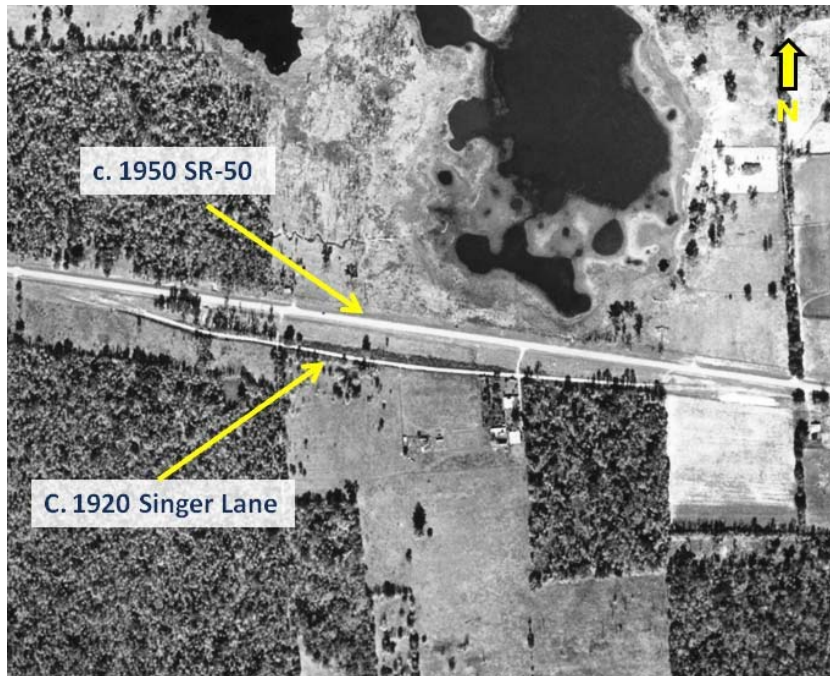
Figure 5-8 1952 PALMM aerial depicting the construction of SR 50 around 1950 and the remaining section of the 1920s roadway, renamed Singer Lane
