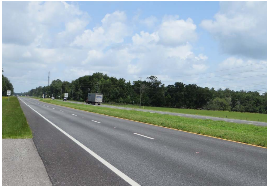
Photo 5-24 SR 50 (8HE742), looking west
