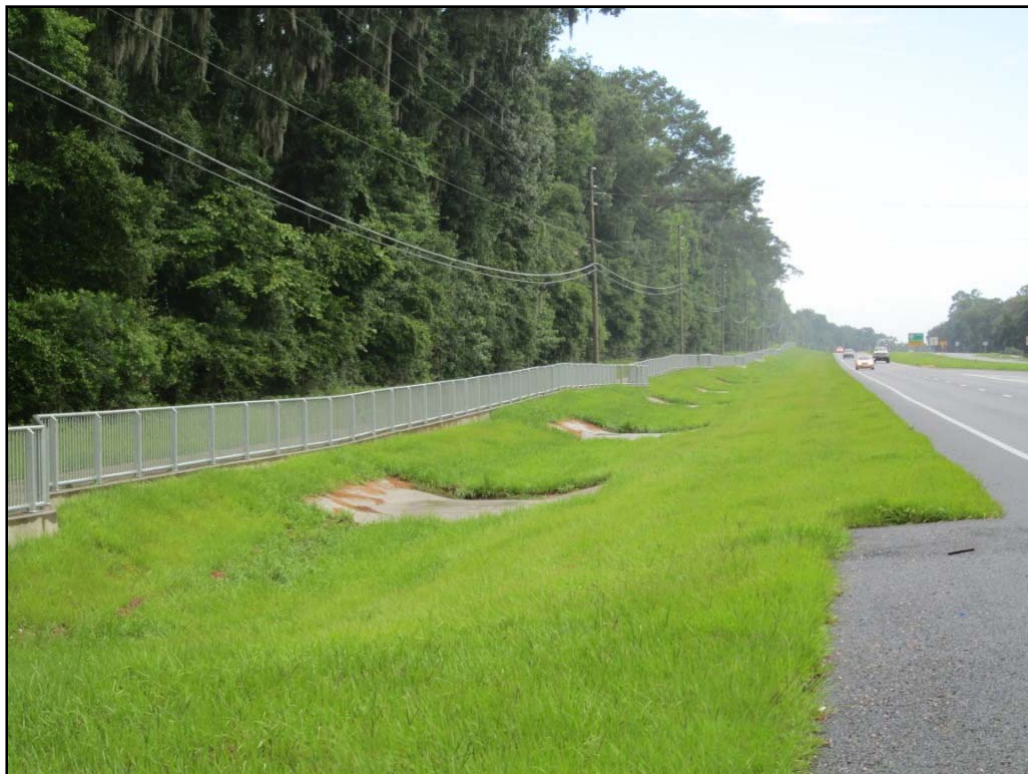
Photo 2-1 General view of SR 50, looking to the west.
