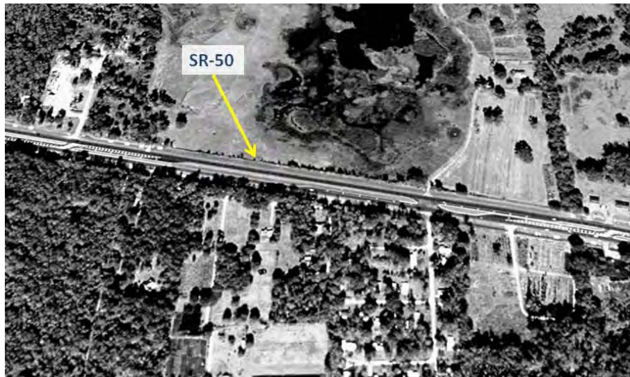
Photo 2. 1999 satellite image depicting an enlarged SR 50 featuring four lanes and a median (Google Earth 1999).
