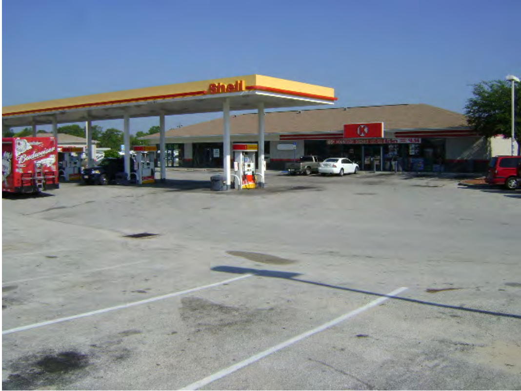
Photo #17: View of Site 17 from the south.
