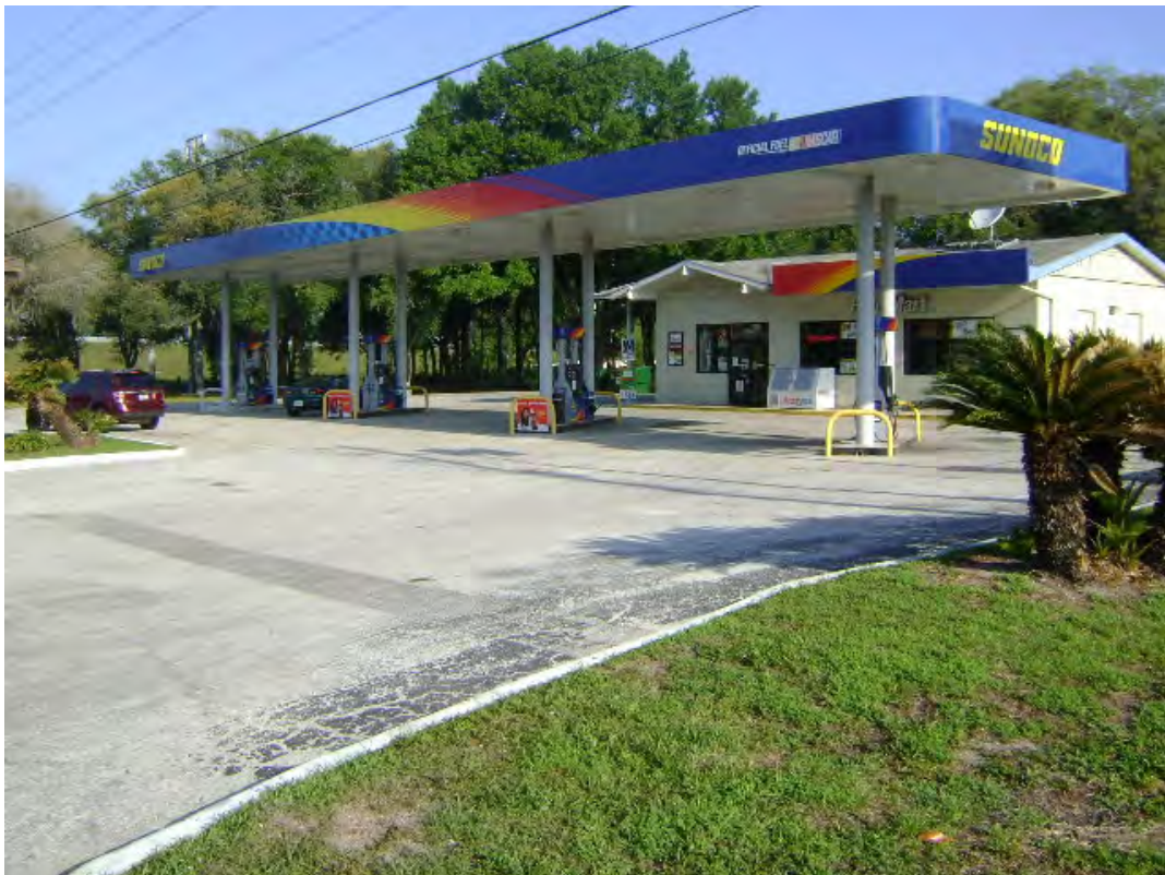
Photo #4: View of Site 4 from the southeast.
