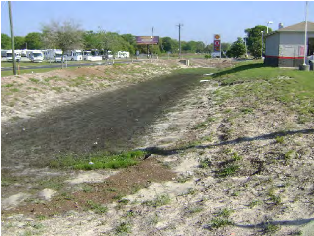
Photo #18: View of the stormwater pond/swale at Site 17.
