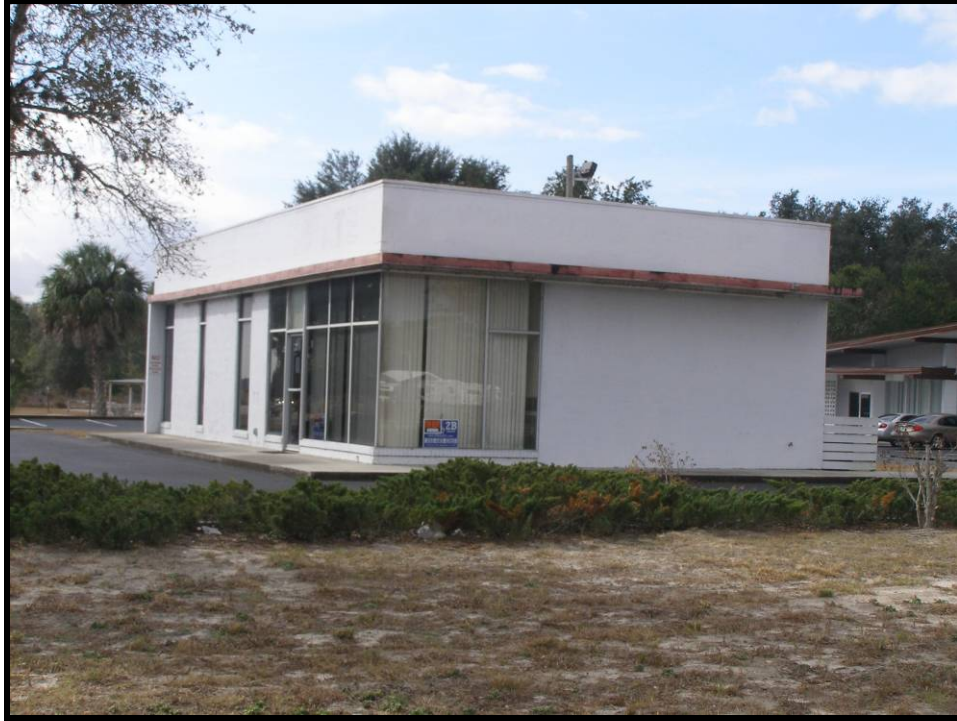
Photo 16. North and east elevations of 34508 Cortez Boulevard, 8HE692.
