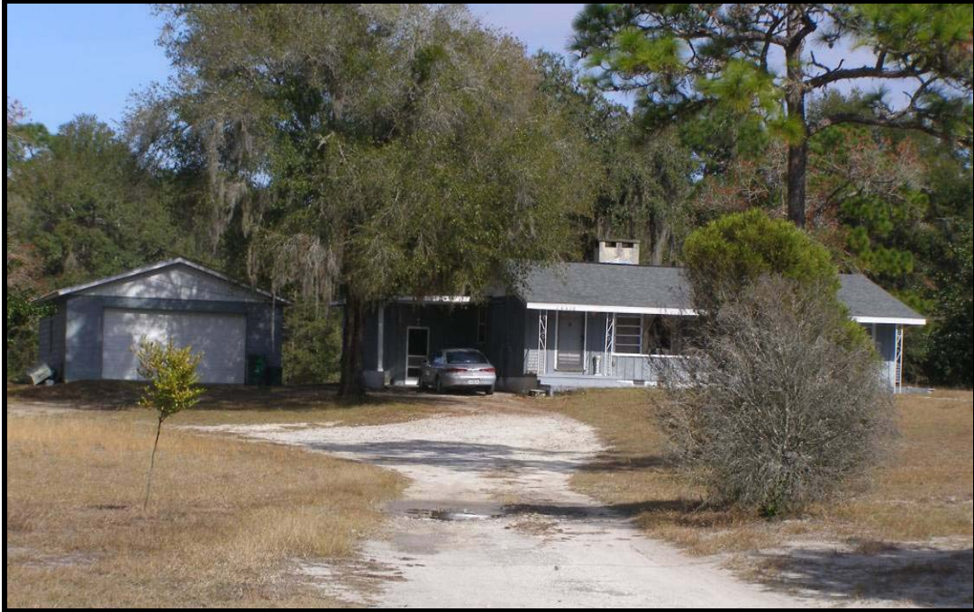
Photo 10. South elevation of 34415 Cortez Boulevard, 8HE687.
