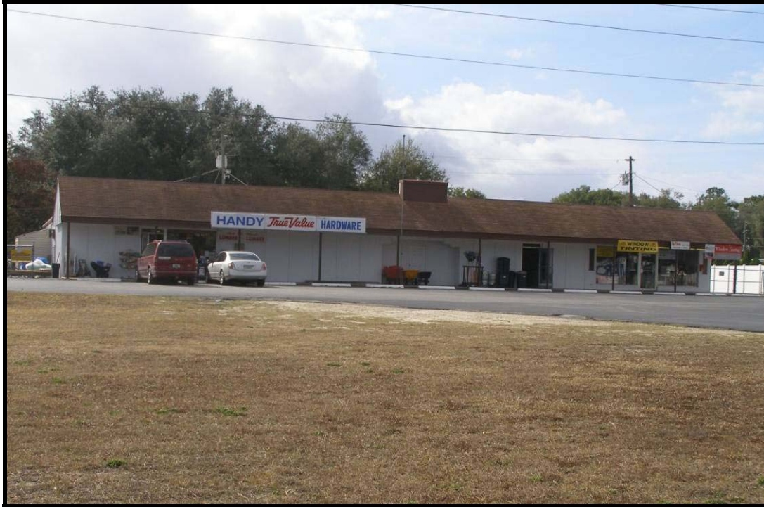
Photo 15. North elevation of 34486 Cortez Boulevard, 8HE691.
