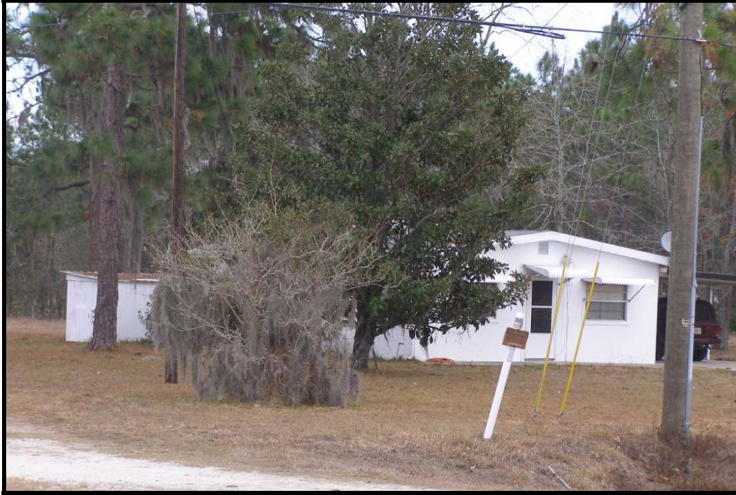
Photo 3. South and west elevations of 29373 Cortez Boulevard, 8HE680.
