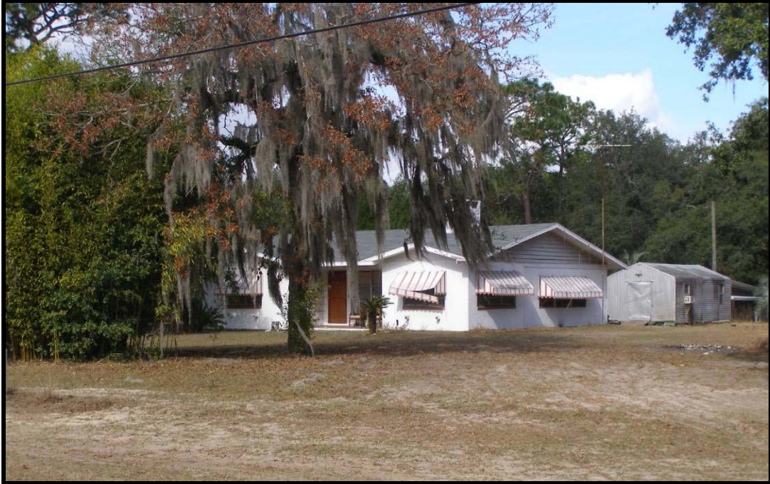
Photo 8. South and east elevations of 33555 Westwood Drive, 8HE685.
