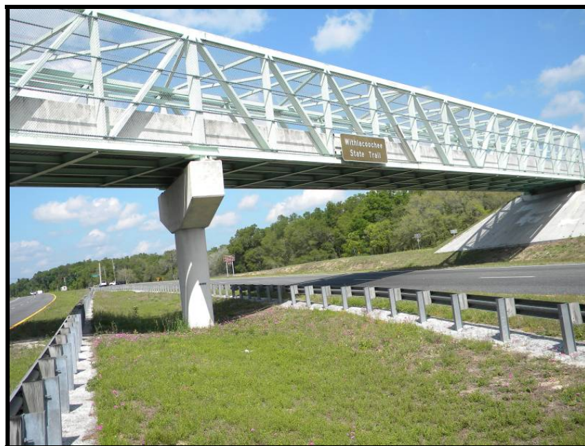
Photo 1. Looking west from SR 50 (Cortez Boulevard) at CSX Railroad segment.
