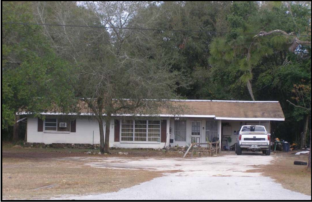
Photo 5. South elevation of 33325 Cortez Boulevard, 8HE682.
