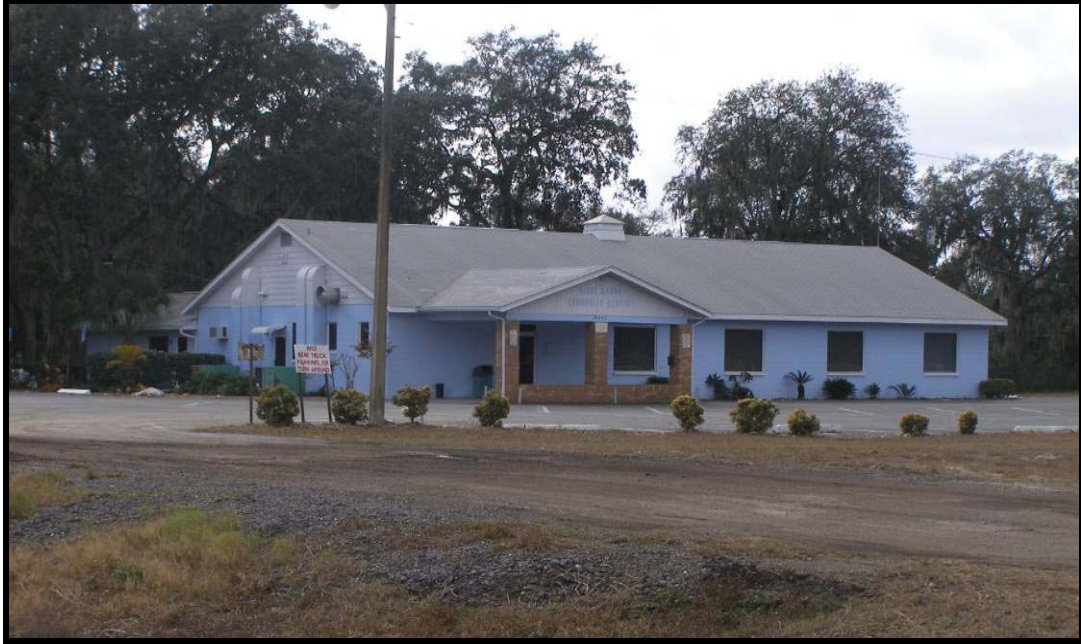
Photo 9. North and east elevations of 34240 Cortez Boulevard, 8HE686.
