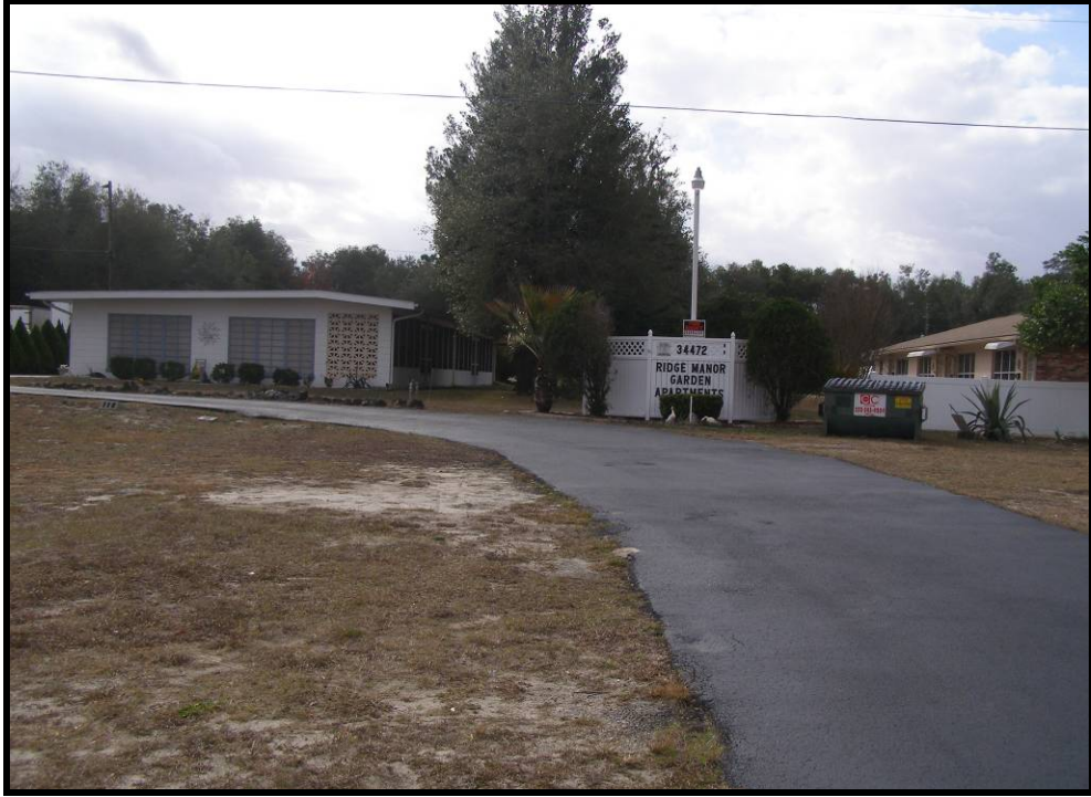
Photo 12. General view of the Ridge Manor Garden Apartments, 8HE678.
