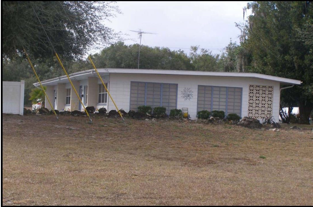
Photo 14. South and east elevations of 34472 Cortez Boulevard, Building 2, 8HE690.
