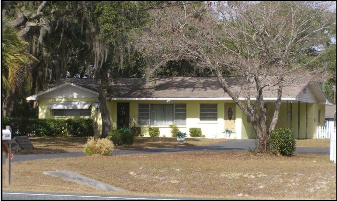
Photo 4. South and east elevations of 33297 Cortez Boulevard, 8HE681.
