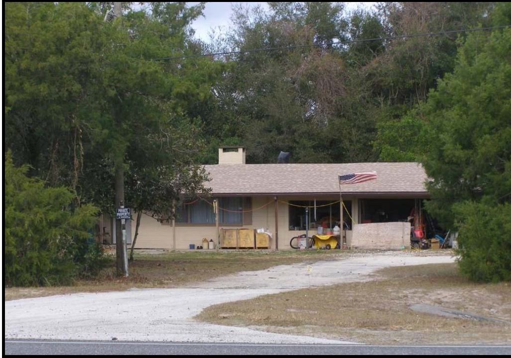
Photo 6. South elevation of 33345 Cortez Boulevard, 8HE683.
