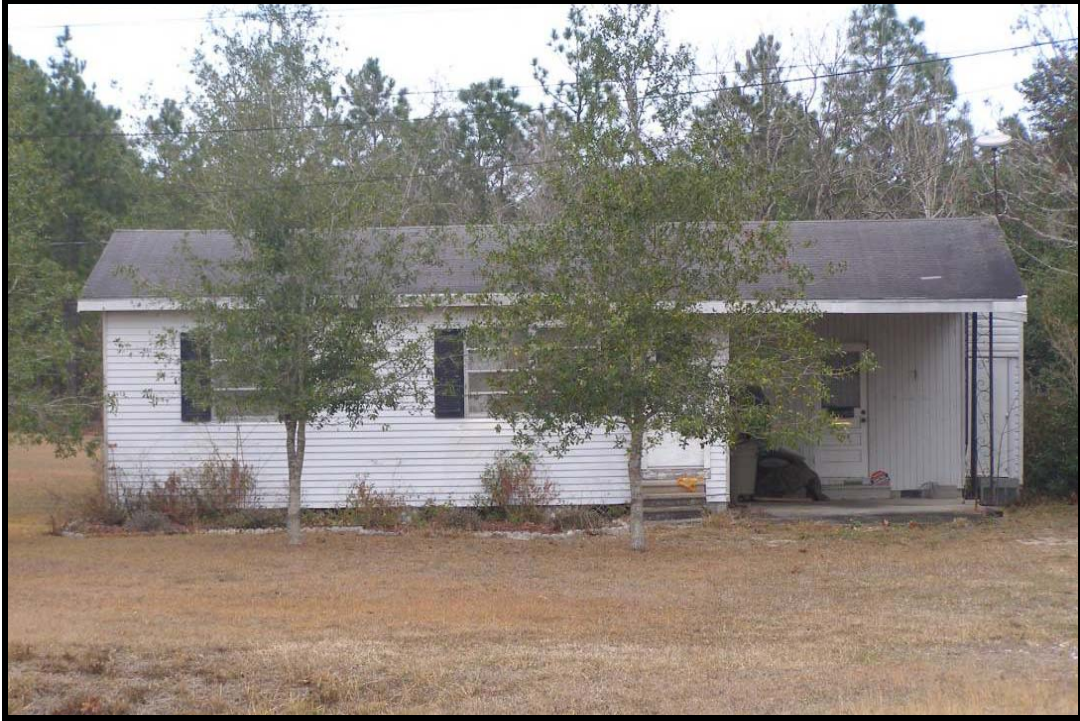
Photo 2. South elevation of 29367 Cortez Boulevard, 8HE679.
