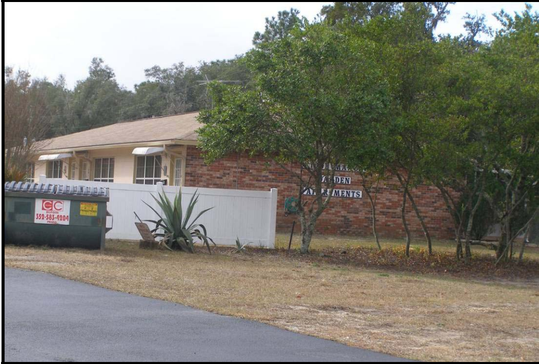
Photo 13. North and east elevations of 34472 Cortez Boulevard, Building 1, 8HE689.
