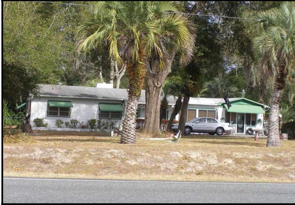
Photo 7. South elevation of 33359 Cortez Boulevard, 8HE684.
