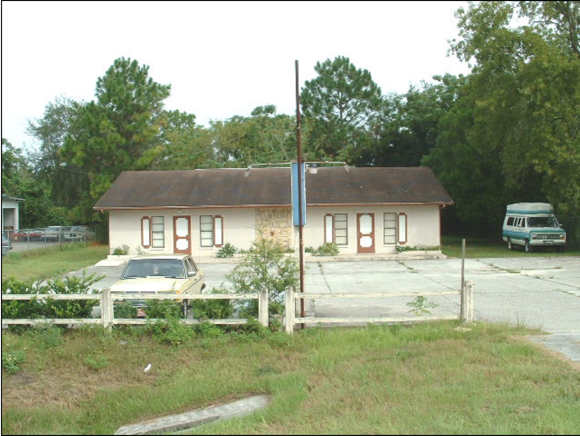
Location: 15531 Cortez Boulevard Reason for Possible Relocate: Right turn lane at B.W. Stevenson Road Building Faces: South
