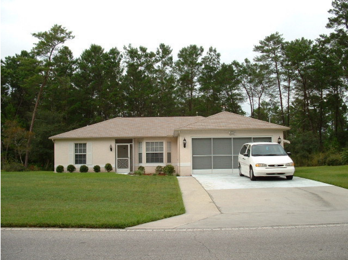
Location: 6377 Freeport Drive (Residential) Reason for Possible Relocate: Proposed Pond Location - Basin B Building Faces: Southwest
