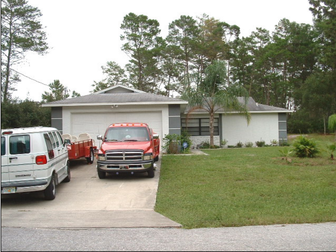
Location: 6310 Melshire Avenue (Residential) Reason for Possible Relocate: Proposed Pond Location - Basin B Building Faces: West
