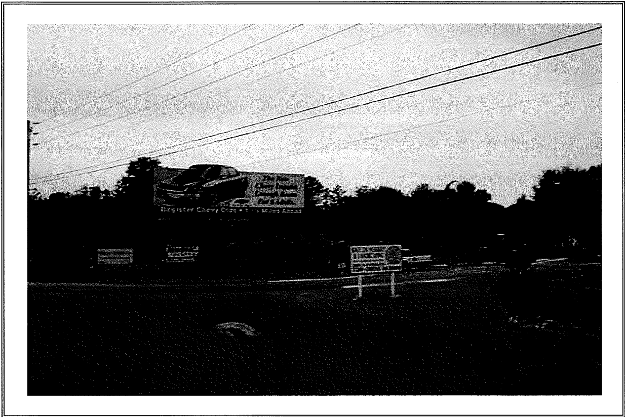
Photo 9. View from the south showing the Save-on Nursery Facility (60-P/HM/HW-H).
