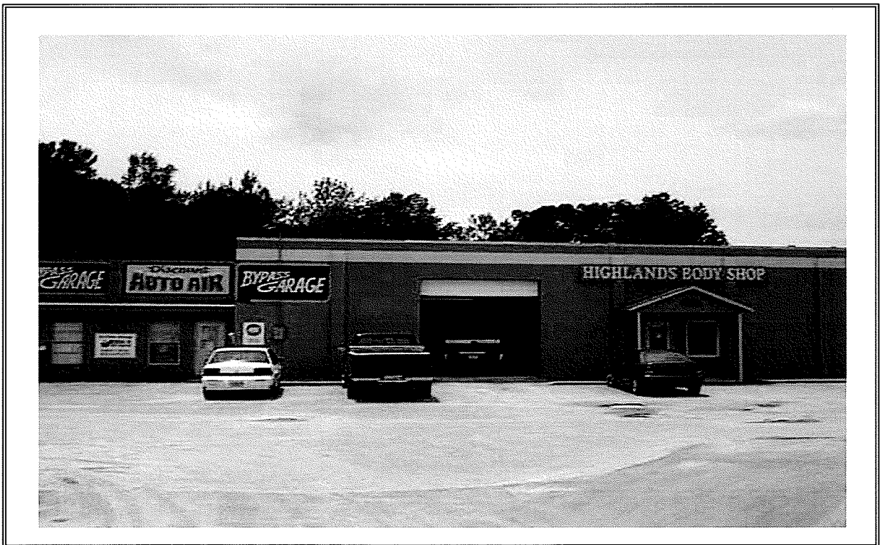
Photo 14. View from the east showing both the Highlands Body Shop and ByPass Garage Facilities (81-P/HM/HW-M and 82-P/HM/HW-M).
