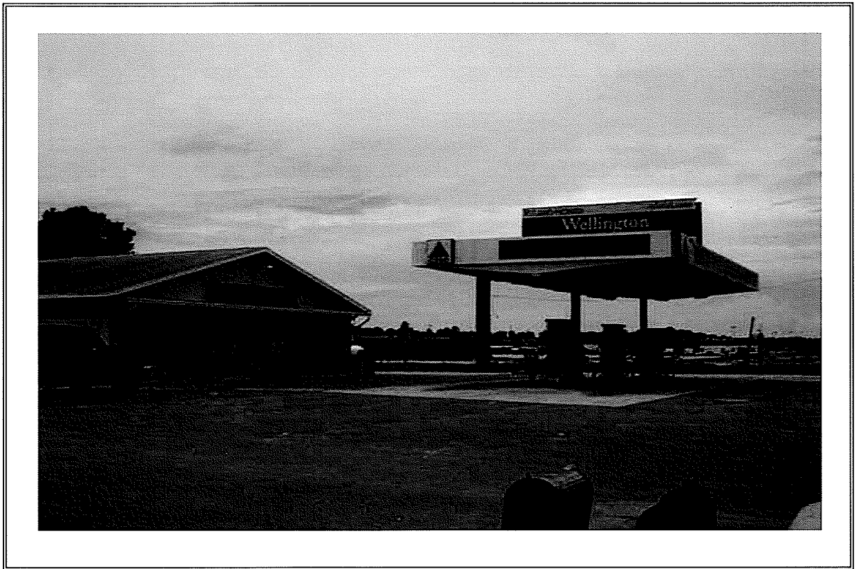
Photo 4. Photo from east showing the Citgo Beverage/Deli gas station (39-P/HM/HW-M) located east of Wal-Mart .
