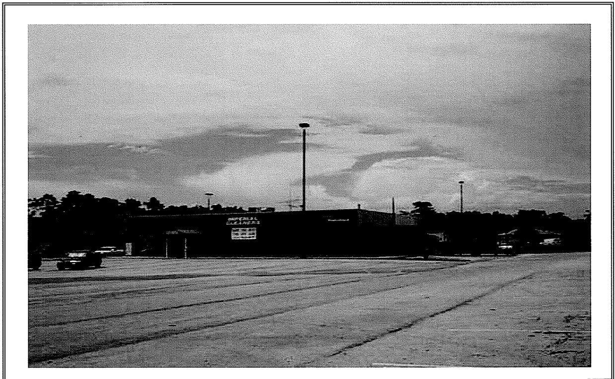
Photo 18. View from the south showing the Imperial Dry Cleaners (former Touch of Quality Cleaners) facility (97-HM/HW-M).
