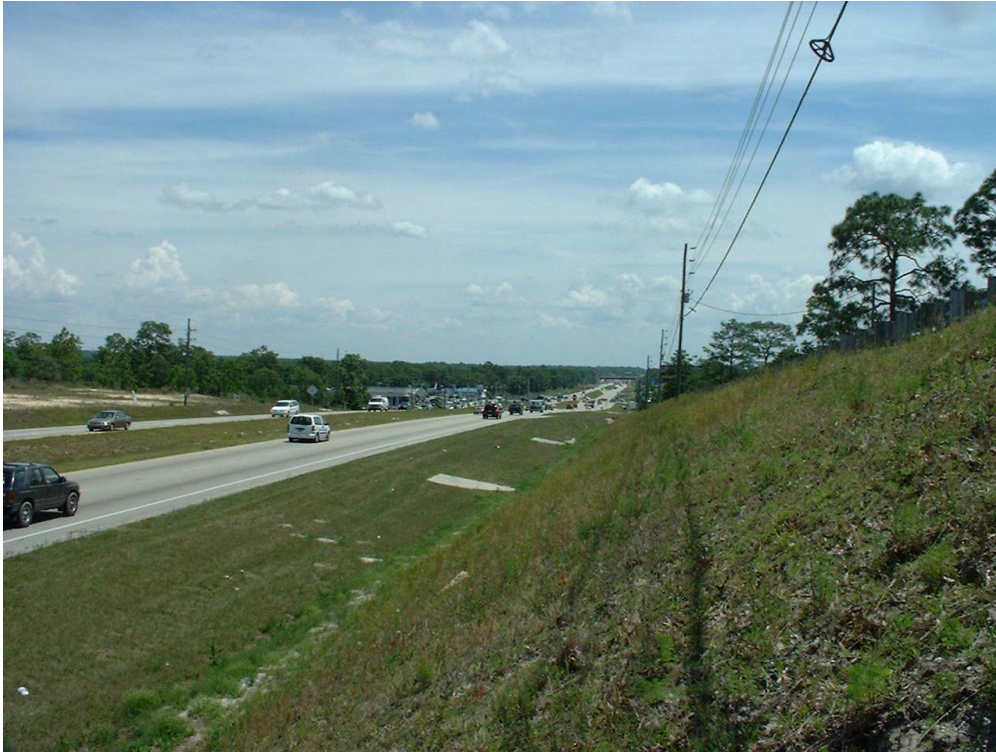
Photo 1.2. Looking Northeast Along S.R. 50.
