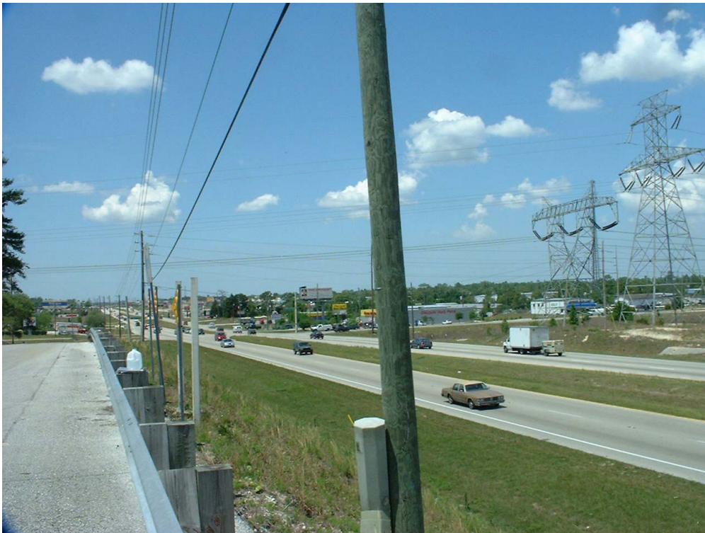
Photo 1.1. Looking Northwest Along S.R. 50.
