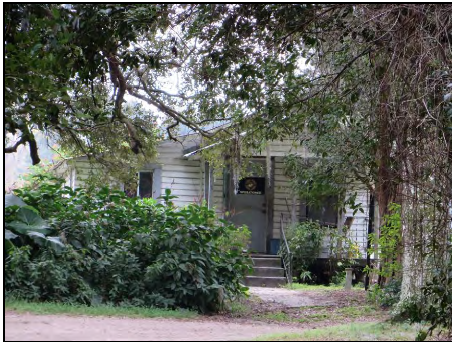
Photo 5-7: North elevation of 35024 Clinton Avenue, 8PA02787, looking south
