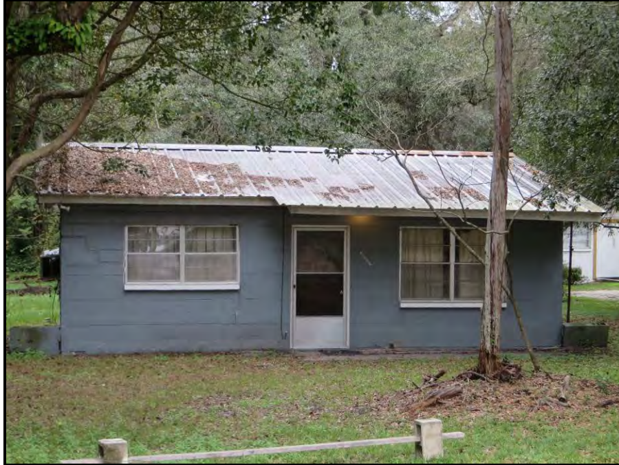
Photo 5-10: South elevation of 31005-A SR 52, 8PA02899, looking north.
