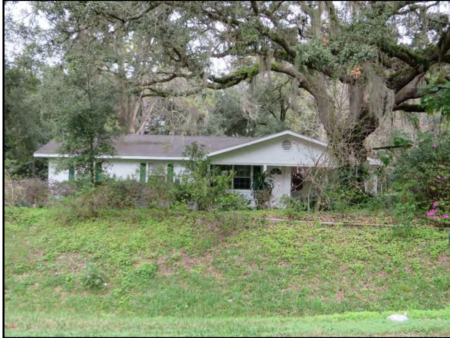
Photo 5-13: South elevation of 36005 Clinton Avenue, 8PA02902, looking north
