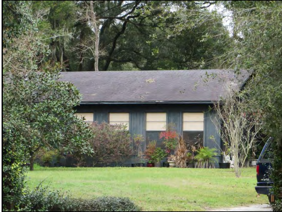
Photo 5-12: South elevation of 35045 Clinton Avenue, 8PA02901, looking north
