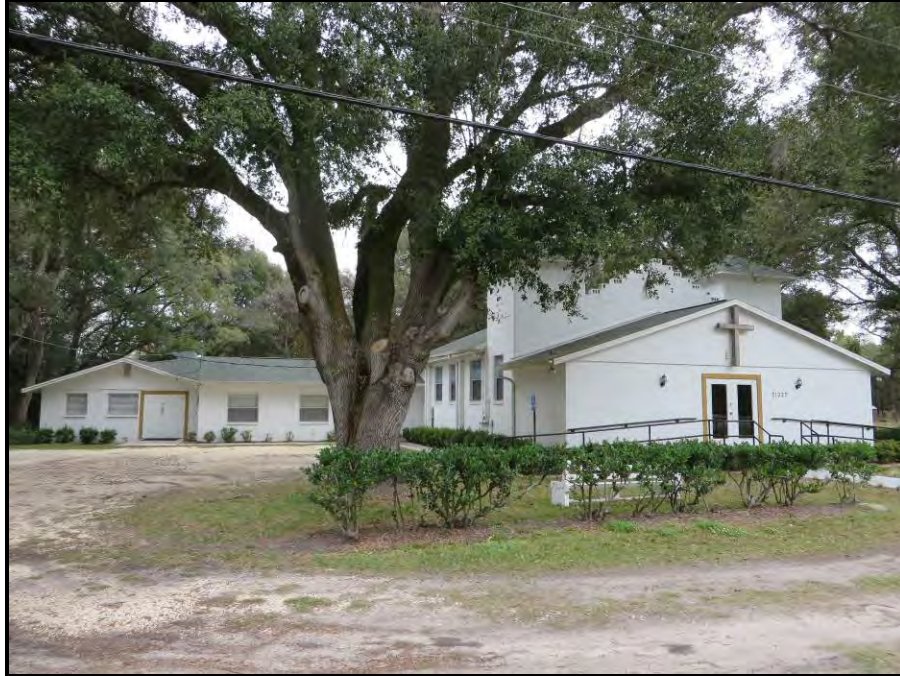
Photo 5-11: South elevation of Piney Grove Missionary Baptist Church, 8PA02900, located at 31027 SR 52, looking north
