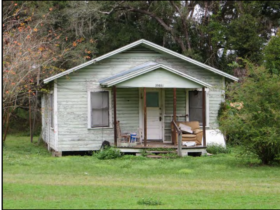
Photo 5-2: South elevation of 35031 Clinton Avenue, 8PA02218, looking north
