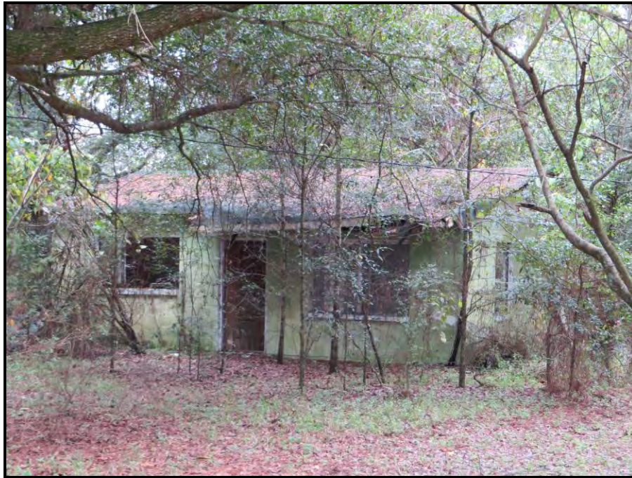
Photo 5-9: Southeast elevation of 31005 SR 52, 8PA02897, looking north.
