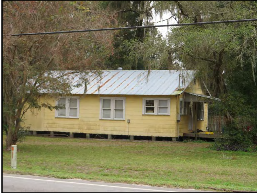
Photo 5-4: West elevation of 35040 Prospect Road, 8PA02785, looking east
