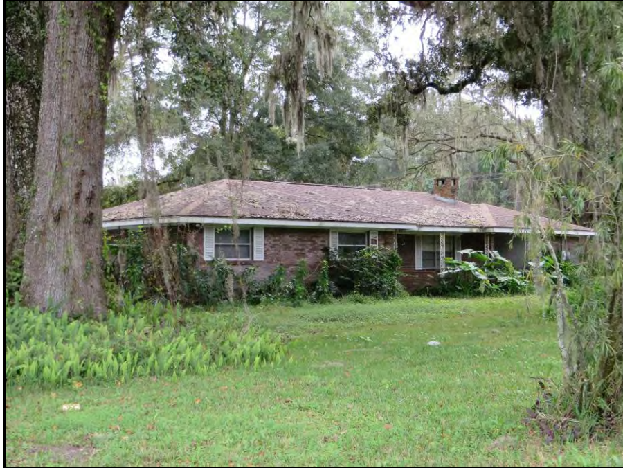
Photo 5-5: West elevation of 35010 Prospect Road, 8PA2786, looking southeast
