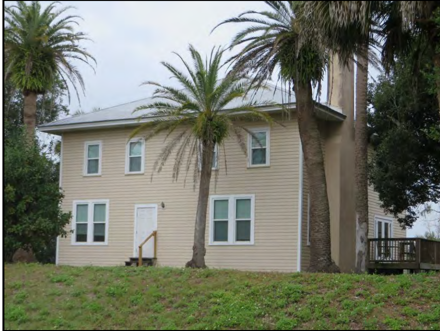
Photo 5-1: South elevation of 35621 Clinton Avenue, 8PA02217, looking north
