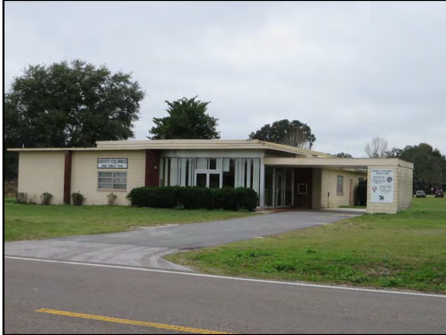
Photo 5-3: East elevation of 11549 Curley Road, (8PA02783), looking west
