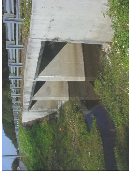
Triple Box Culvert at New River
