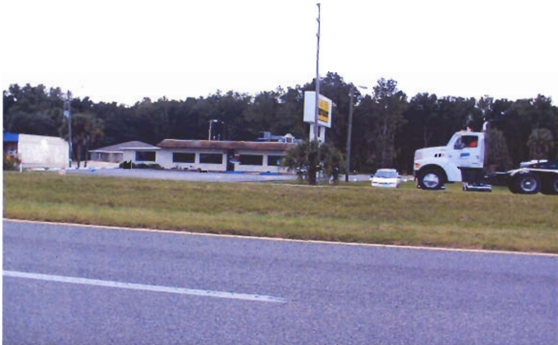
Site 94. Judy Cressey-former gas station, 2051 NW Hwy 19
