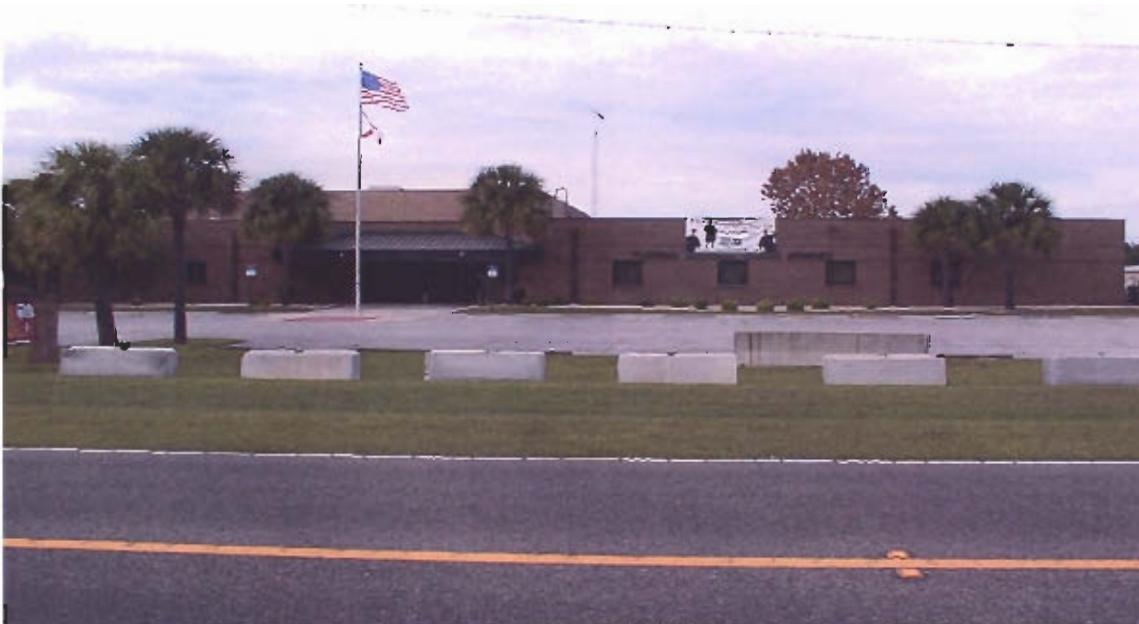
Site 43. National Guard Armory, 8551 W. Seven Rivers Drive.
