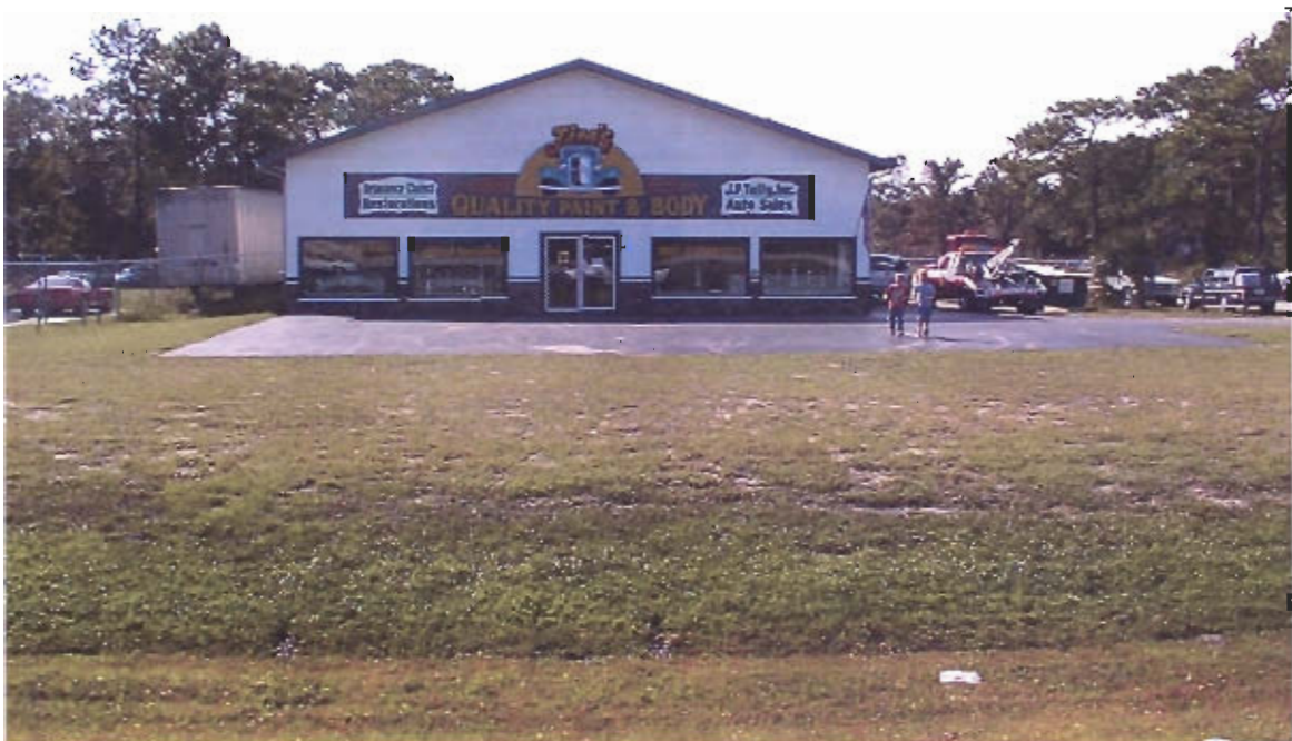
Site 8. Justin Case Auto Repair, 5880 S. Suncoast Blvd.
