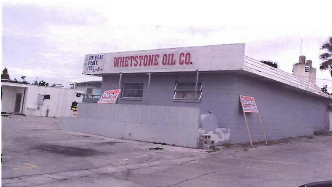
Site 60. Florida Power Corp.-Whetstone Oil Unit #5, 1017 US Hwy 19.
