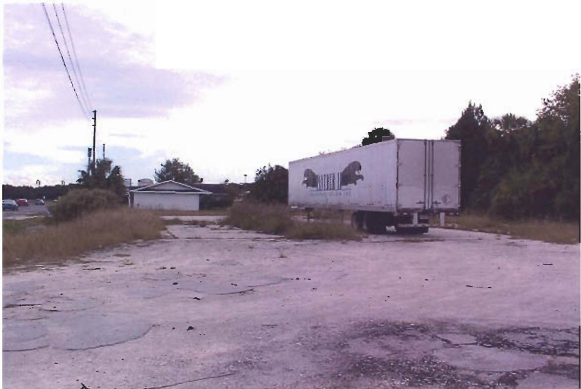
Site 44. Former gas station pump island, 548 N. Suncoast Blvd.
