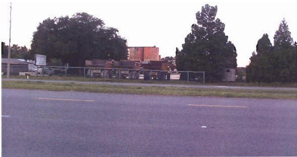
Site 104. Crystal River Quarries, Inc., 7040 N. Suncoast Blvd.
