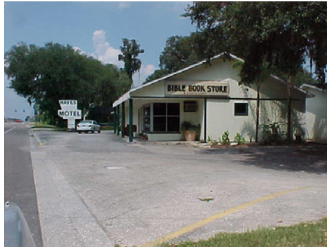
View of Book Store - south end of building
