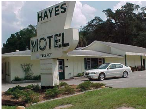
View of Motel office on north end of building
