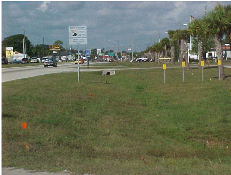
Photo 15 Station 704+10, 40 RT. Looking north on US 19 North Bound ROW.
