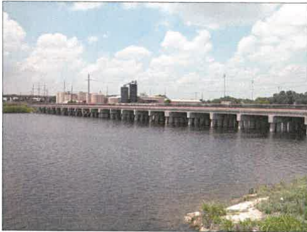
Figure 1 CSX Railroad upstream
