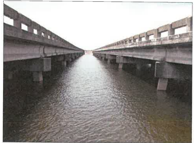
Figure 7 SR 60 looking west between spans
