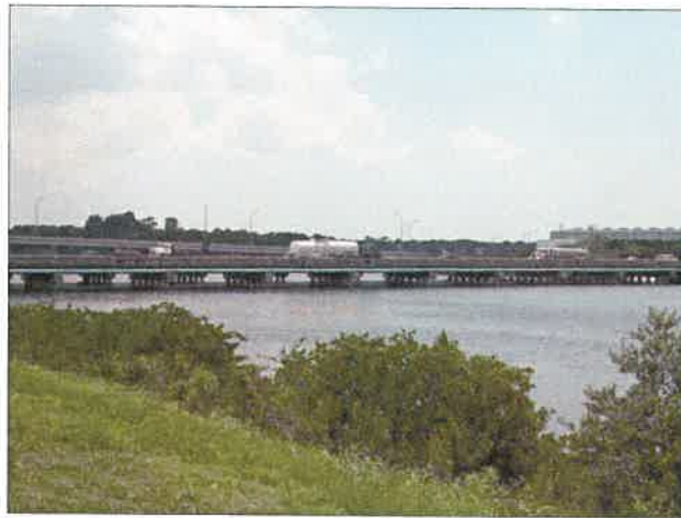
Figure 3 SR 60 looking south at spans
