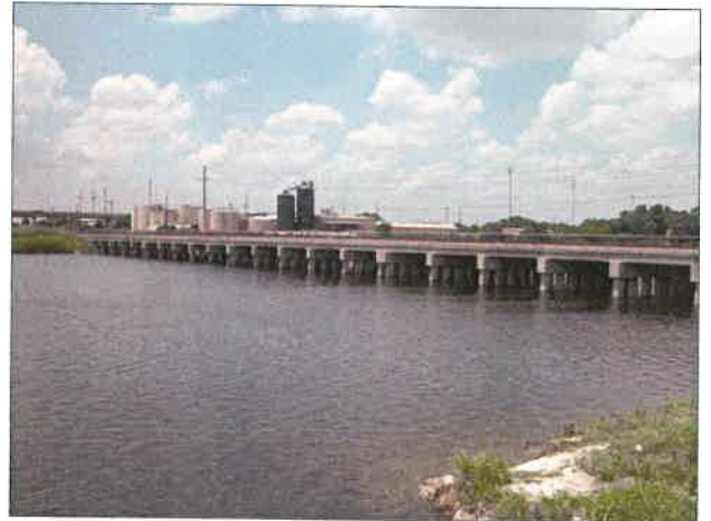
Figure 14 SFWMD Tampa Bypass Canal lock from CSX
