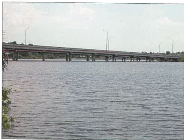
Figure 15 Leroy Selmon Expressway looking south from SR 60
