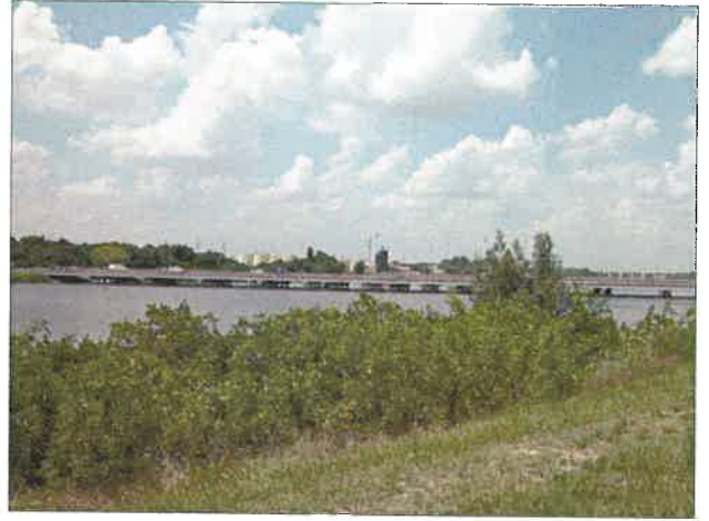
Figure 12 South of SR 60 looking north
