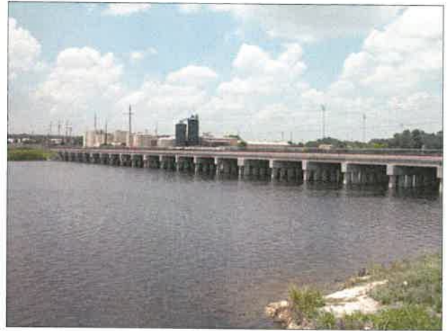
Figure 5 CSX Railroad upstream
