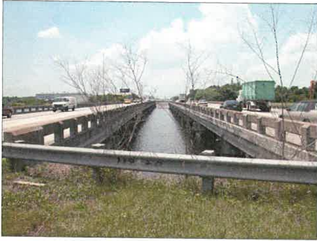
Figure 11 SR 60 looking west
