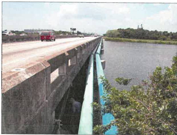
Figure 9 Eastside of SR 60 looking west
