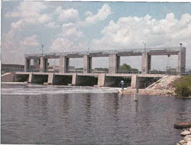
Figure 6 SFWMD lock upstream from CSX Railroad
