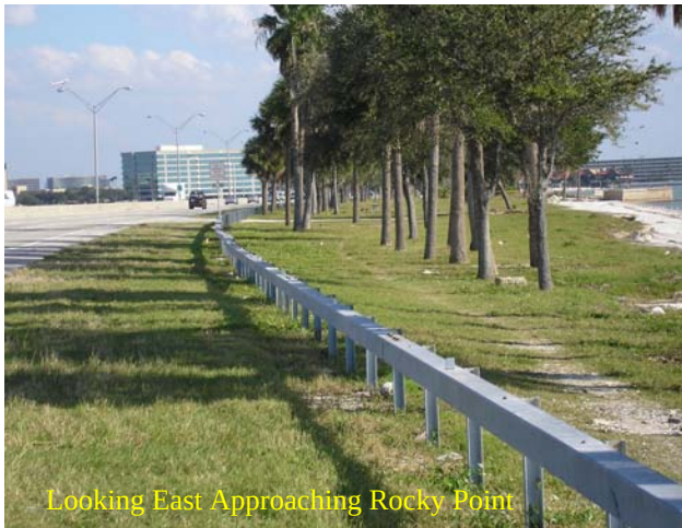
Access Road Southside Between Structures 1 & 2
