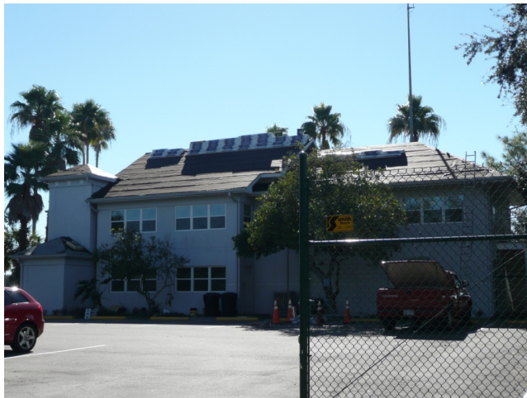
Photo 5-2 North Elevation of 3204 Gulf to Bay Boulevard, 8PI11966
