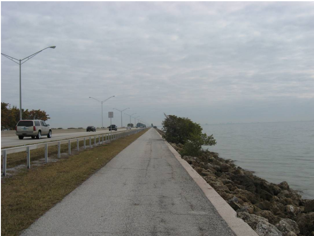
Picture 2 – Typical along south side of Causeway located east of Structure 1
