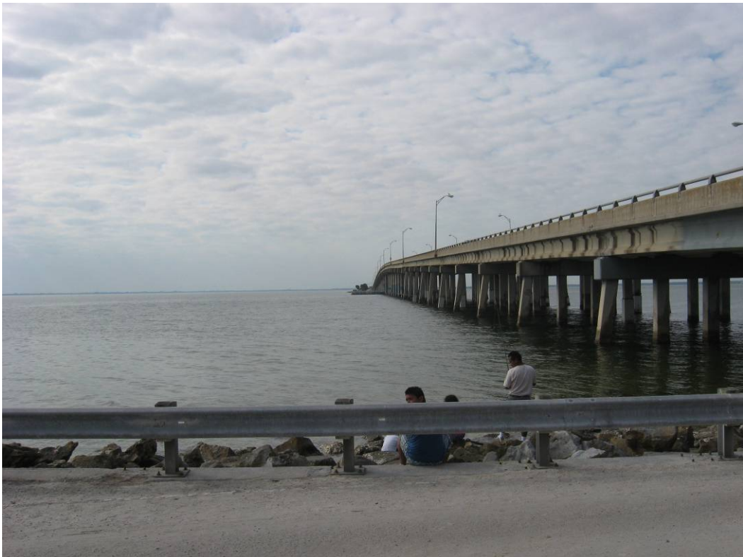
Picture 4 – East side of Structure 2 facing toward the west
