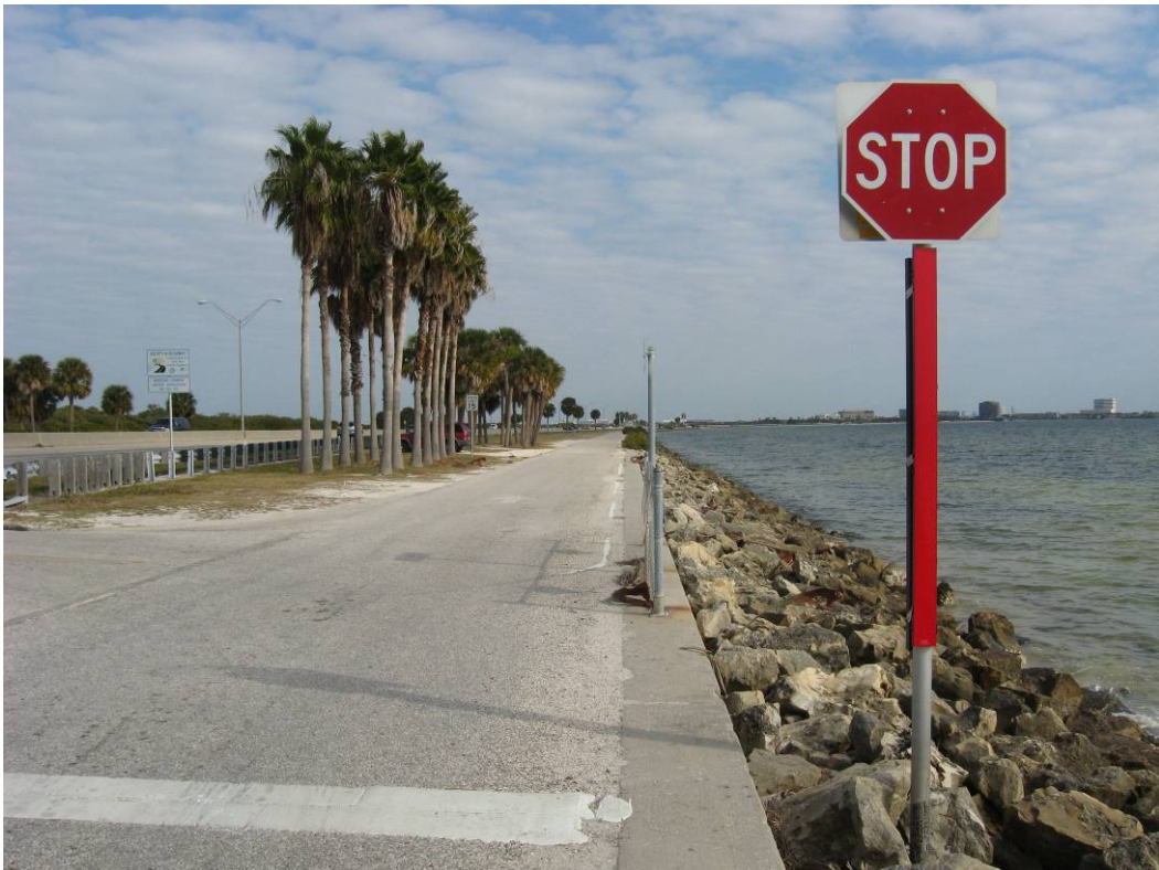
Picture 6 – Entrance near boat ramp on south side of Causeway facing east
