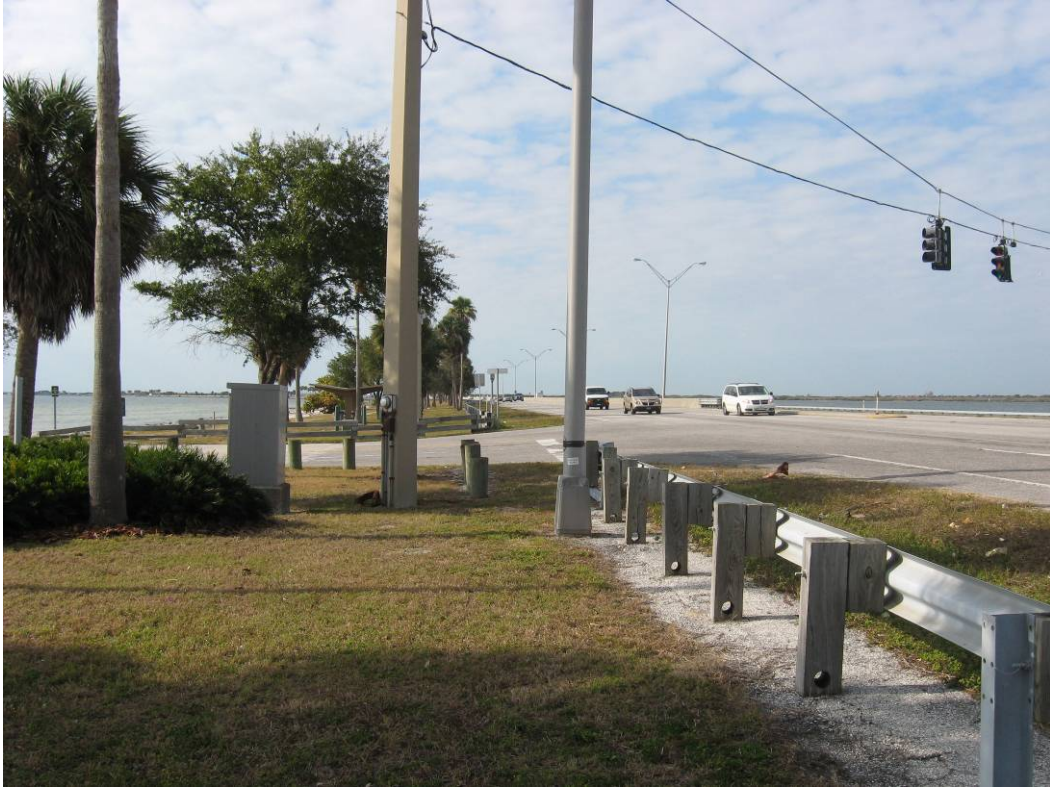
Picture 9 – West entrance of Ben T. Davis Beach, eastern terminus of project
