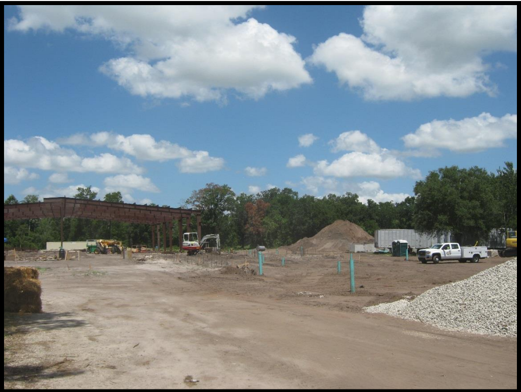
Photo 58: FPC-12, construction in progress, facing west toward SMF 15
