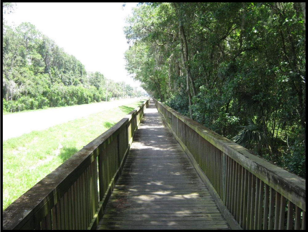
Photo 7: Typical elevated walkway located along stretches of US 92 west of Plant City
