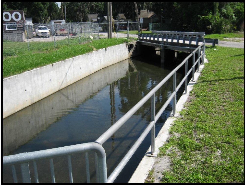
Photo 1: Hardened canal near N. Vermont St. and US 92
