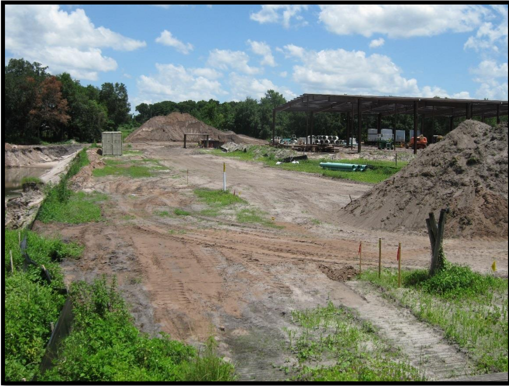
Photo 31: SMF 15, SMF site and construction of adjacent pond
