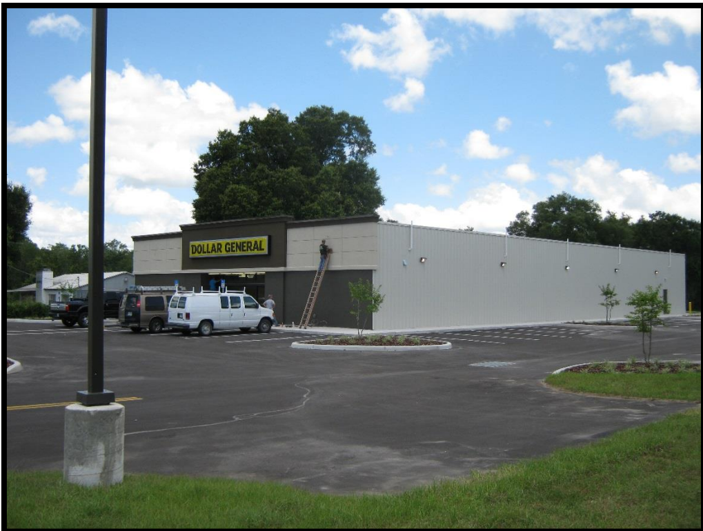
Photo 64: FPC-14B, newly constructed Dollar General
