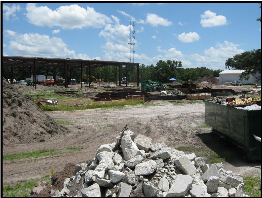
Photo 30: SMF 15, site has been cleared with construction in progress
