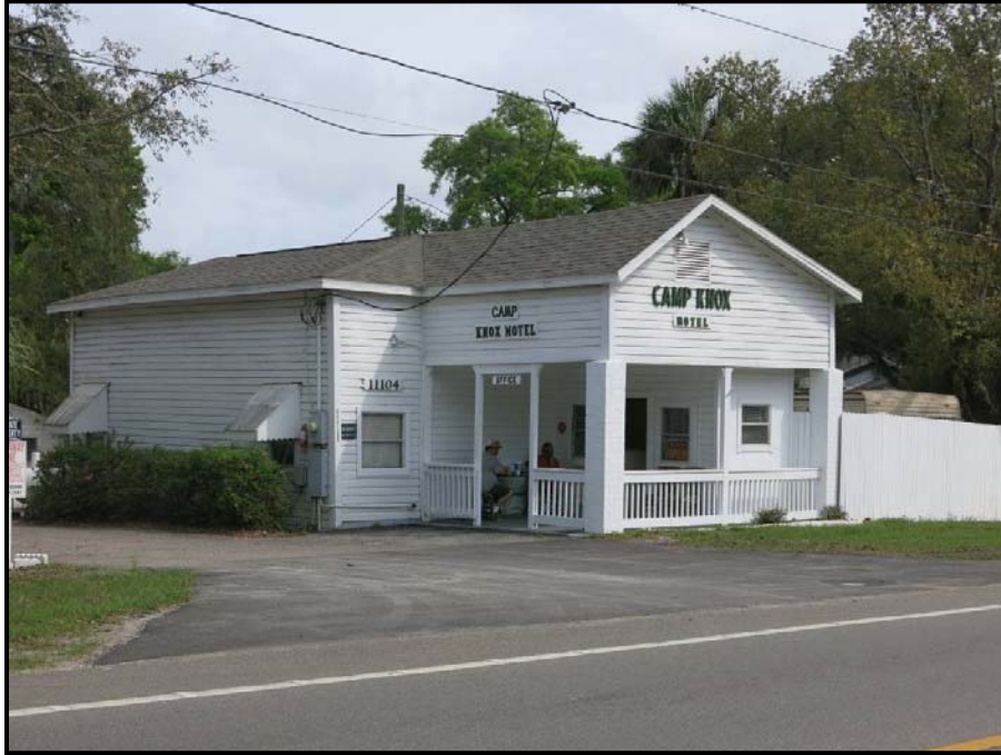
Photo 4-3. Camp Knox Main Building (8HI13032) at 11104 E. SR 600 (US 92) Highway, looking northeast.
