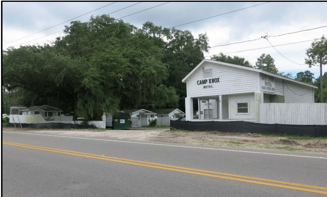
Photo 6-1. Approximate location of the noise barrier wall.
