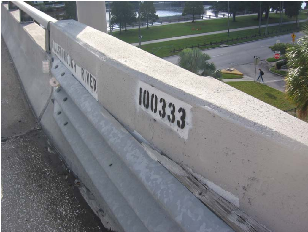
PHOTO 10 – 10/07/09 – SAMPLE TCLP-03 GRAY PAINT ON STUCCO ON CONCRETE
