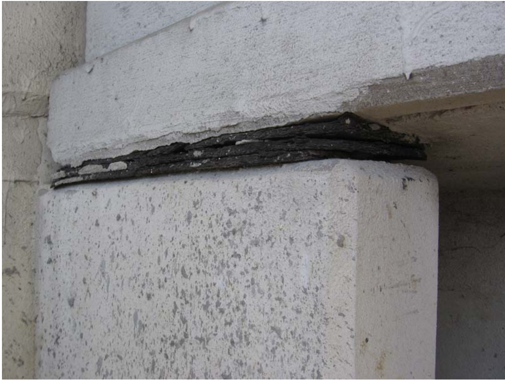
PHOTO 9 – 10/07/09 – SAMPLE TCLP-02 BEIGE PAINT ON CONCRETE
