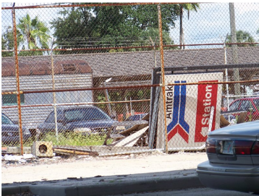
15. CSX/Amtrak Station. Site ID 6.
