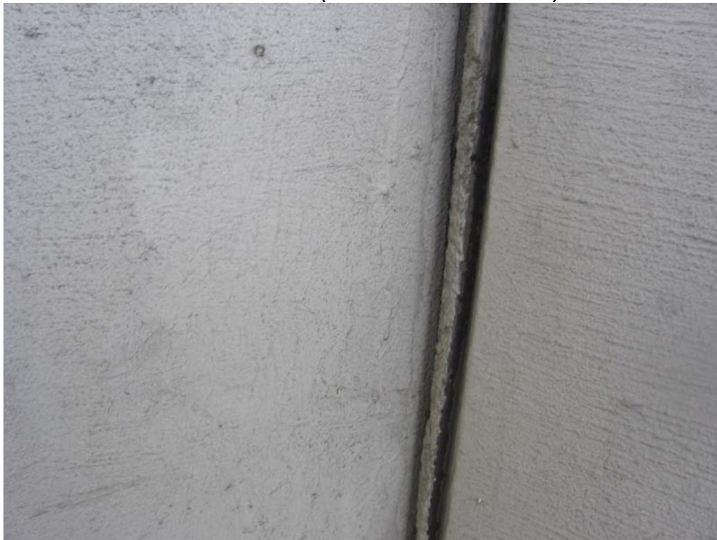
PHOTO 12 – 10/02/09 – SAMPLE TCLP-01 LIGHT GRAY/WHITE PAINT ON CONCRETE
