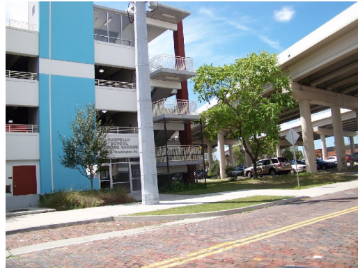
8. Hills. Cty Parking Garage.
