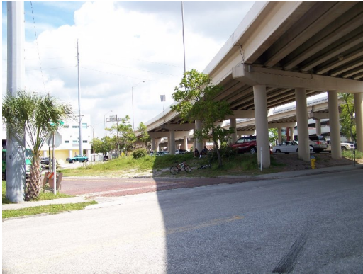
3. Cumberland Ave Under Crosstown
