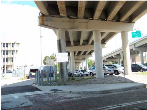
7. View Under Crosstown
