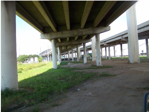
21. Crosstown near International Ship. Site ID 10
