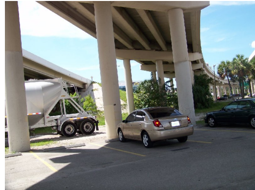
4. View under Expressway near Con Agra. ID 3
