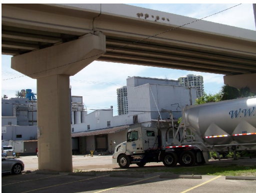
5. View of Con Agra Near Expressway. Site ID 3
