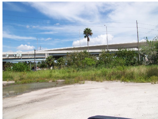
16. View of Channel side Spill Site. Site ID 8
