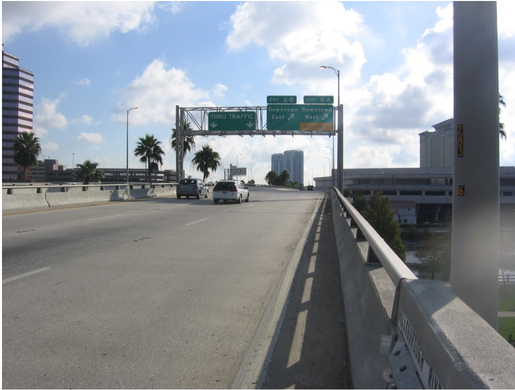
PHOTO 1 – 10/07/09 BRIDGE 100333 – LEE ROY SELMON CROSSTOWN EXPRESSWAY EASTBOUND FROM EXIT 5 TO EXIT 9 TAMPA, HILLSBOROUGH COUNTY, FL
