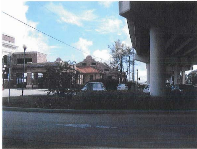
Photo 5-3: South elevation of the Union Station Baggage Building in the background.
