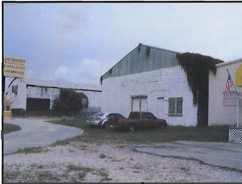
Photo 5-8: South elevation of 1807 East 2nd Avenue, 8HI6841
