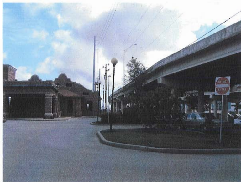
Photo 5-4: The Expressway in relation to the Baggage Building.
