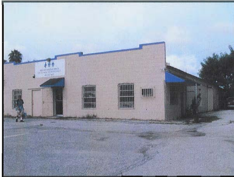
Photo 5-5: East and north elevations of 704 North 13 th Street, 8HI6838
