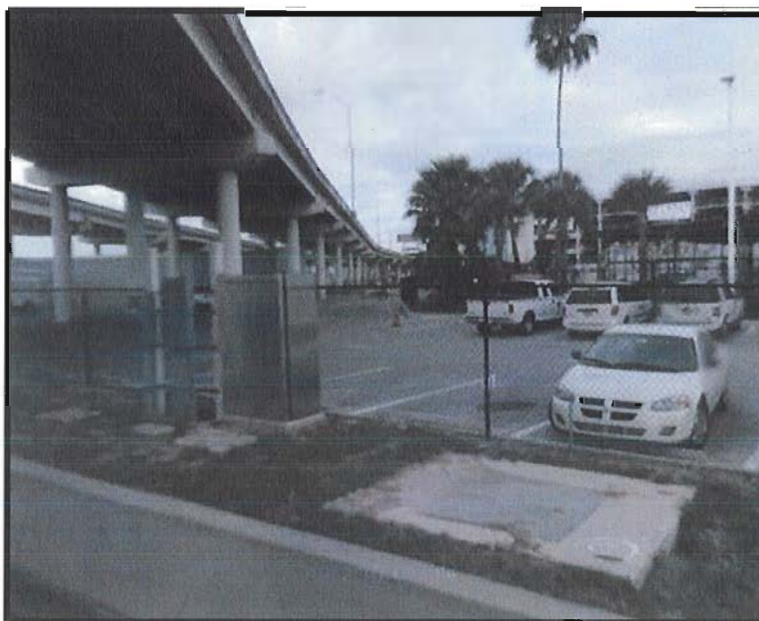
Photo 5-1: Former location of 611 North Meridian Avenue, 8HI6835
