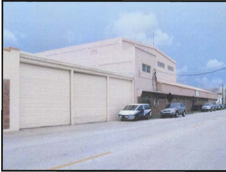
Photo 5-7: North elevation of 1405-1411 East 2 nd Avenue, 8HI6840
