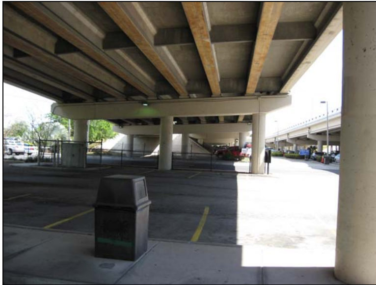
Figure 2-27 Typical Two-Column Pier
