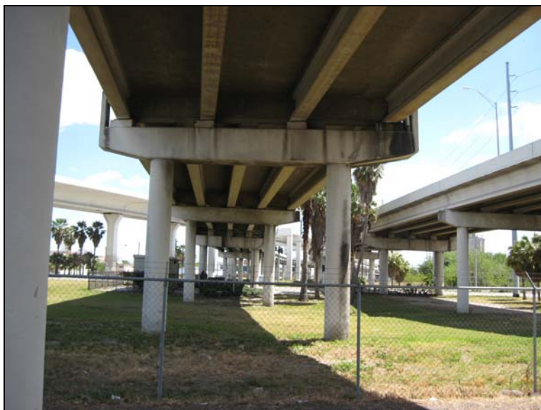
Figure 2-27 Typical Two-Column Pier
