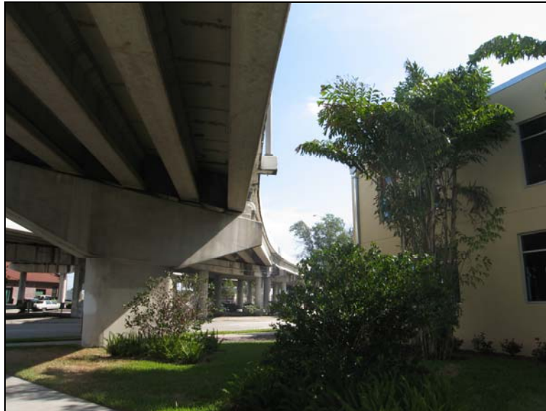
Figure 2-28 Typical Single-Column Pier
