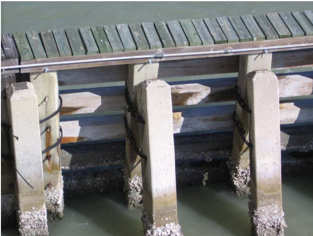
PHOTO 70 – 01/21/09 – SAMPLE 29.2 – HA 29 CONCRETE PILINGS/PIERS AT WOOD FENDERS
