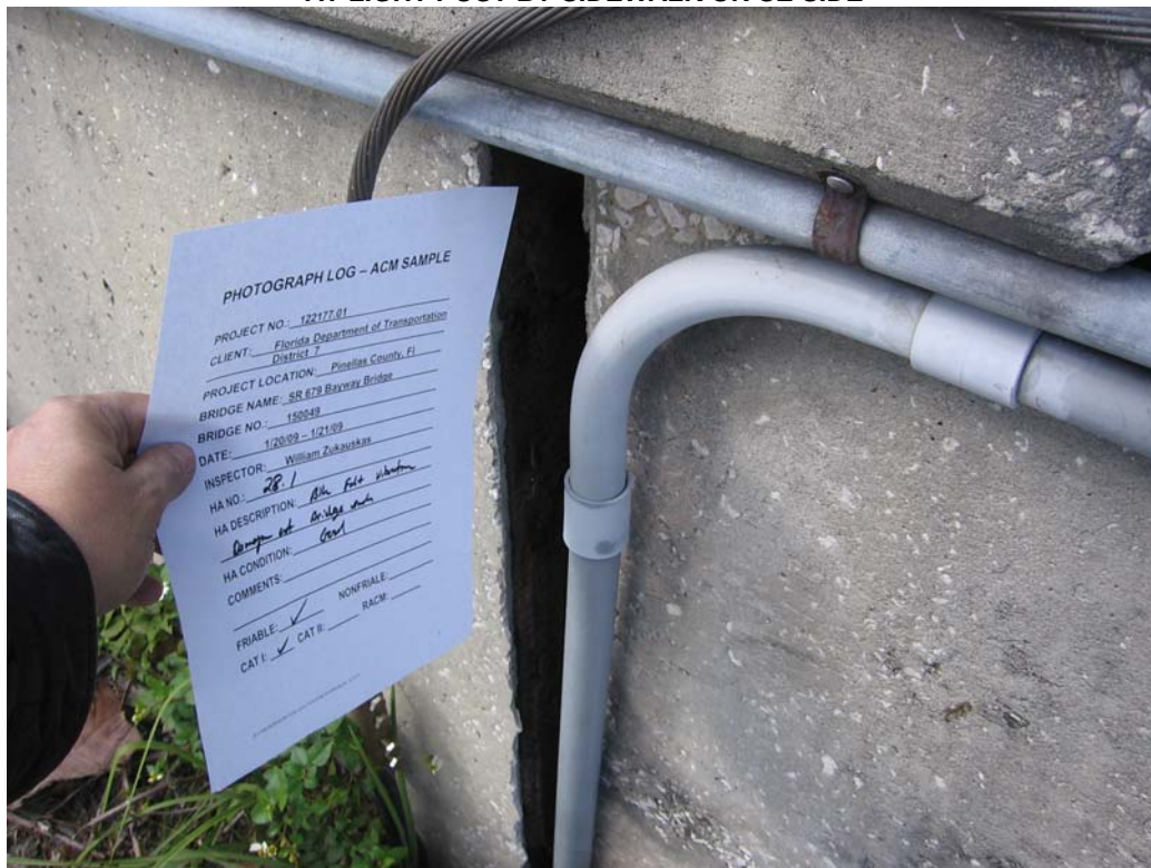
PHOTO 66 - 01/21/09 - SAMPLE 28.1 - HA 28 BLACK VIBRATION DAMPERS AT NORTH AND SOUTH BRIDGE ENDS
