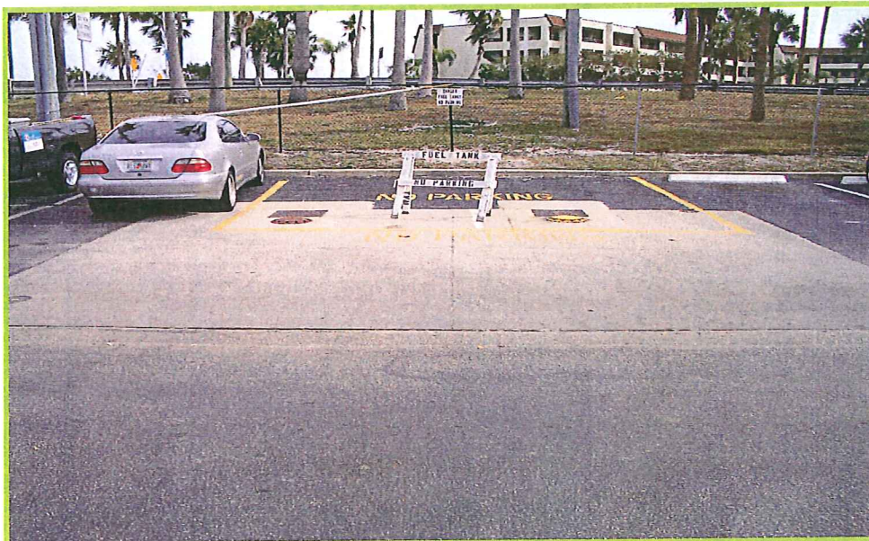
Photo 10 – View of Texaco-Tierra Verde Marina/BP Station – Site No. 4 – Close-up view of underground fuel storage tank farm located west of S.R. 679 (station 278+00)
