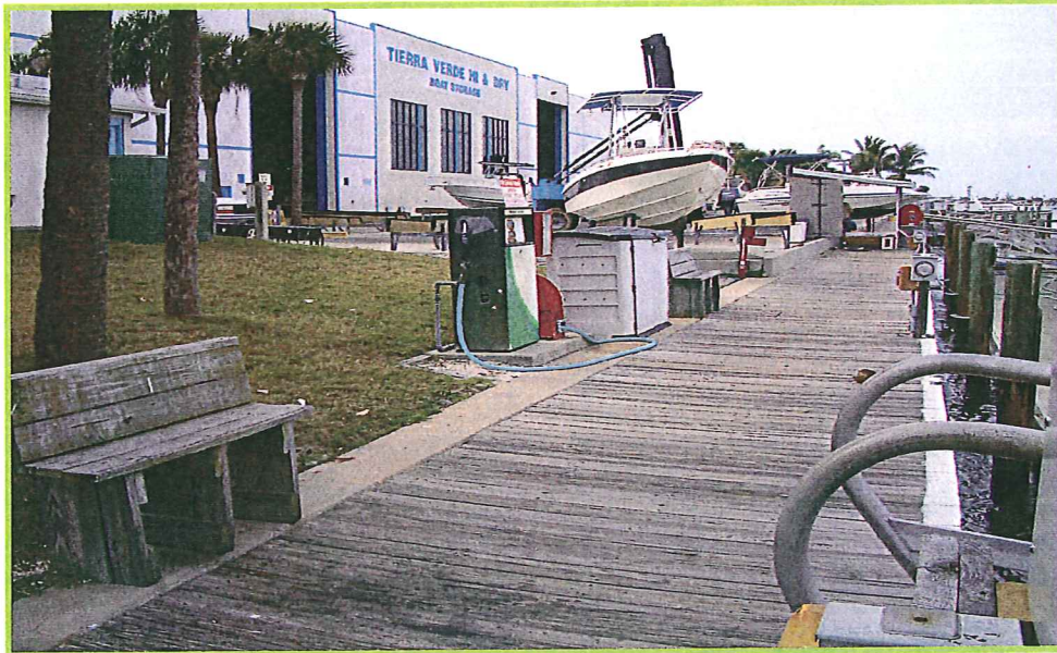
Photo 15 - View of Texaco-Tierra Verde Marina/BP Station – Site No. 4 – Close-up view of pumps located west of S.R. 679 (station 279+00)
