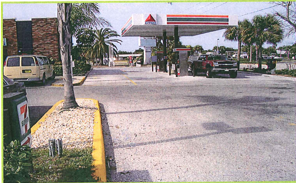
Photo 5 - View of 7-11 Food Store No. 29301 – Site No. 2 – View of the pump islands located west of S.R. 679 (station 270+50)
