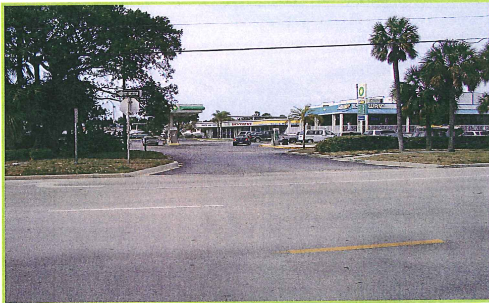
Photo 7 - View of BP Station, Texaco-Tierra Verde Marina – Site No. 4 – View of adjacent property to the west of S.R. 679 (station 273+00)
