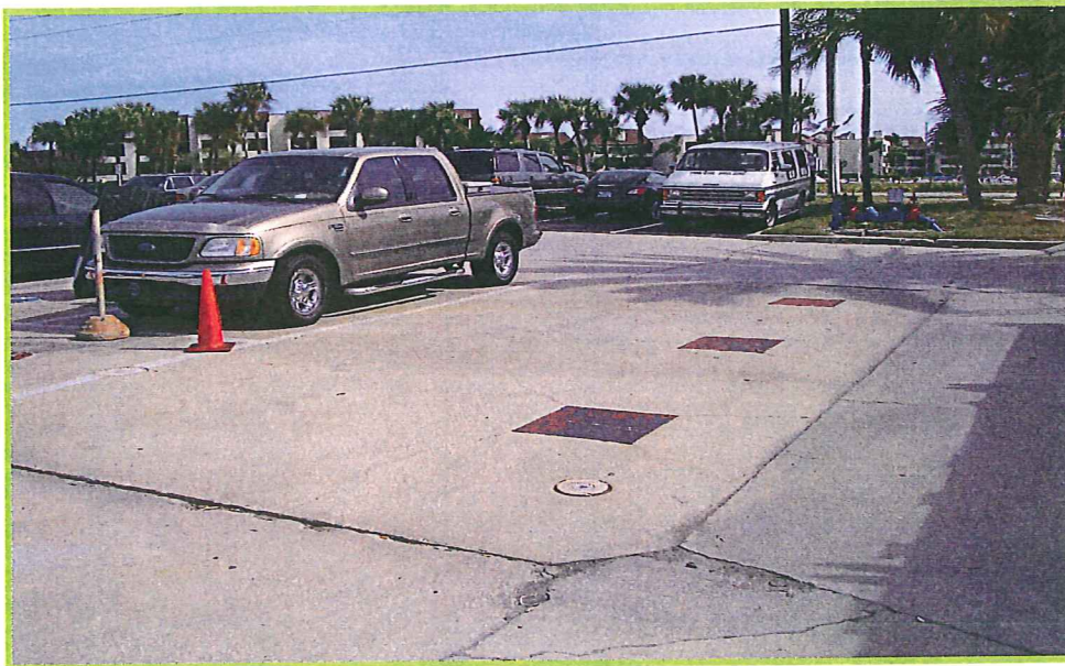
Photo 4 – View of Tierra Verde Resort & Marina – Site No. 1 – Close-up of monitoring wells and the underground fuel storage tank farm area located west of S.R. 679 (station 268+50)
