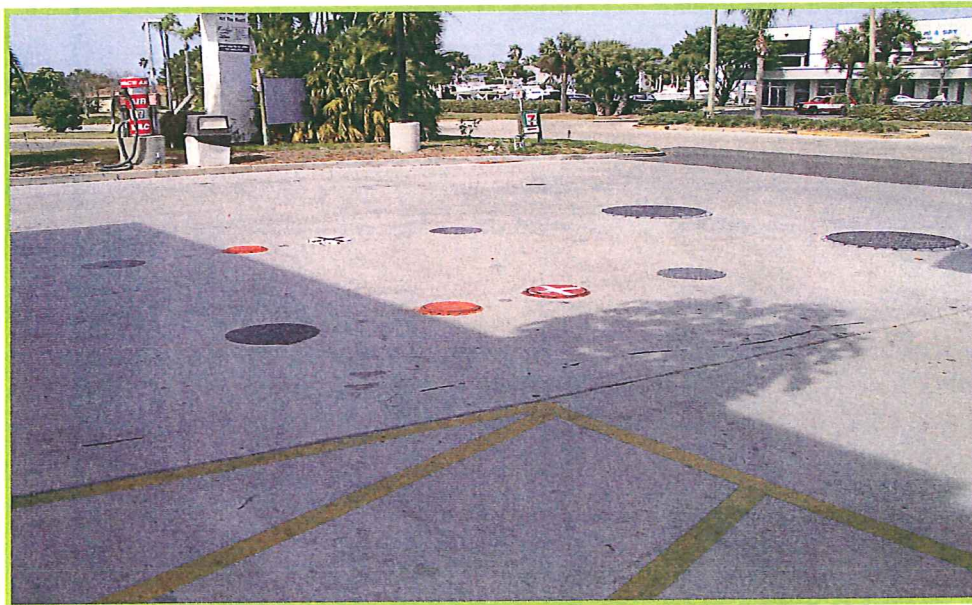
Photo 6 – View of 7-11 Food Store No. 29301 – Site No. 2 – View of the underground fuel storage tank farm area located west of S.R. 679 (station 270+50)
