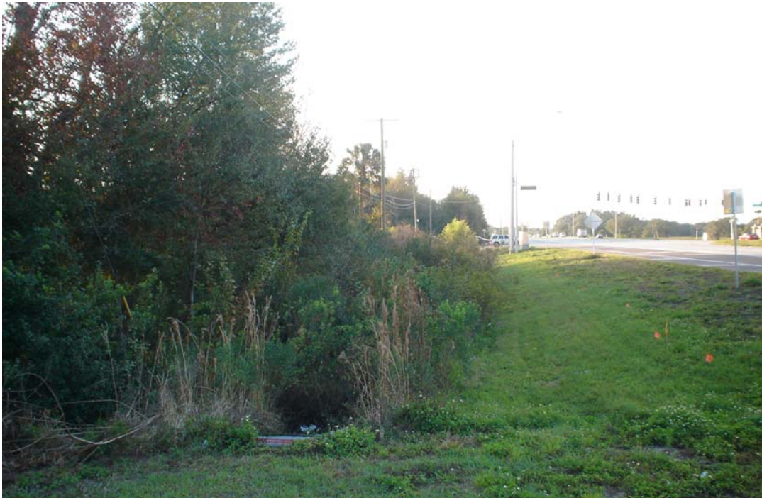
Photo 5 : Swale in front of 7-Eleven, facing south
