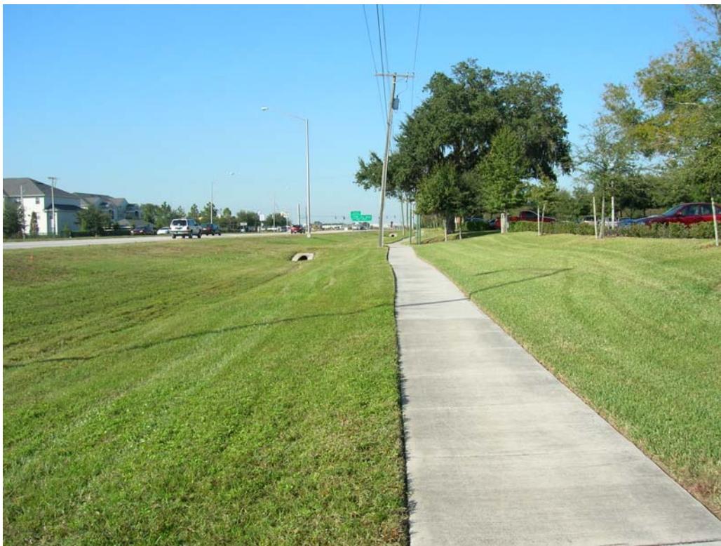
Figure 10: Parallel Berm and Ditch in the Existing U.S. 301 Right-of-way, Facing North
