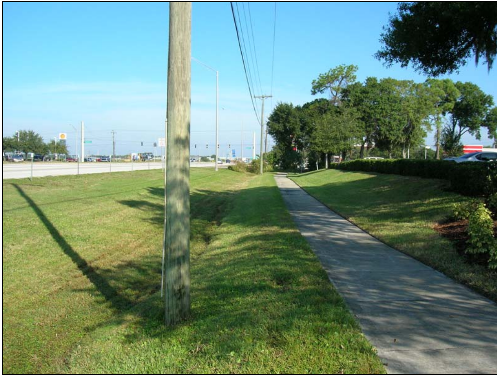
Figure 9: Parallel Berms and Ditch in the Existing U.S. 301 Right-of-way, Facing North
