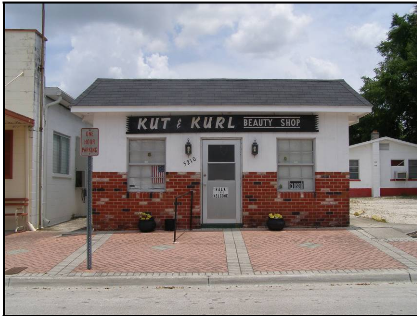
Photo 4-1. Southwest elevation of 5210 7 th Street, 8PA2742, looking northeast.
