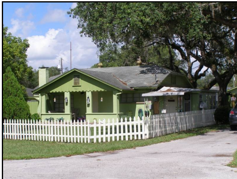
Photo 4-11. North and east elevations of Building 1, 3927 Old Crystal Springs Road (8PA1164).
