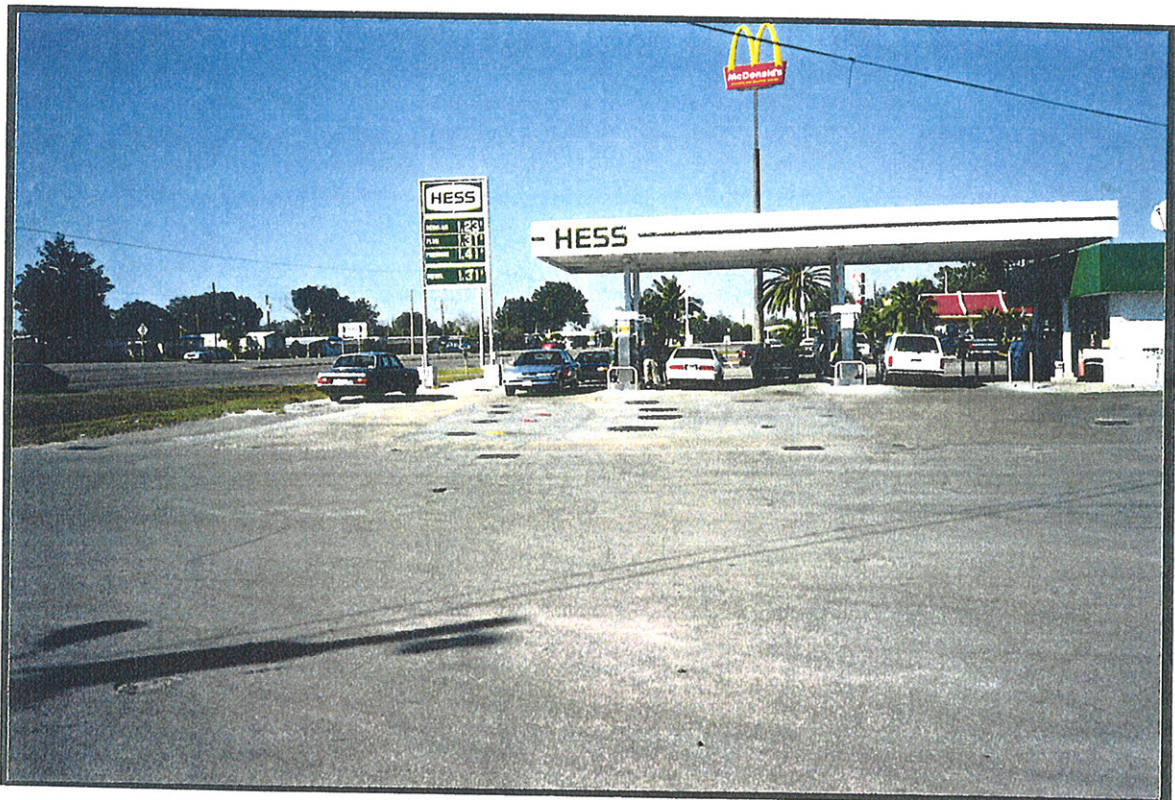
Photo #33-Hess #09415 (Former Pick Kwik #144)- view north of UST area, recovery wells.
