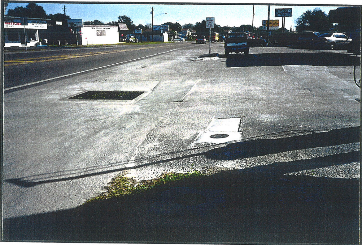
Photo #31-Circle K #0180– view south along US301. Note monitor wells adjacent to ROW.
