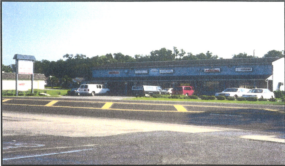
Photo #21-Strip Plaza (former gas station)- looking east at site.
