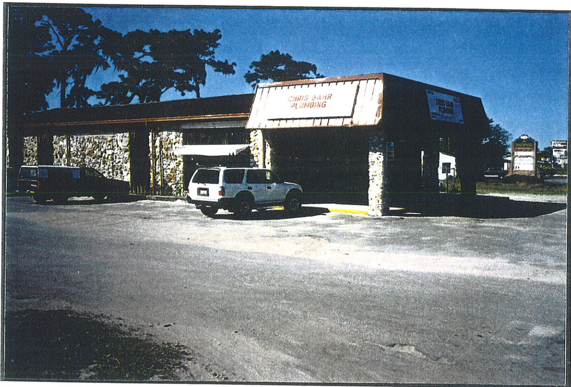
Photo #29-Chris Bahr Plumbing- view NW at building. Note vent pipe on side of building.
