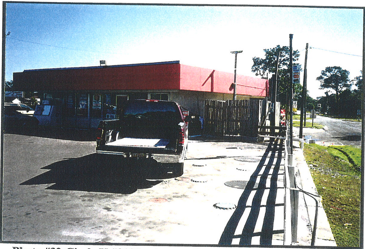
Photo #32-Circle K #0180– view south of UST's, remedial system in privacy fenced area. 6th Street visible in right of photo.
