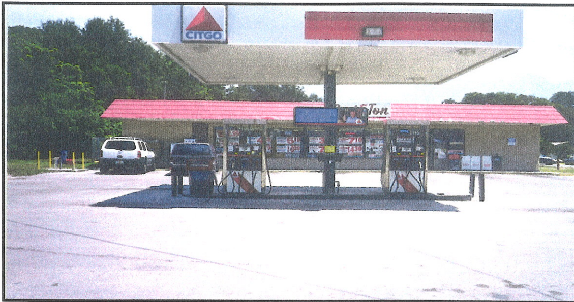
Photo #9-Sav-a-Ton/Citgo- view east at pump island store
