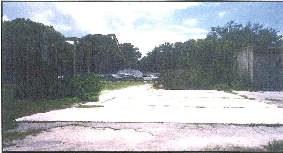
Photo #11-Former Texaco Station- view south along east side of site at 5 UST's
