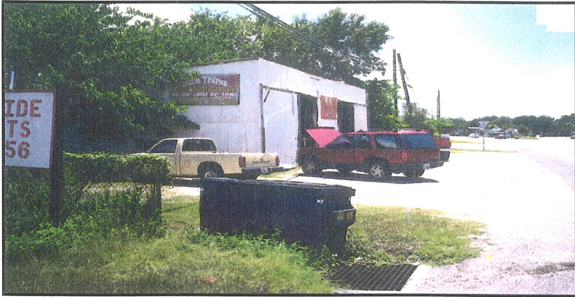
Photo #3- Sure Thing Auto Repair-view south at site, note closeness to right-of-way
