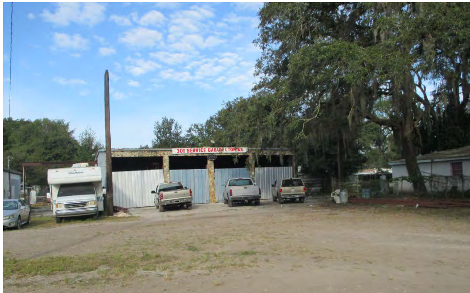
14. View to the northwest across Site No. 11 – 301 Service Garage & Towing (former Power’s Garage)
