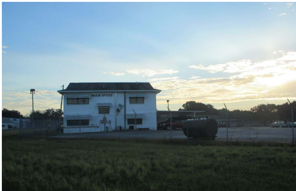
4. View to the northeast of main office building located on the southern portion of Site No. 4 - Festival Park
