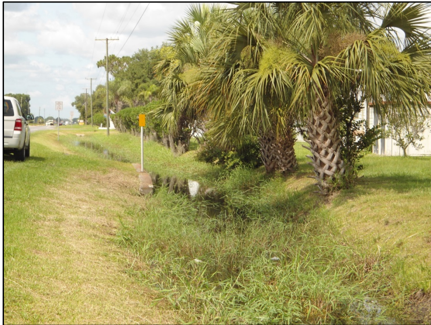
Photo 14: Ditch 4 facing south. FLUCFCS: 510 – Streams and waterways
