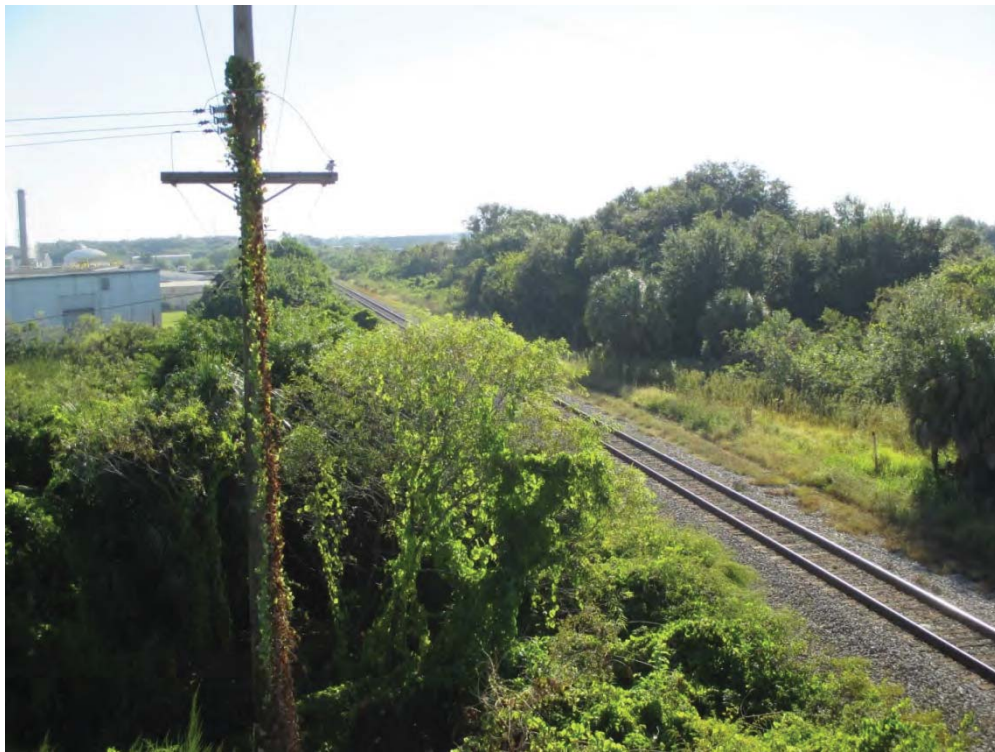
6. View to the east along Site No. 14 – Railroad CSXT Mainline (South)
