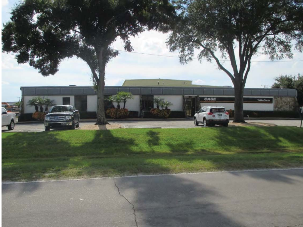
15. View to the west of Site No. 26 – Case Construction (1504 Tampa East Boulevard)
