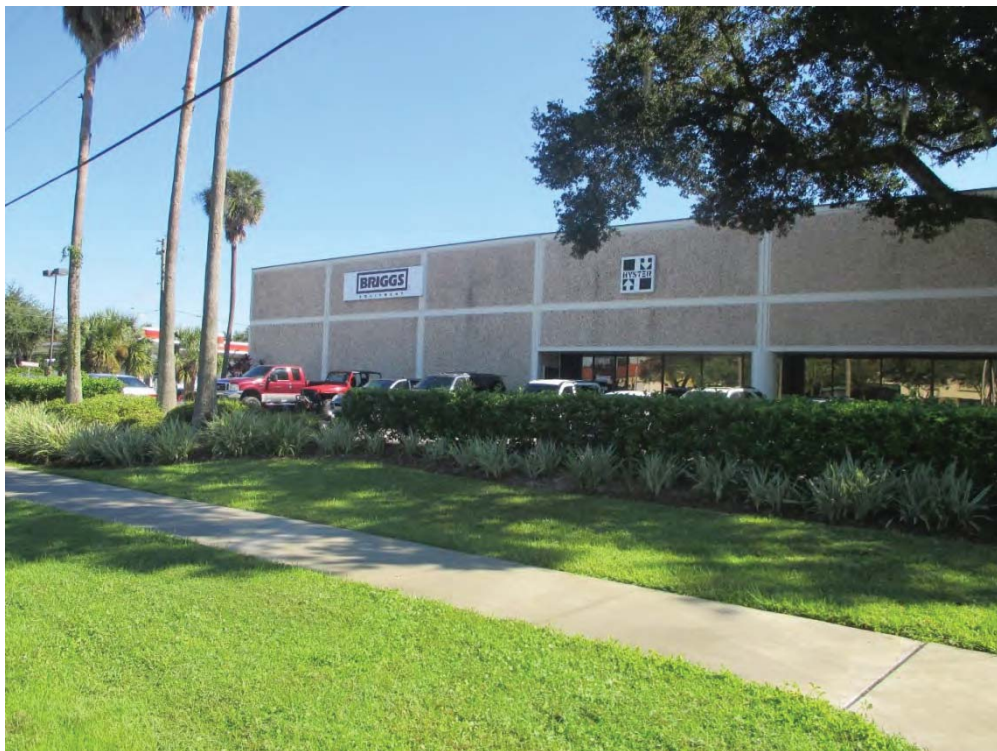
38. View to the northeast of site No. 54 – Briggs Equipment (3915 US 301)
