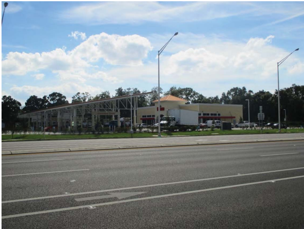
40. View to the south across Dr. Martin Luther King Jr. Boulevard, towards Site No. 56 – Wawa #5114
