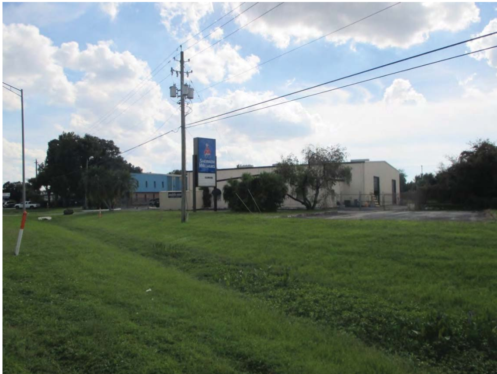
20. View to the southwest towards Site No. 32 – Sherwin Williams (1926 US 301)
