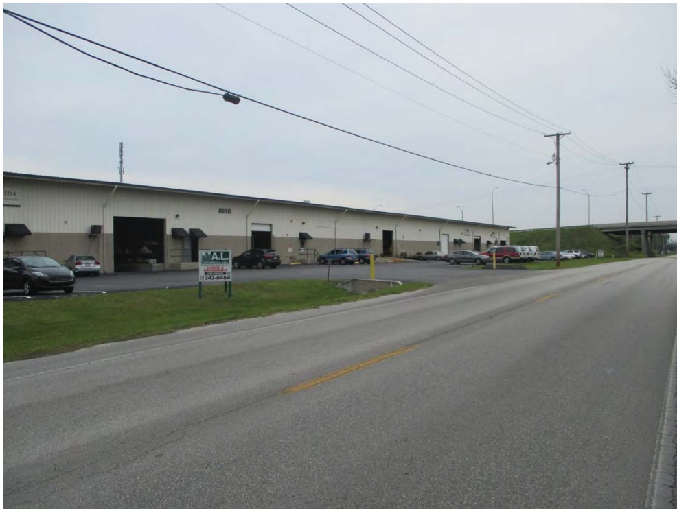
26. View to the northeast across Broadway Avenue, towards Site No. 40 – Unique Granite (8100 Broadway Avenue)
