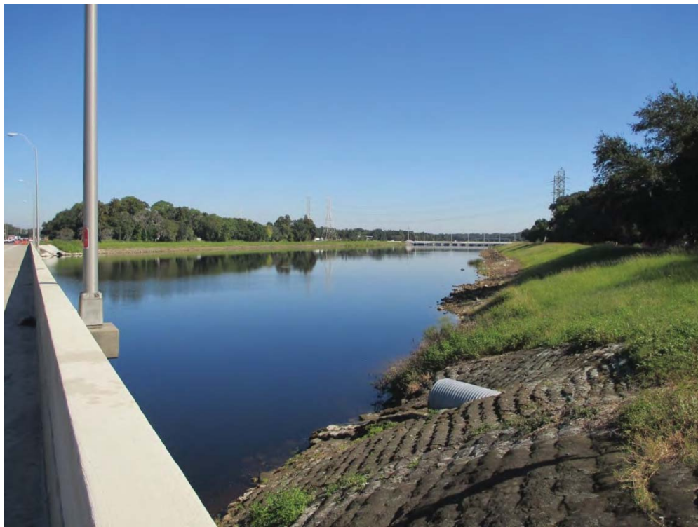
34. View to the northeast across Tampa Bypass Canal
