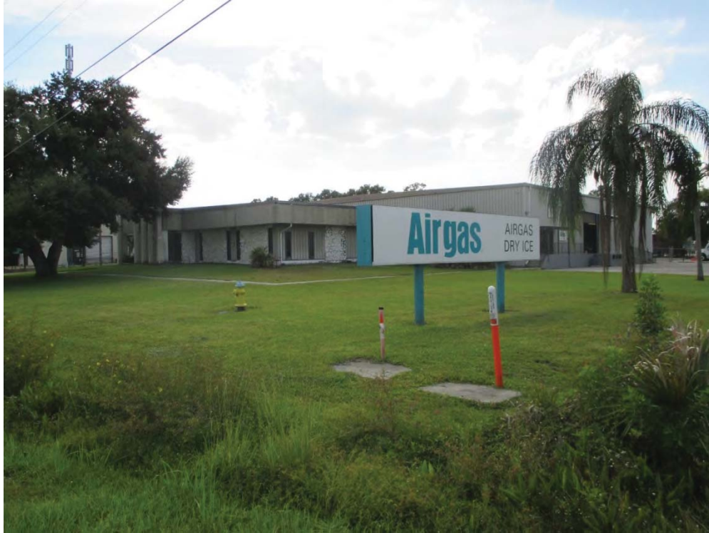
27. View to the southwest of Site No. 42 - Airgas Dry Ice (2914 US 301)
