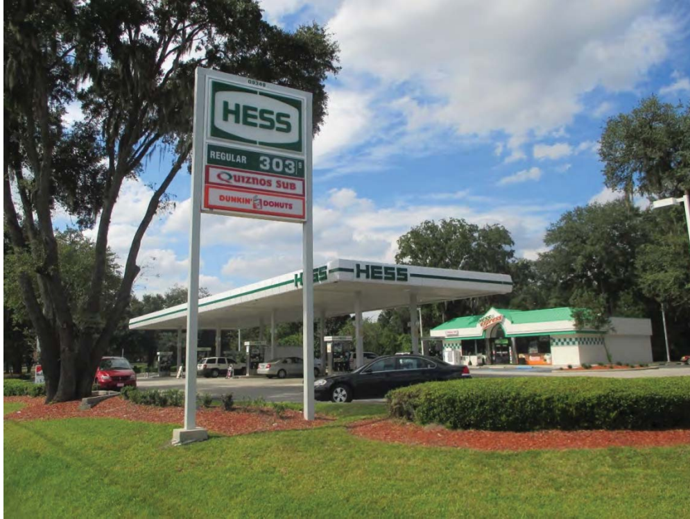
41. View to the northwest across Site No. 60 – HESS #09348 (8350 Dr. Martin Luther King Jr. Boulevard)
