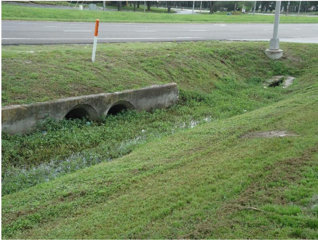
Double 36" Cross Drain at Station 147+11
