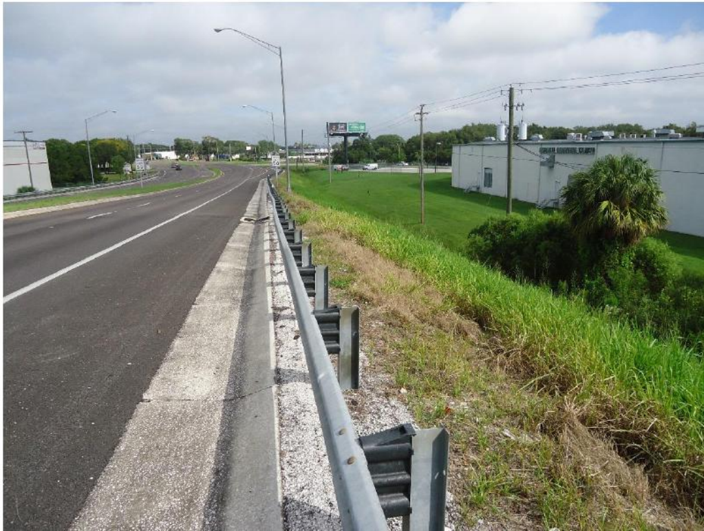
Swale/Ditch adjacent to Overpass Shoulder Gutter on Overpass
