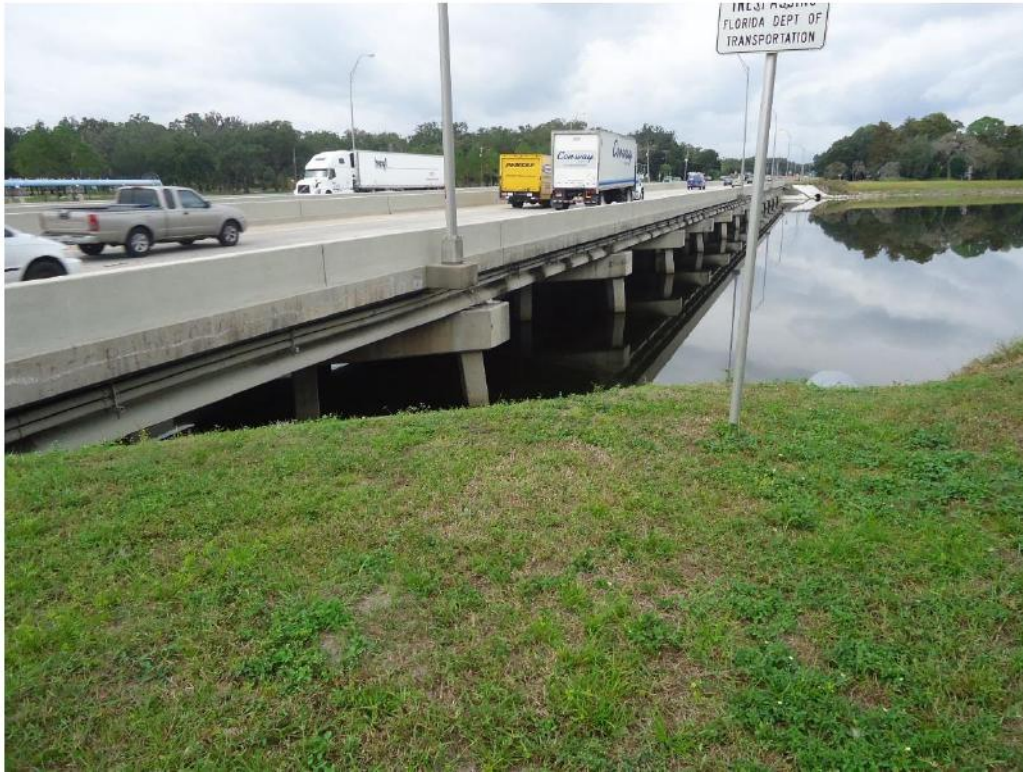
Bridge Over Tampa Bypass Canal
