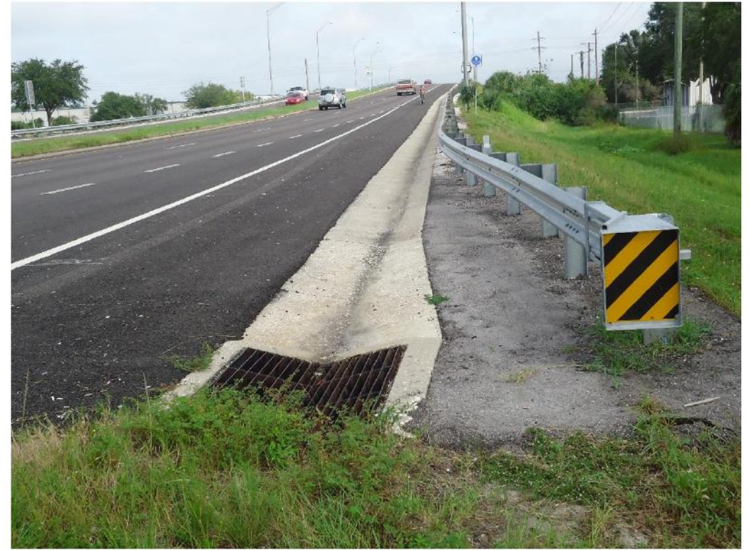
Shoulder Gutter Inlet on Overpass
