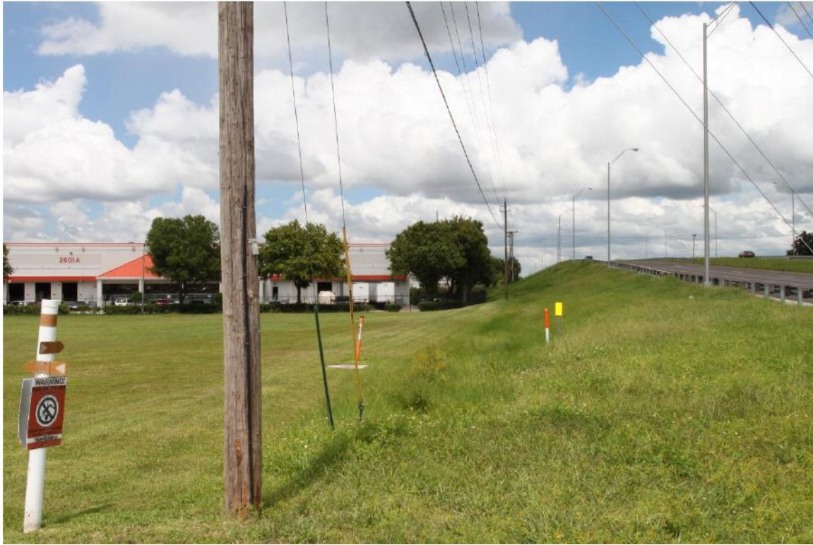
Overpass Embankment West Side of US 301 South of Broadway Avenue
