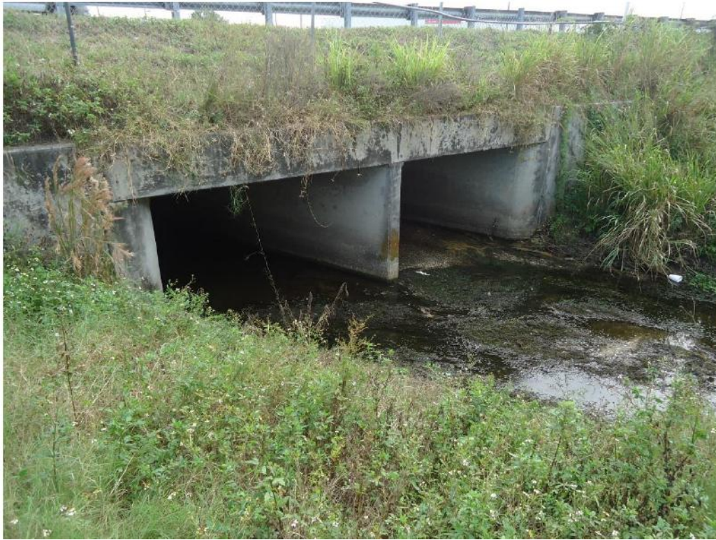
Double 10'x8' Bridge Culvert at Bruce Creek, Station 121+09
