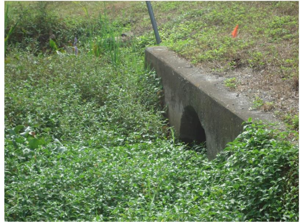
30" Cross Drain at Station 175+49
