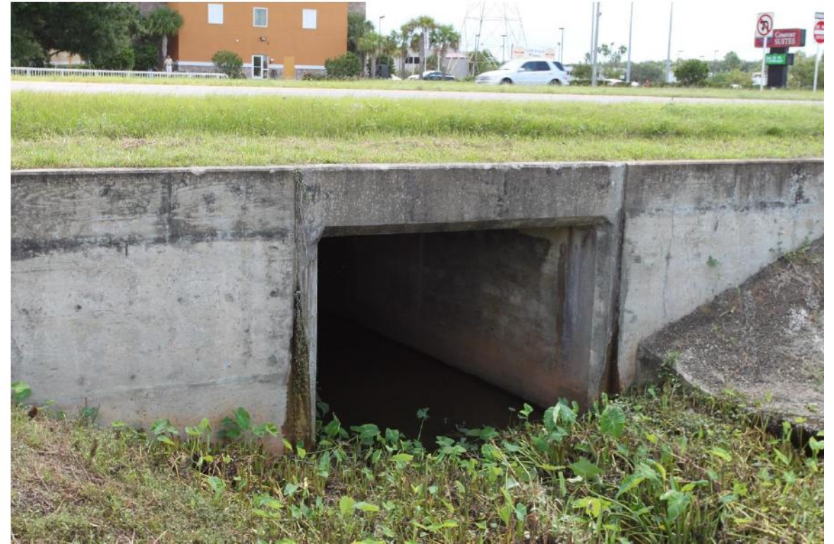
10'x8' Box Culvert at Station 248+42
