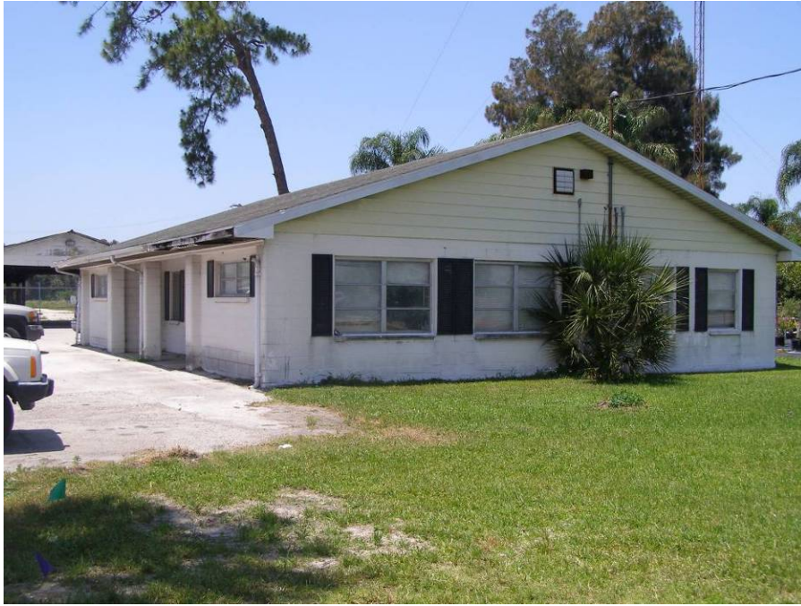
Photo 6-23 South and east elevations of 103 Big Bend Road, 8HI11370.
