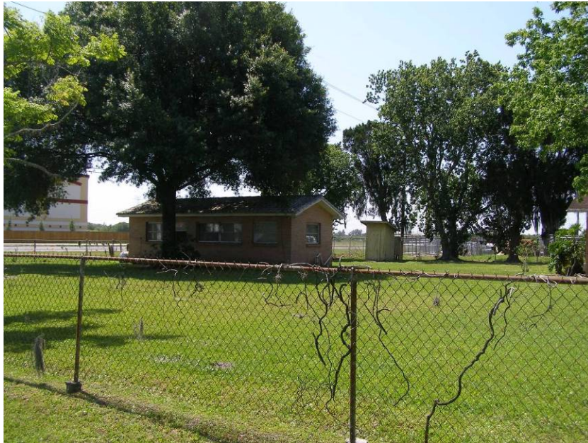
Photo 6-25 Ancillary structure to 6125 Adamsville Road, 8HI11371.
