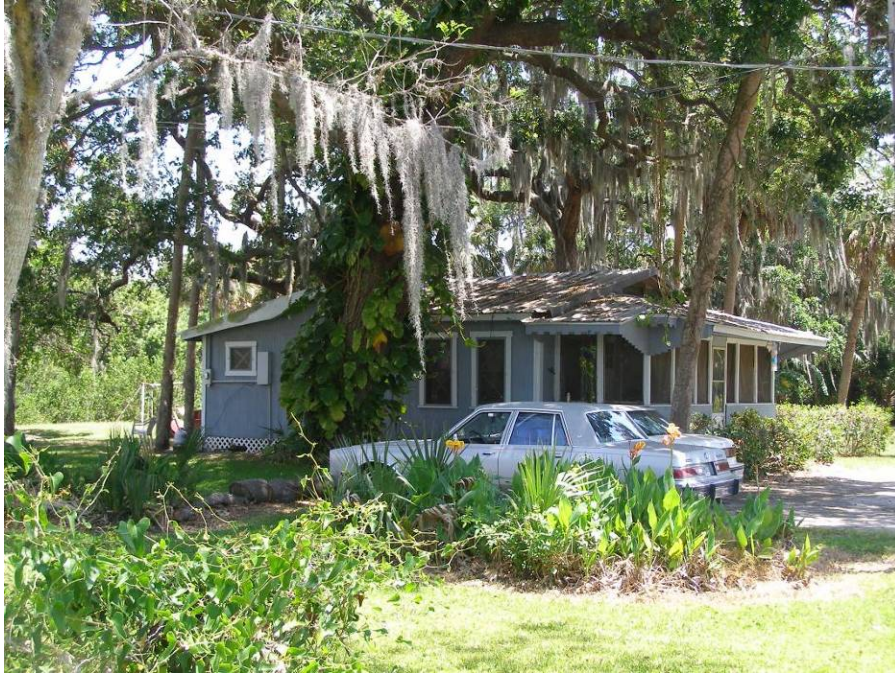
Photo 6-33 South and west elevations of 6214 Kracker Avenue, 8HI11379.
