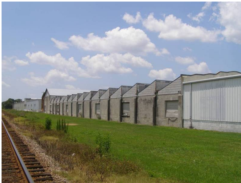
Photo 6-8 East elevation of the Ruskin Vegetable Corporation Warehouse, 8HI11362.
