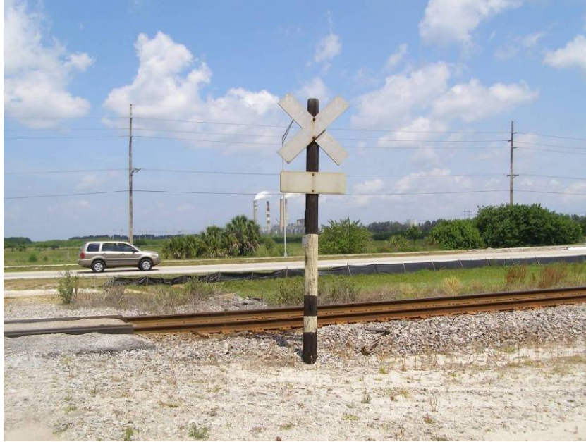
Photo 6-2 Detail of the northern railroad crossing within the recorded segment.
