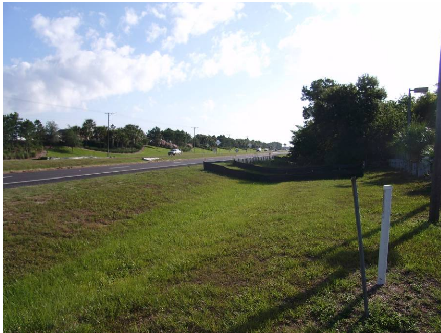
Photo 3-1 General view of the US 41 project corridor, looking north.
