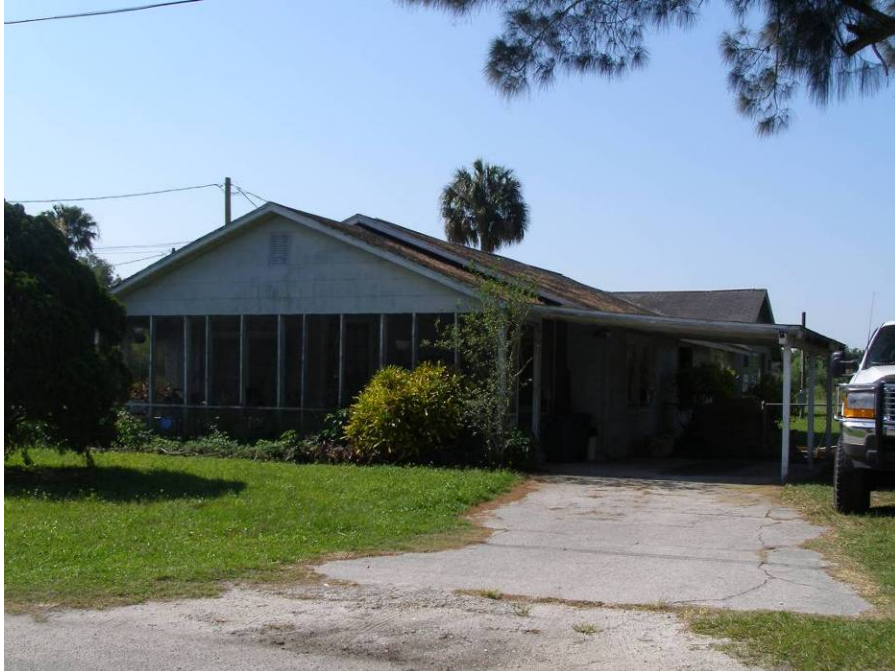
Photo 6-31 North and west elevation of 6115 Kracker Avenue, 8HI11377.
