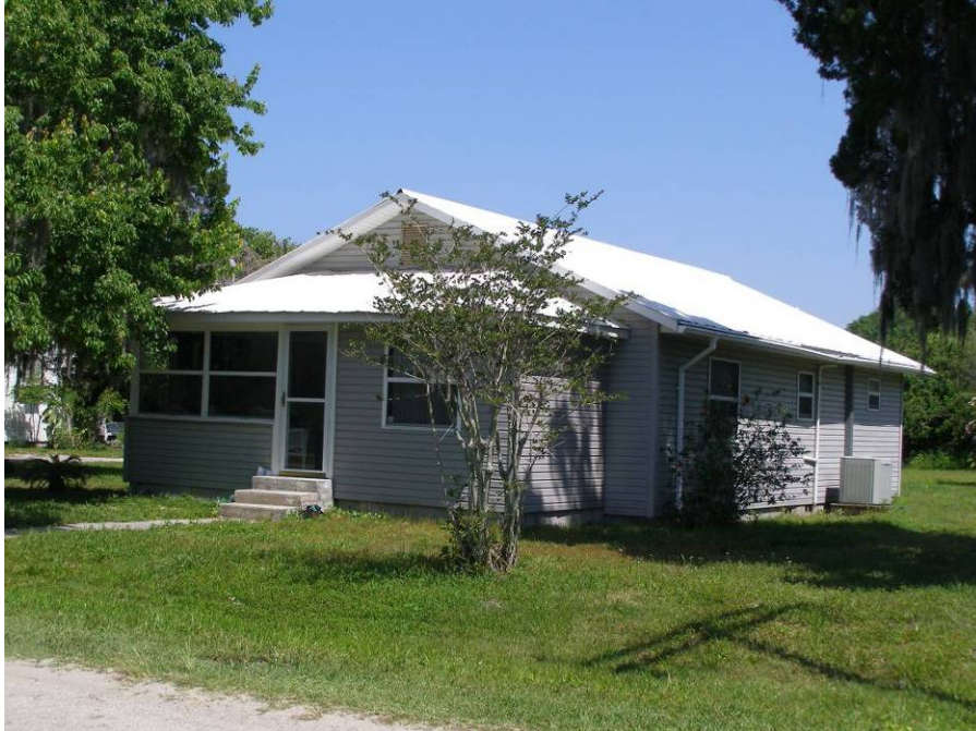
Photo 6-28 South and east elevations of 6126 Adamsville Road, 8HI11374.
