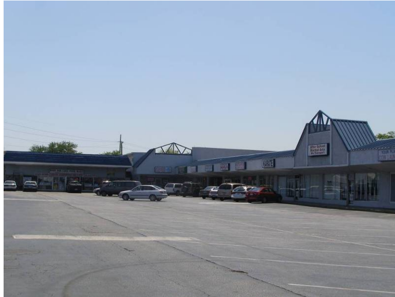
Photo 6-9 North and east elevations of 6018 South US Highway 41, 8HI11363.
