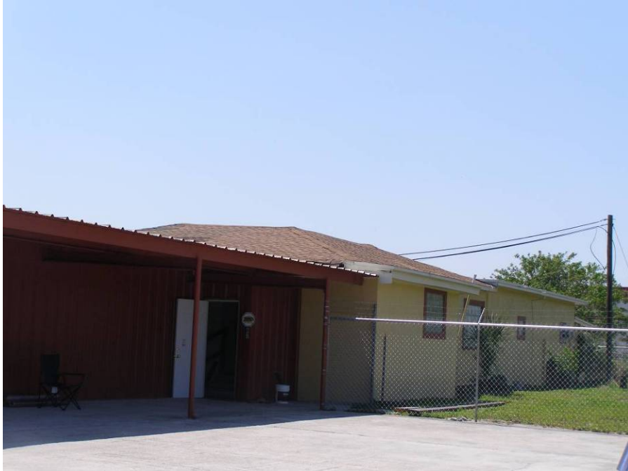
Photo 6-29 North and west elevations of 12623 South US Highway 41, 8HI11375.
