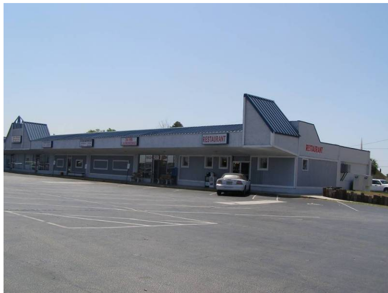
Photo 6-10 North and east elevations of 6018 South US Highway 41, 8HI11363.
