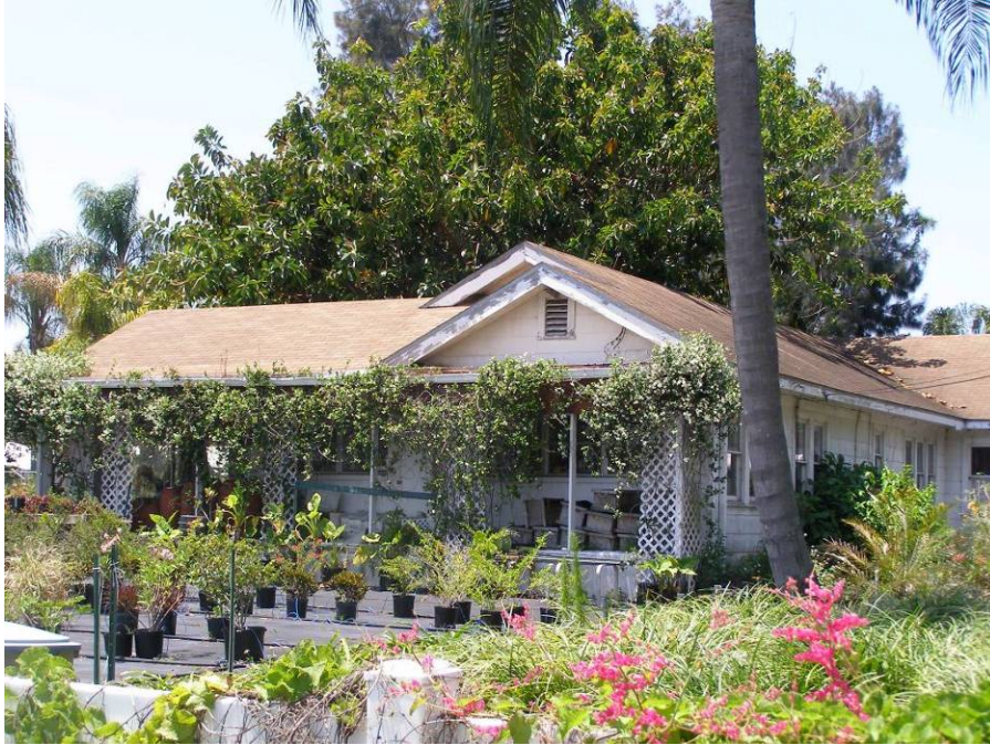
Photo 6-22 North and east elevations 101 Big Bend Road, 8HI11369.
