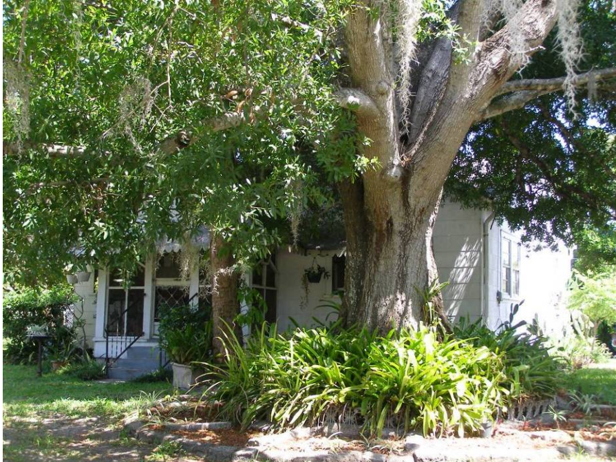
Photo 6-27 South and east elevations of 6124 Adamsville Road, 8HI11373.
