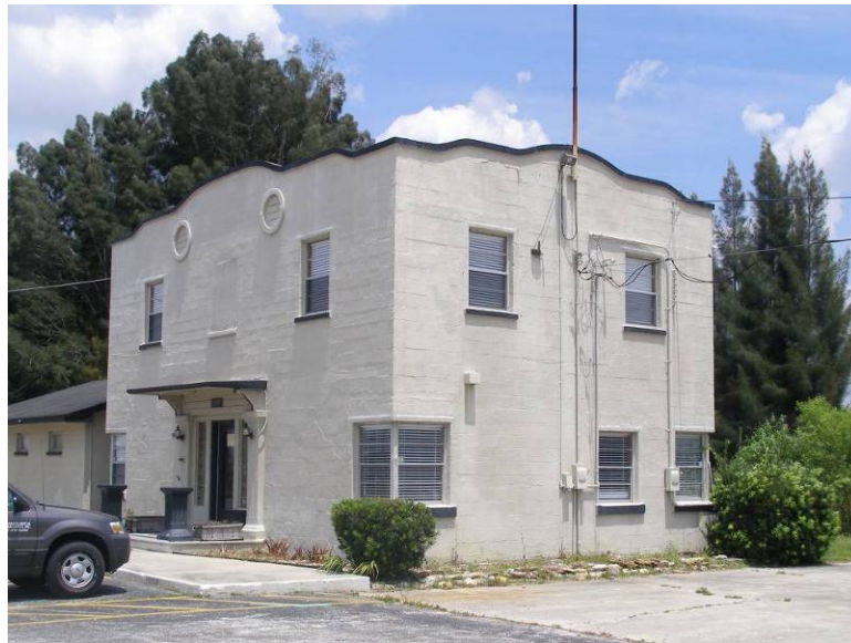
Photo 6-6 South and west elevations of the Ruskin Vegetable Corporation Office, 8HI1010.
