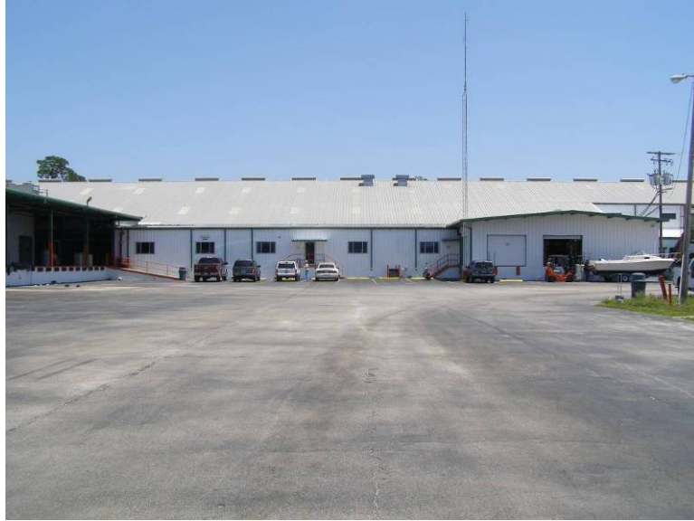
Photo 6-16 West elevation of the Pacific Tomato Growers Ltd. Packinghouse at 6855 North US Highway 41, 8HI11365.
