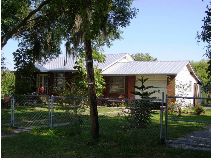
Photo 6-32 South and east elevations of 6118 Kracker Avenue, 8HI11378.
