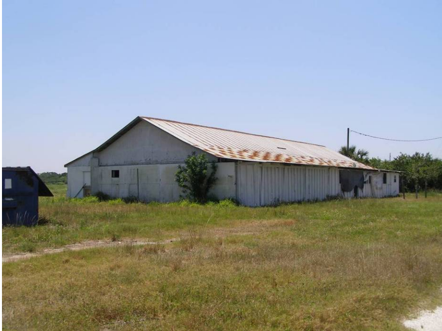
Photo 6-21 North and west elevations of 13124 South US Highway 41 (8HI11360), looking southeast.
