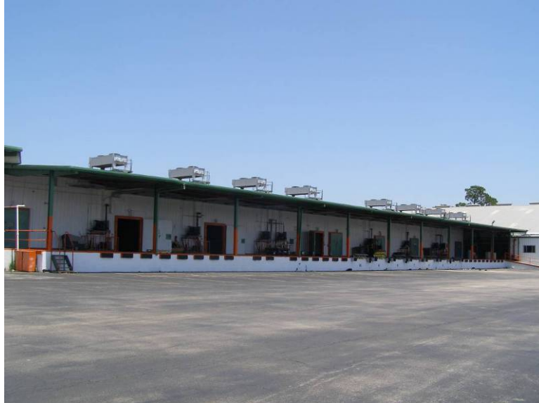
Photo 6-17 Circa 1970 addition to the Pacific Tomato Growers Ltd. Packinghouse at 6855 North US Highway 41, 8HI11365.
