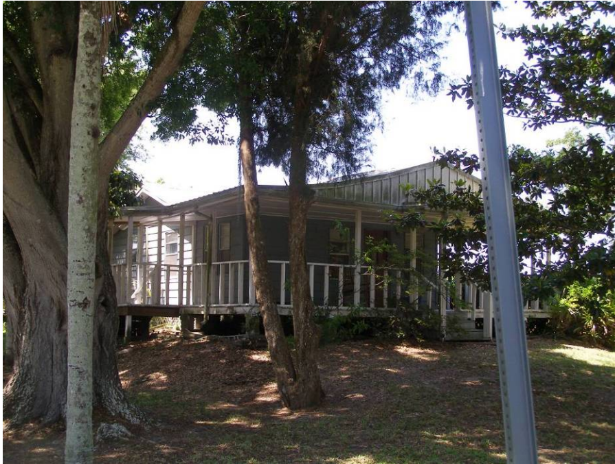
Photo 6-26 North and east elevations of 6123 Adamsville Road, 8HI11372.
