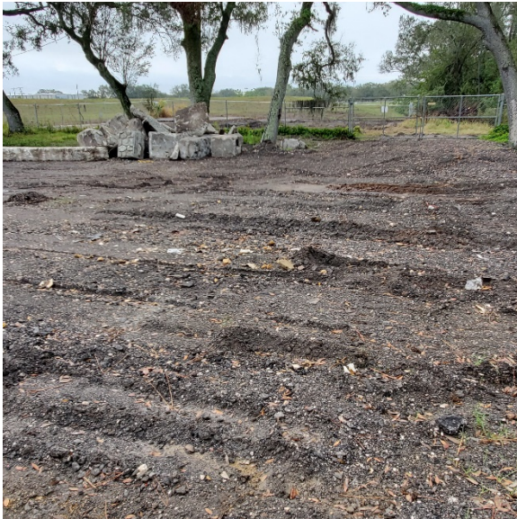
POND 2B – West boundary looking south
