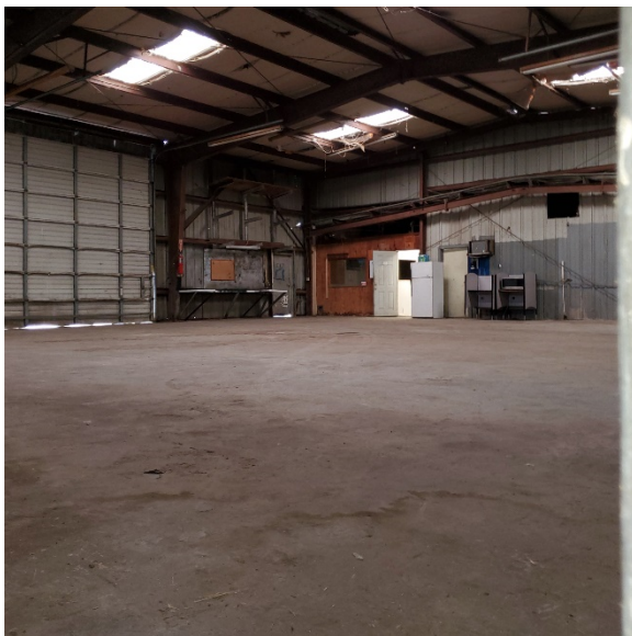
POND 1A – inside building looking northeast
