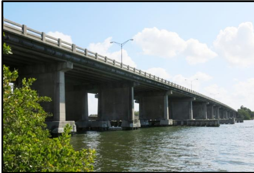
Photo 5-21: The Doyle E. Carlton Bridge/Alafia River Bridge (8HI11793), facing southeast.
