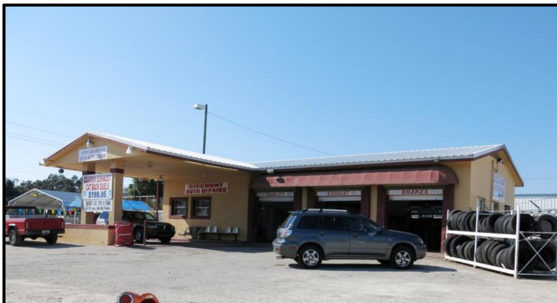
Photo 5-10: The east and north elevations of the Masonry Vernacular style auto repair shop at 10181 S US 41 (8HI12085).
