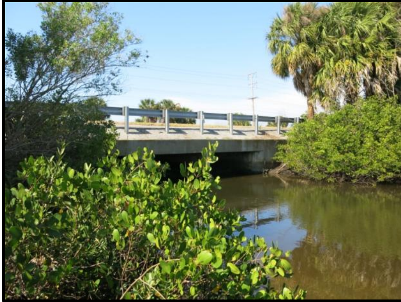
Photo 5-26: The Archie Creek Bridge (8HI12021), facing northwest.
