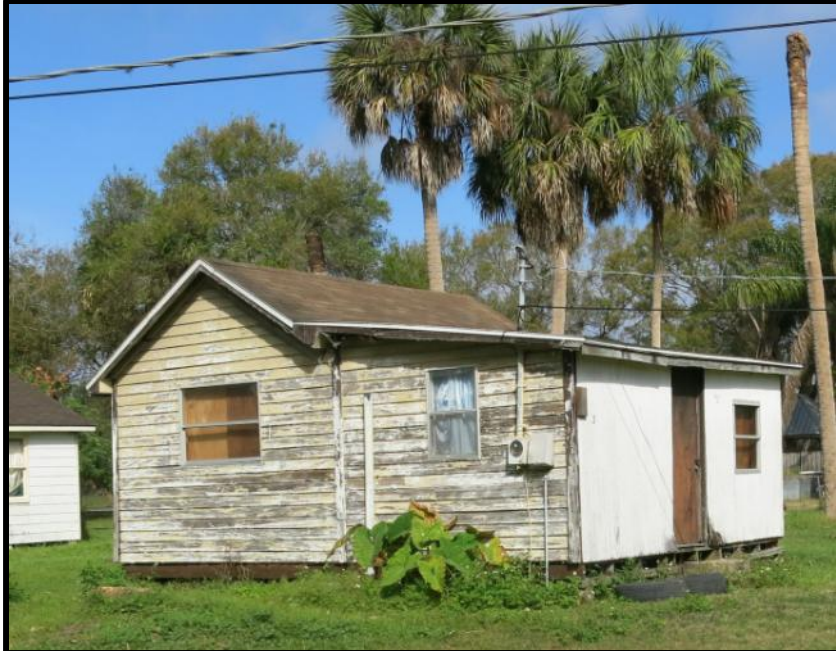
Photo 5-13: The west and south elevations of the Frame Vernacular style residence at 12150C S US 41 (8HI12032).
