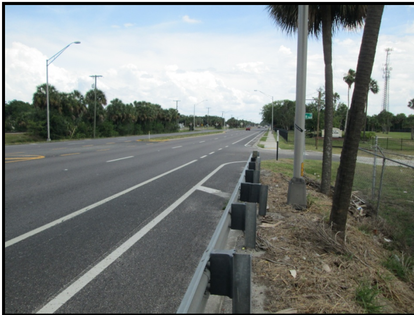
Photo 2-1: General view of US 41, looking south-southeast.
