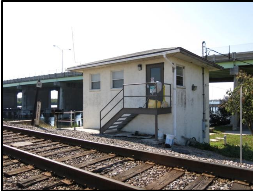
Photo 5-24: The Alafia River Swing Span Bridge's Tender Station (8HI1007), facing southwest.
