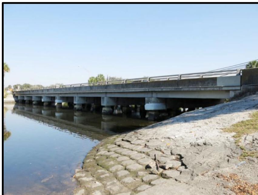
Photo 5-20: The Bullfrog Creek Bridge (8HI12019), facing northeast.
