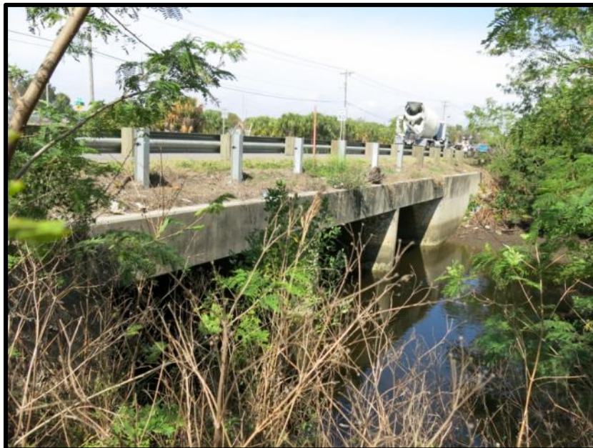
Photo 5-28: The Delaney Creek Bridge (8HI12023), facing northwest.
