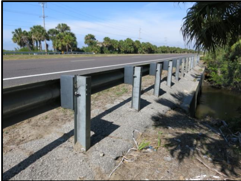
Photo 5-25: The Archie Creek Bridge (8HI12020), facing northwest.
