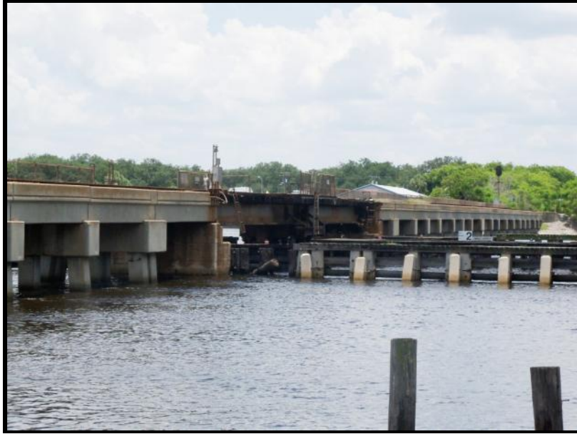
Photo 5-22: The Alafia River Swing Span Bridge (8HI1007), facing northwest.
