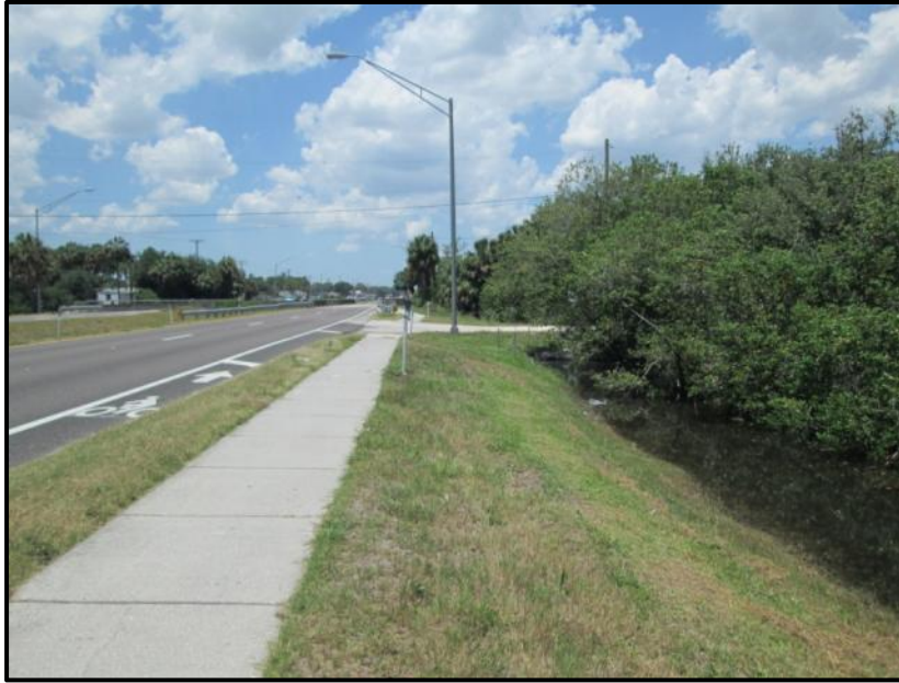
Photo 2-2: US 41, facing north toward Bullfrog Creek.
