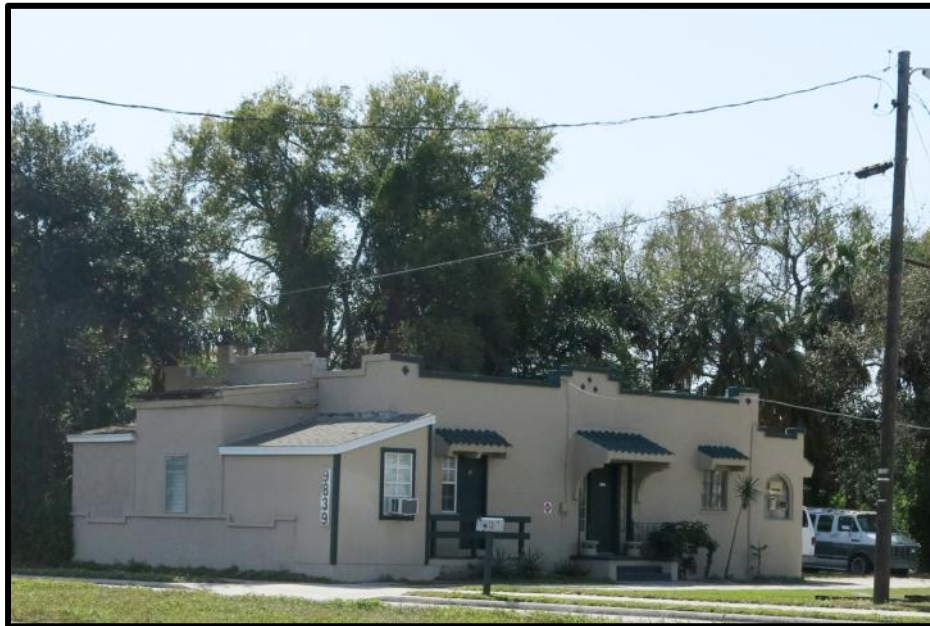
Photo 5-18: The east and north elevations of the Mediterranean Revival style motel building at 9839 S US 41 (8HI1058A).
