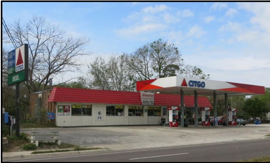
Photo 5-11: The south and east elevations of the Masonry Vernacular style commercial building at 10143 S US 41 (8HI12086).
