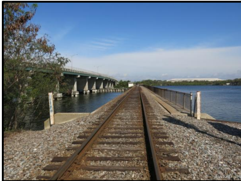
Photo 5-23: The Alafia River Swing Span Bridge (8HI1007), facing north. The CSX Railroad (8HI10237) is in the foreground. The Doyle E. Carlton Bridge/Alafia River Bridge (8HI11793) is to the left.
