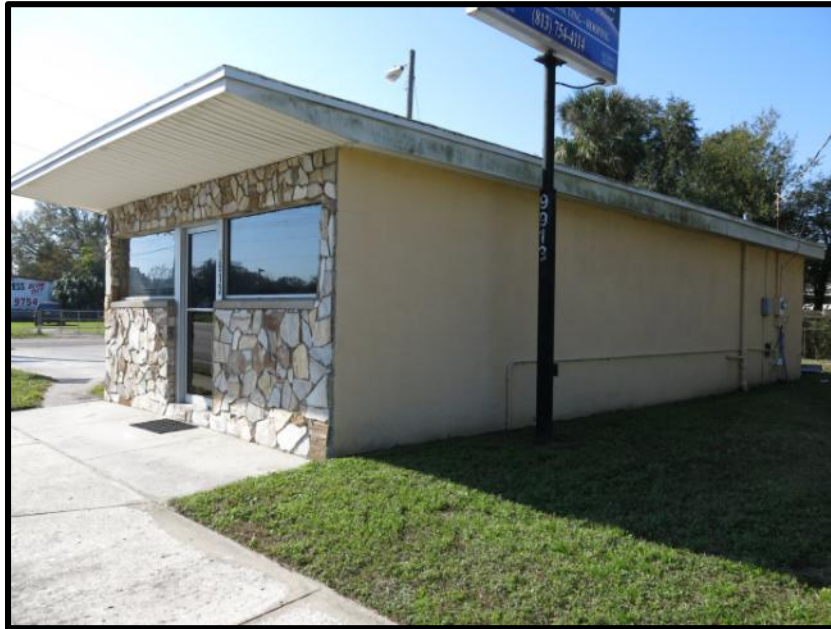
Photo 5-9: The east and north elevations of the Masonry Vernacular style commercial building at 9913 S US 41 (8HI12092).
