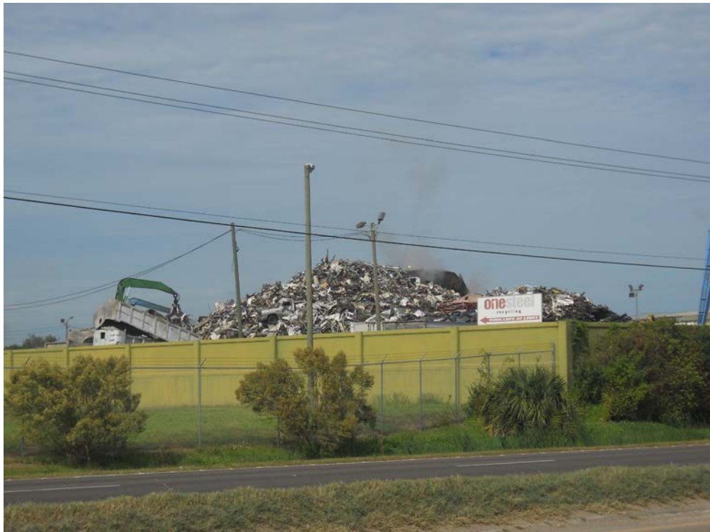
PHOTO 36: Site No. 41 - Nematode Controllers Located at 5001 US 41. View to the northwest.
