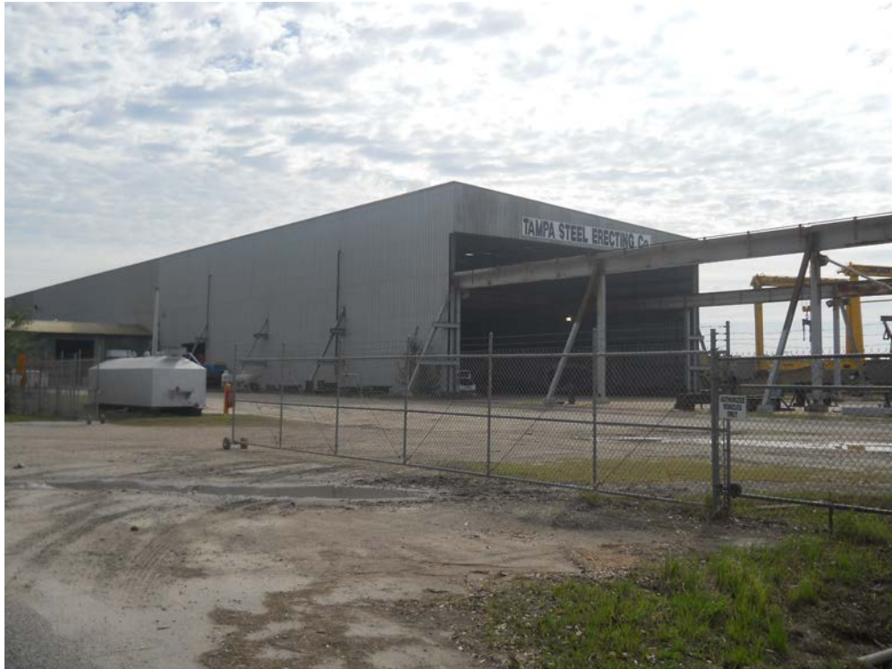
PHOTO 29: Site No.31 - Tampa Steel Erecting Co. Located at 5127 Bloomingdale Avenue.
