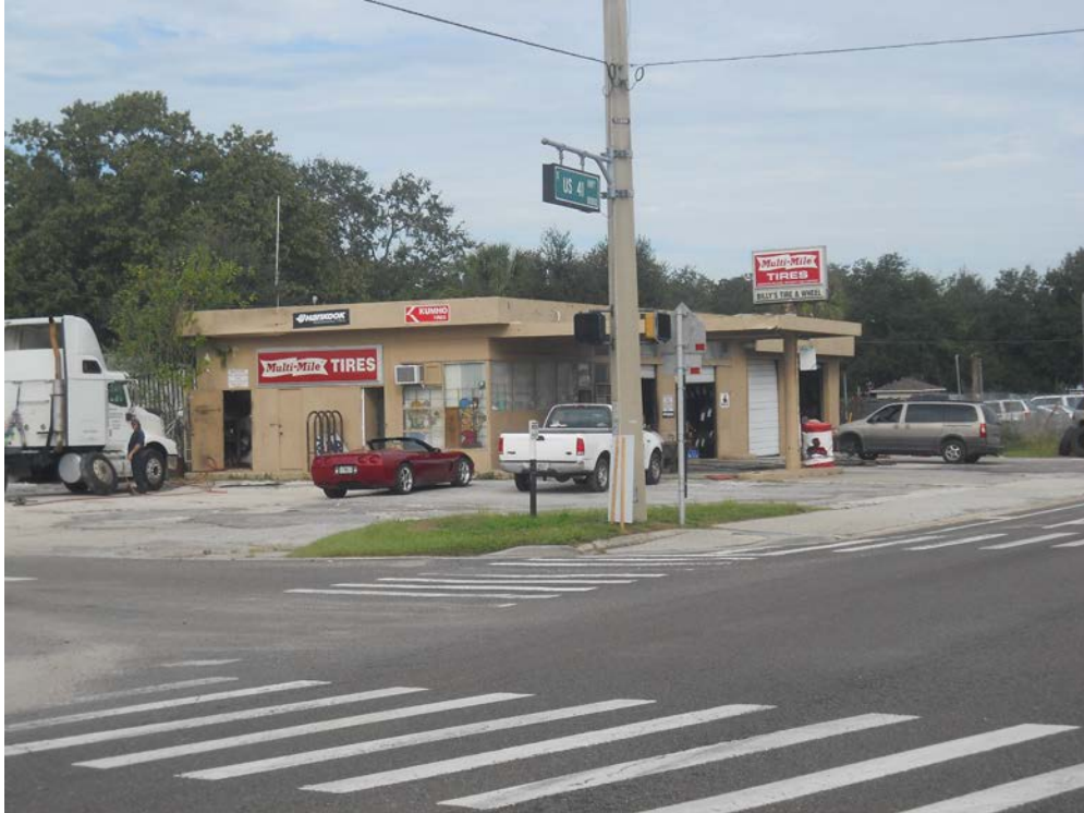
PHOTO 23: Site No. 23 - Billy's Tire & Wheel Located at 10045 US 41. View to the northwest.
