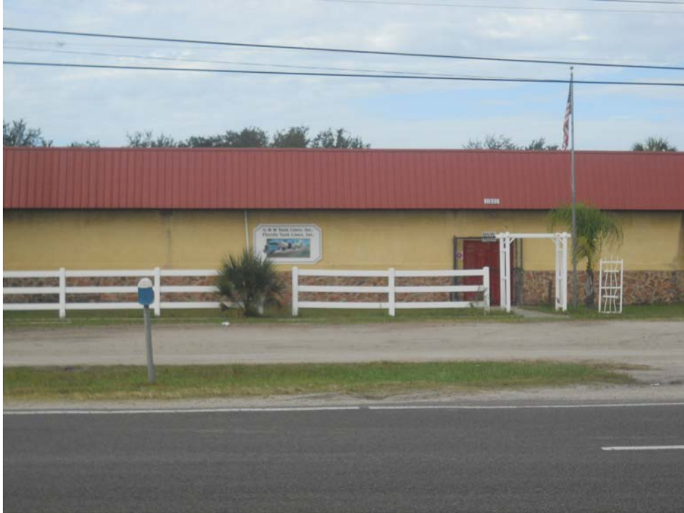
PHOTO 13: Site No. 13 - G & W Tank Lines Located at 11201 US 41
