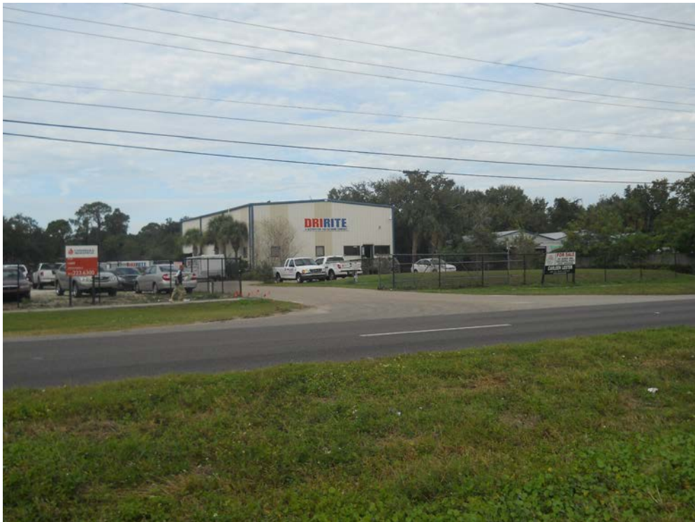
PHOTO 8: Site No. 6 - Dririte Restoration and Cleaning Located at 11841 US 41.
