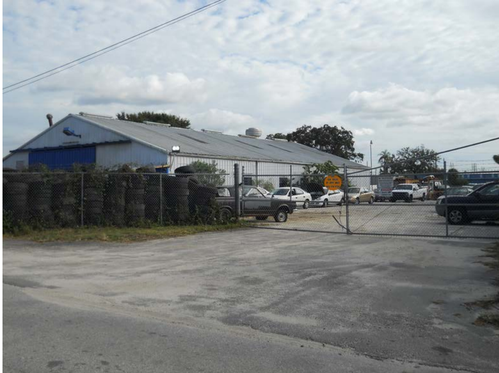
PHOTO 41: Site No. 47 - Former HiTech Products Located at 4917 Hartford Street. View to the southeast.
