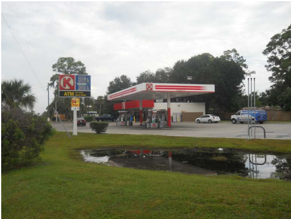
PHOTO 4: Site No. 2 - Circle K #7032 Located at 12140 US 41. View to the north.
