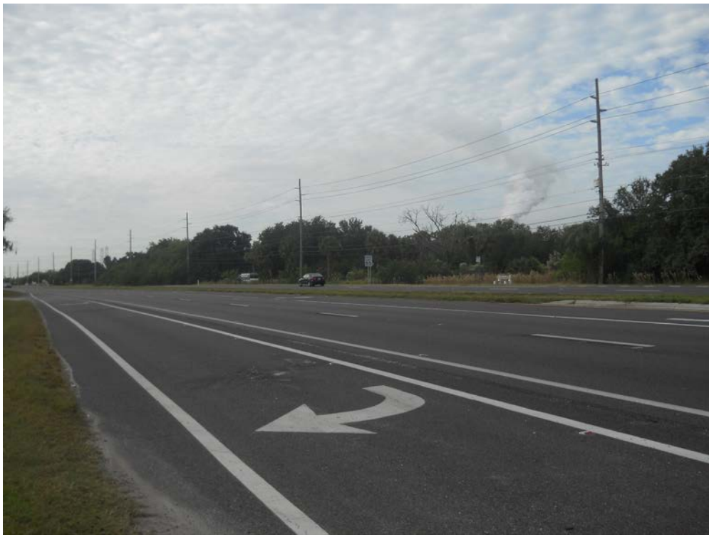
PHOTO 2: View to the south along US 41 from Kracker Avenue
