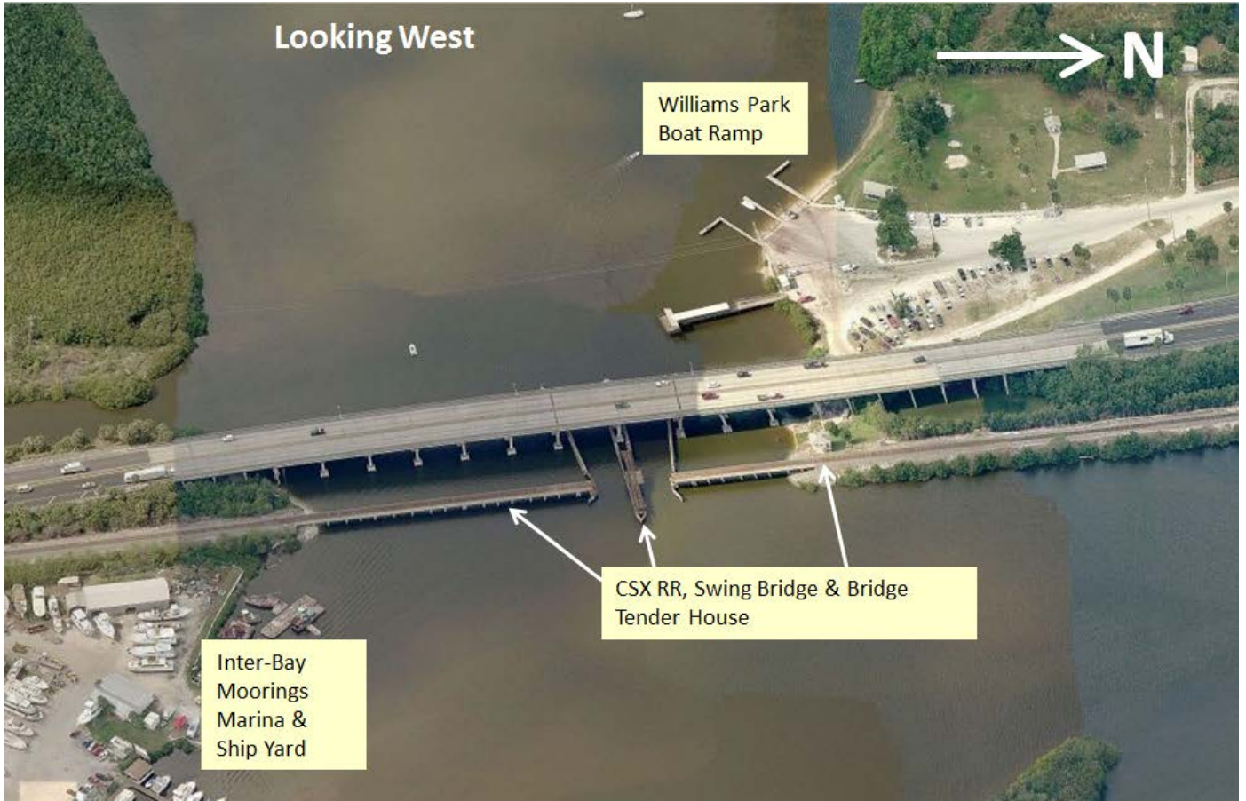
Looking north along US 41 at the top of the bridges – note the narrow sidewalks and lack of shoulders and bike lanes
