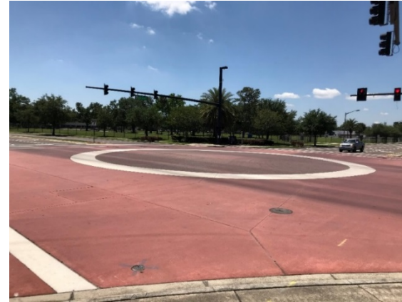
Exhibit 47. Concrete Intersection at Livingston St. and Maguire Blvd.
