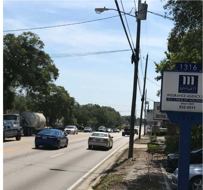
Exhibit 23. Existing West Busch Boulevard Sidewalk Gap (Between N. Orleans Ave. and N. Willow Ave.)
