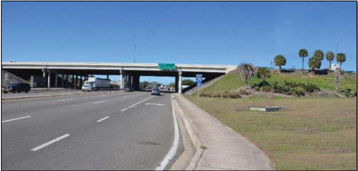
Existing View looking West
