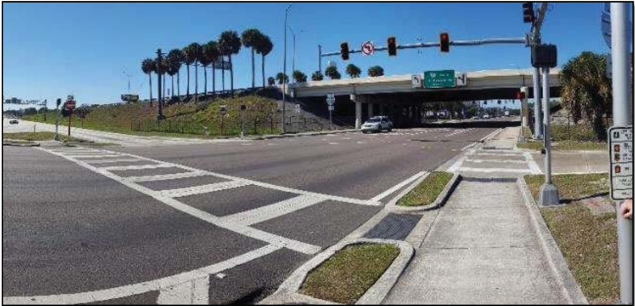
Existing View looking West
