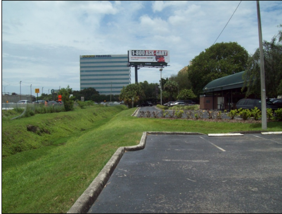
Photo 1: Drainage ditch between Site C and I-275. Looking west.
