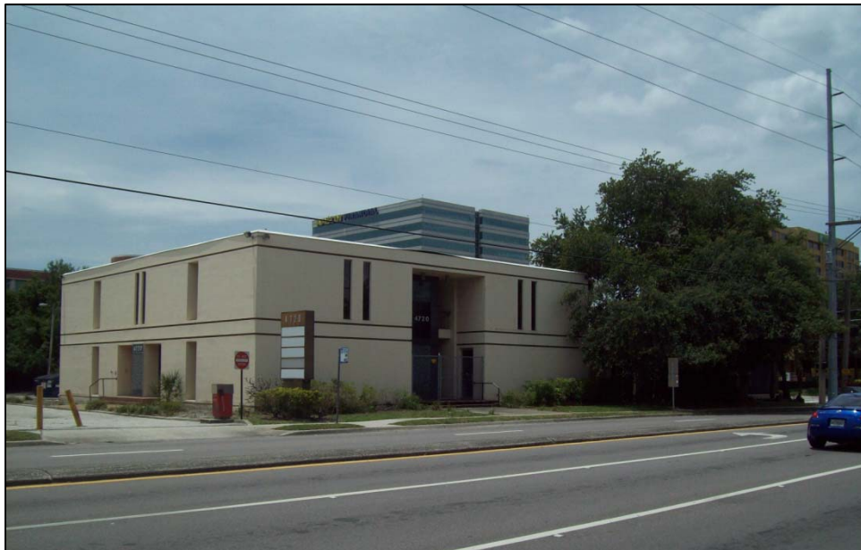
Photo 5: 4720 W. Cypress Street, east side. Looking southwest.
