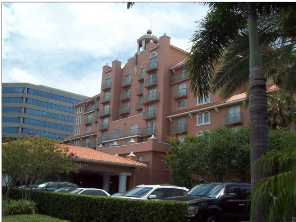
Photo 2: Sheraton Suites Hotel on Site C. Looking southeast.
