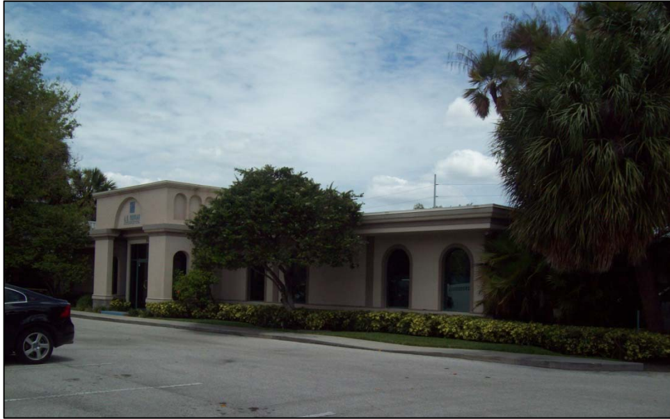
Photo 7: 716 N. Renellie Drive, south façade. Looking northwest.
