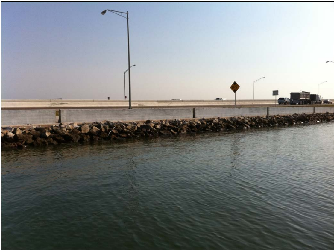
Photo 2. View of bridge embankment and seawall with riprap.
