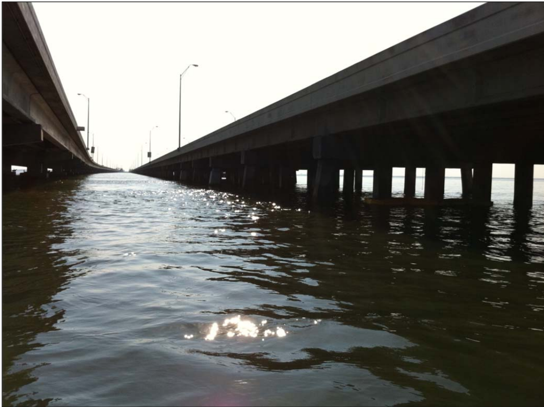
Photo 5. View of habitat between bridge spans.
