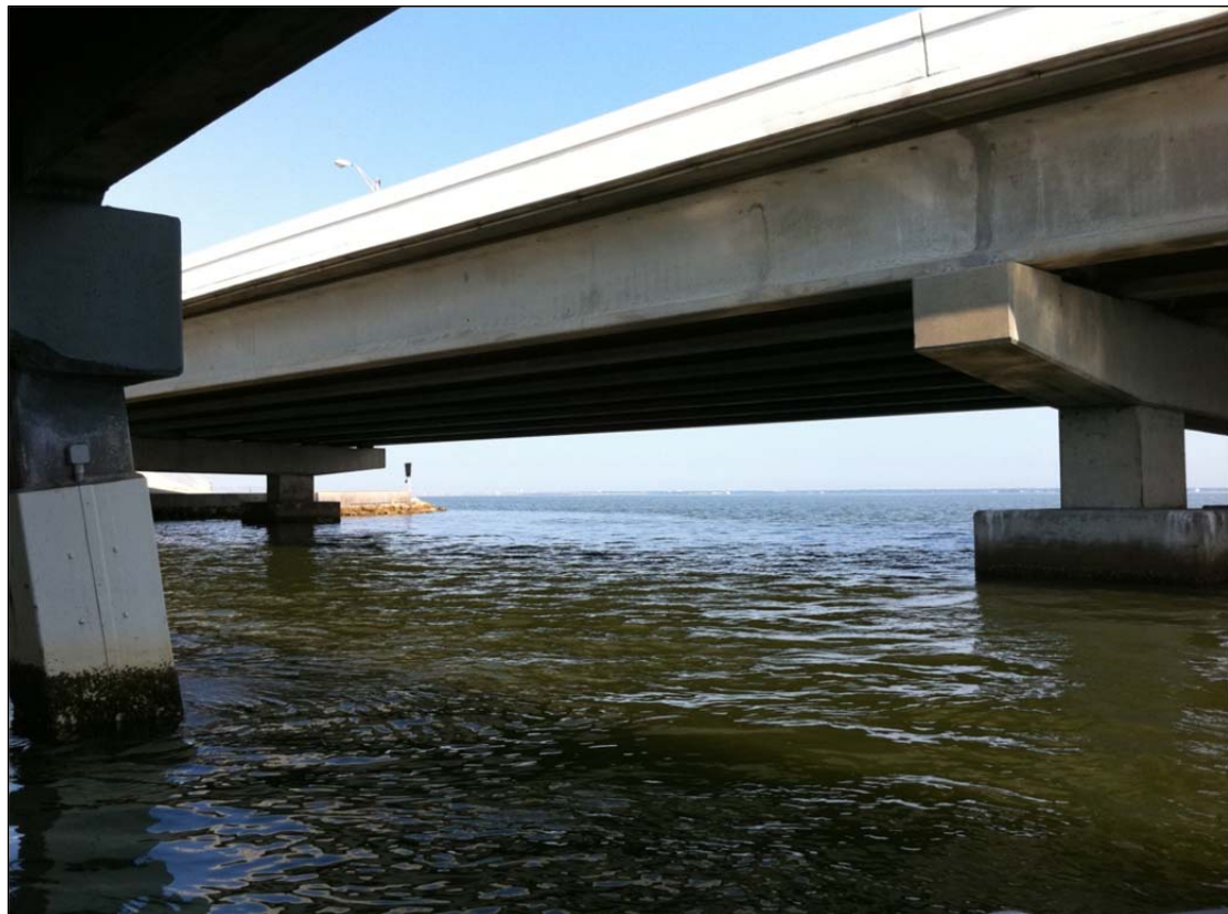
Photo 4. View of bridge piers.
