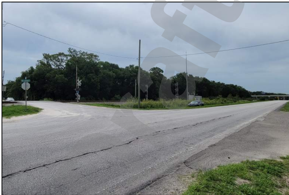
Photo 5-22 Old Lakeland Highway (8PA03343), looking southeast from the northwest corner of Old Lakeland Highway and Messick Road looking southeast
