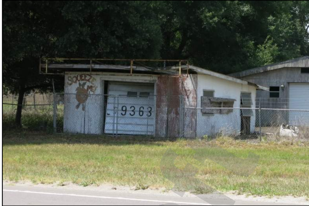
Photo 5-20 Building with no style (8PA03354) located at 9363 US Highway 98, looking south.
