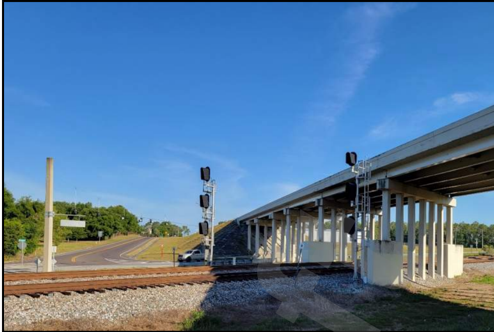
Photo 5-13 South Florida Railroad – Pemberton Ferry Branch/Richloam Railroad (8PA02802), looking northwest.
