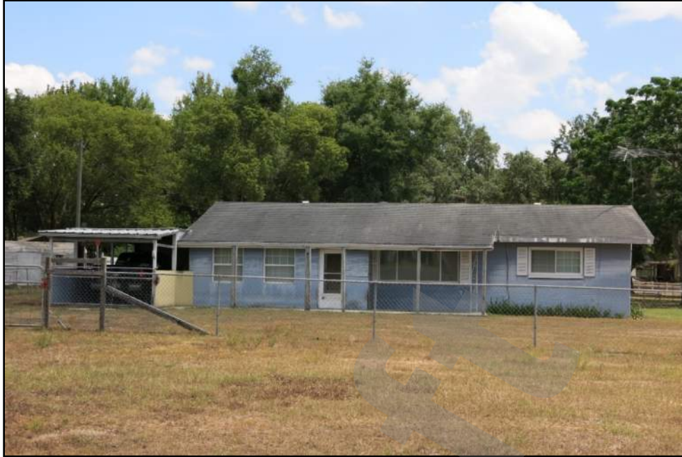
Photo 5-17 Masonry Vernacular style building (8PA03362) located at 10150 US Highway 98, looking northeast.
