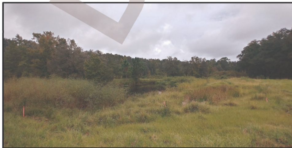
Photo 5. Looking north at a borrow pit impacting SMF 200-1.
