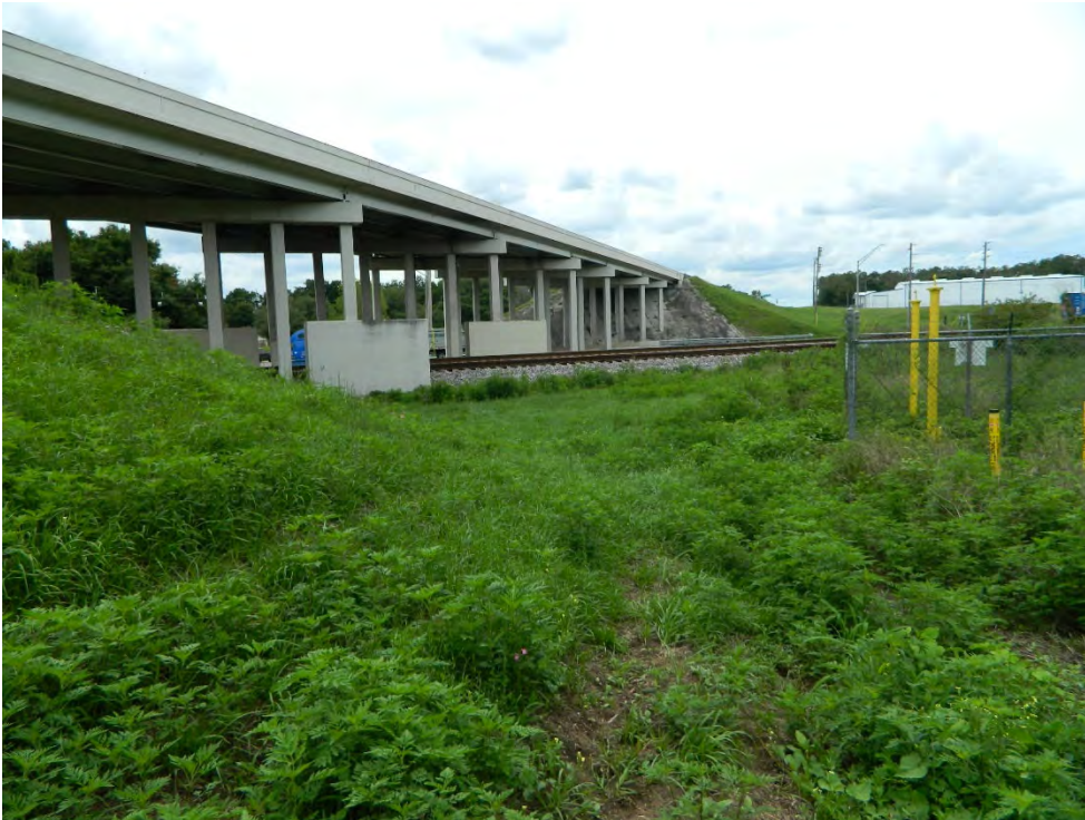
Photo 12: US 98 Bridge Over CR 35A
