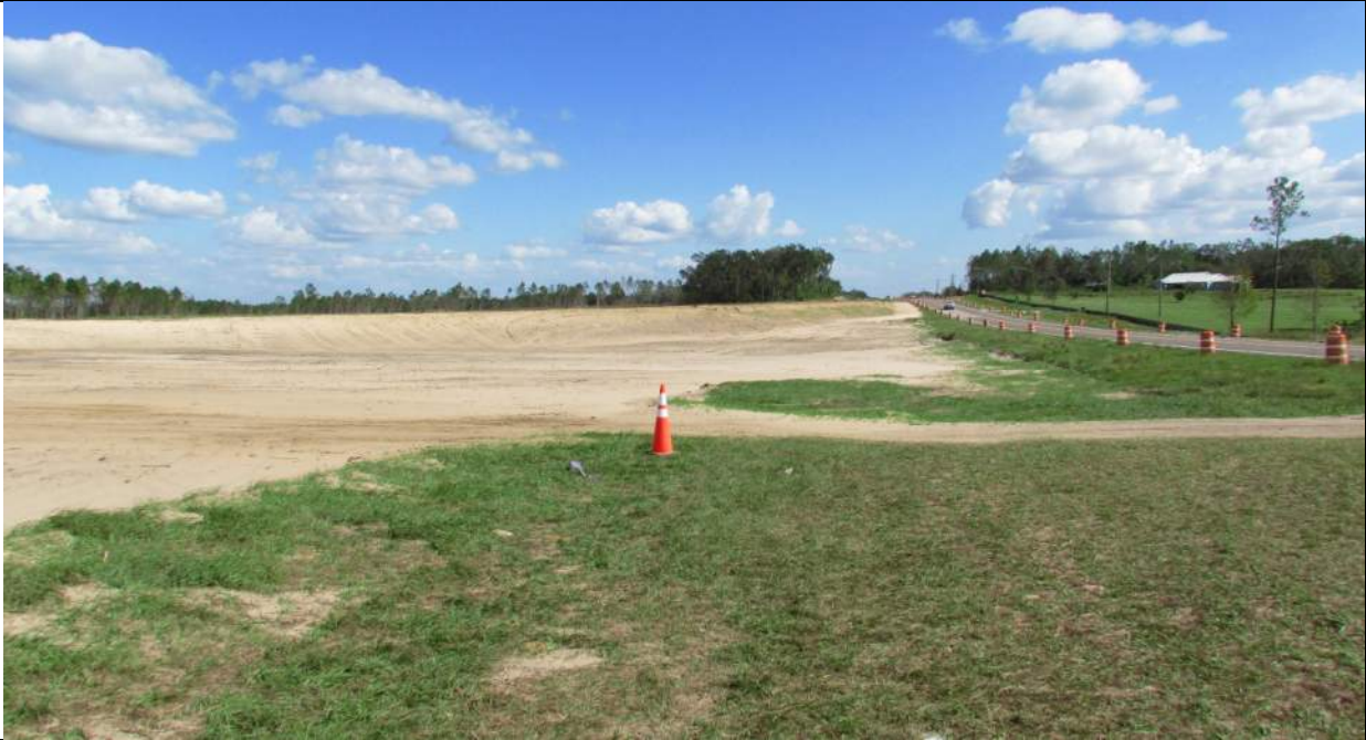
Old US 98 Roundabout
