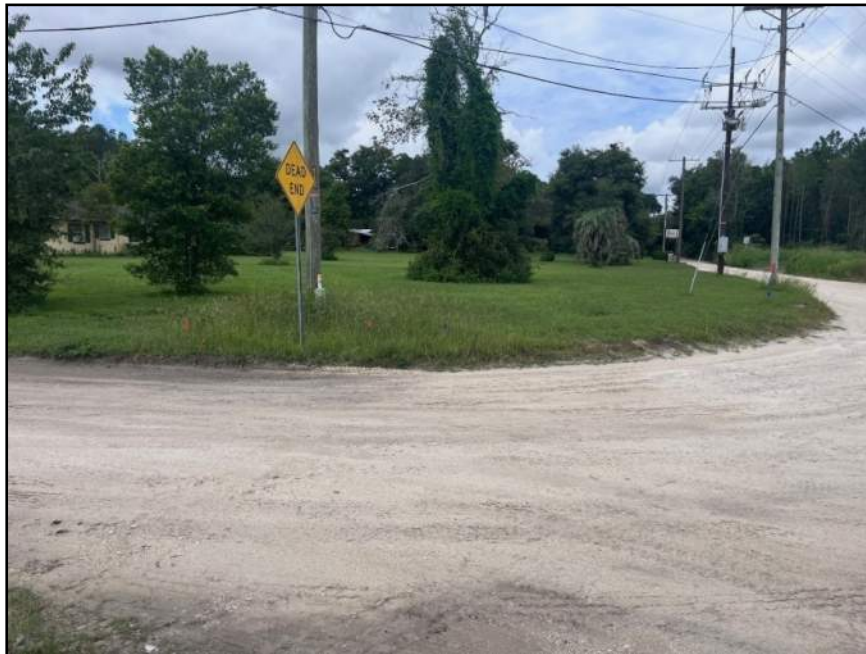
Photo 4: Current Condition of Townsend Road west of US 98
