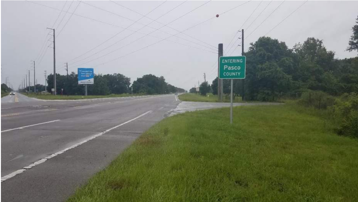
South project limit, looking north along US 98 at CR 54/US 98 intersection
