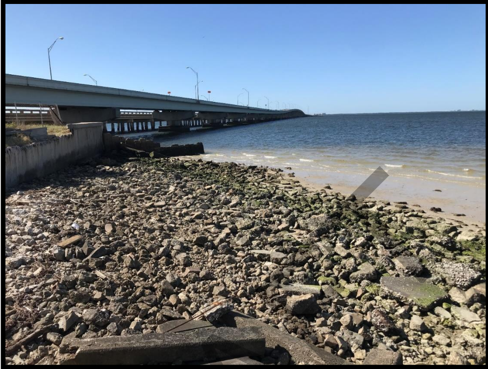
Photo 5: Gandy Bridge over SW 4, facing southwest
